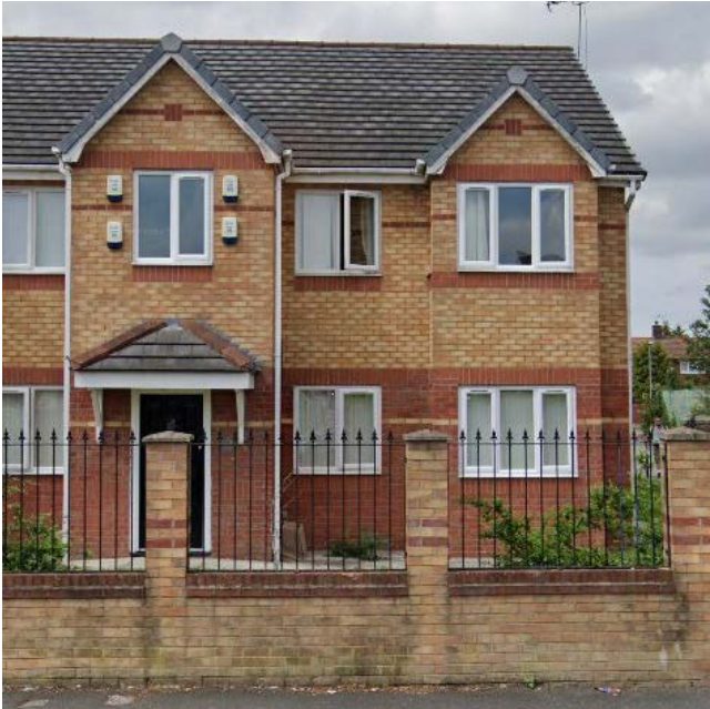
Fig.7 Tall two storey blocks along Brook Hey Drive / Credit Google
