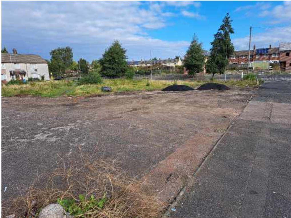
Photograph 3 View north along eastern site boundary showing presence of asphalt stockpile.
