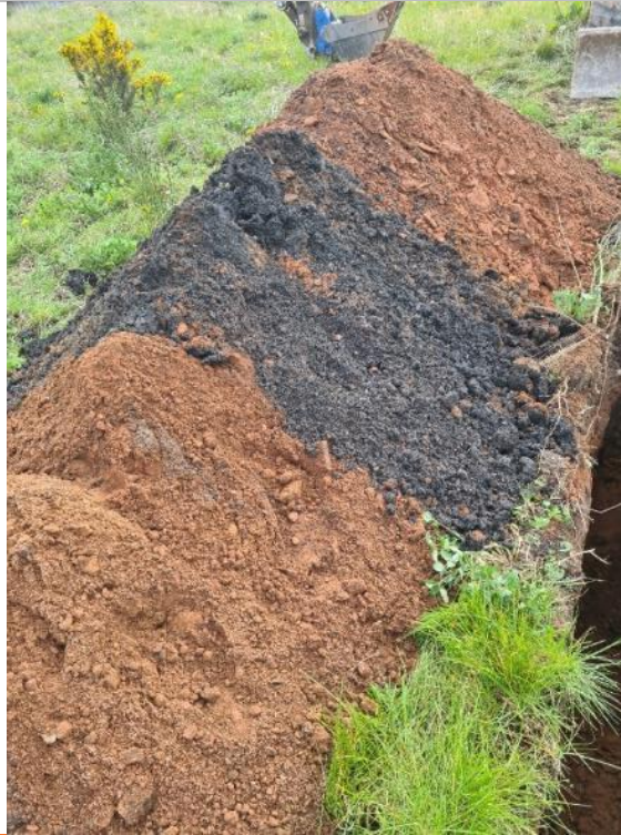
PLATE 12 BACKFILLED TRIAL PIT
