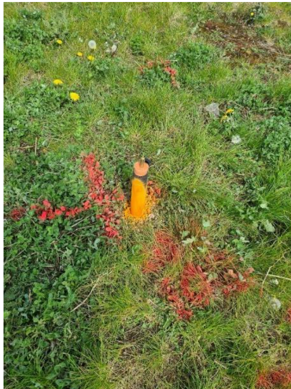
PLATE 8 WS102 MONITORING WELL
