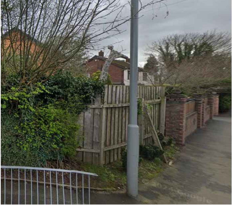
Corner of Tarbock and Wheathill Road boundary is a 1.8m high close boarded timber fence with small trees and hedgerow to be removed and replaced with blockwork wall with render finish.
