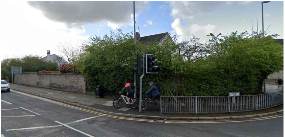
Boundary block wall on Tarbock Road measuring at 2375mm at its highest point and 2150mm at its lowest point. Block wall with coping stone.
