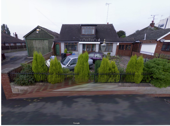
01 - Converted Bungalow, Mill Lane
