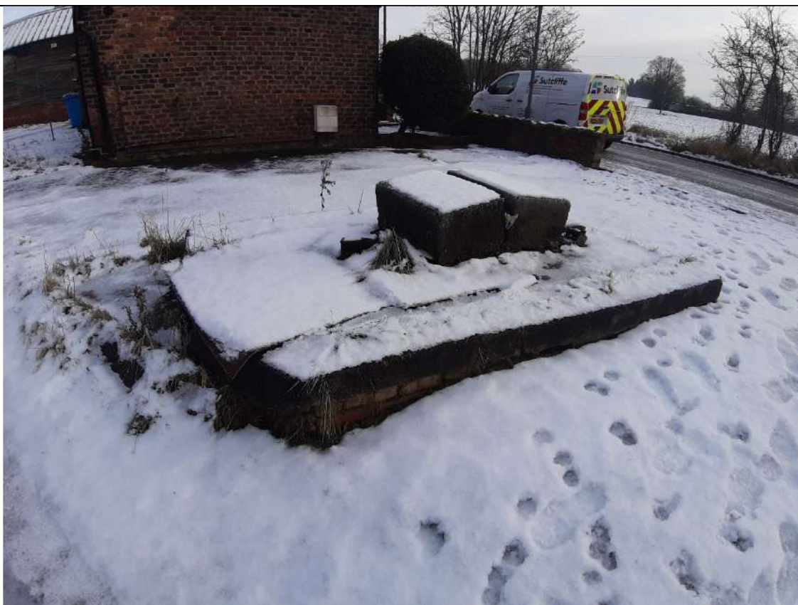
Plate 7 – Detail of former fuel pump
