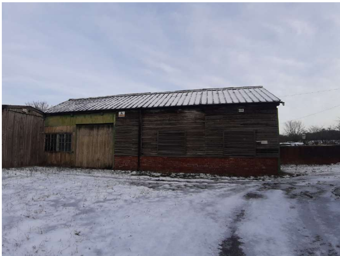
Plate 3 – showing rear yard area and wooden barn
