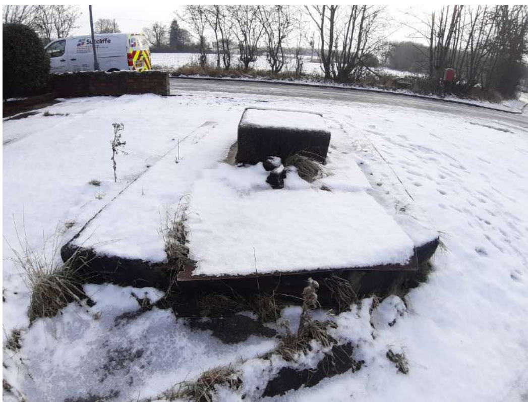
Plate 8 – Detail of former fuel pump
