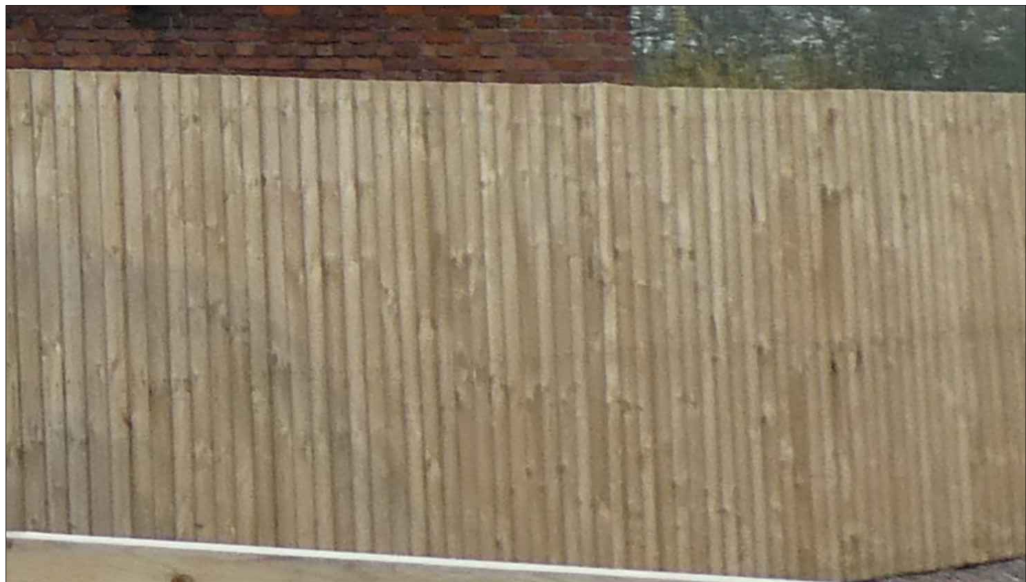
PHOTOGRAPHS OF EXISTING 2.0m HIGH TIMBER FENCE TO FORM NEW 2.0m HIGH WEST BOUNDARY (NTS)
