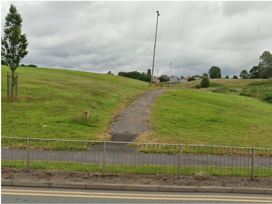
Figure 7: Footway crossing the development site, viewed looking east from the A506
