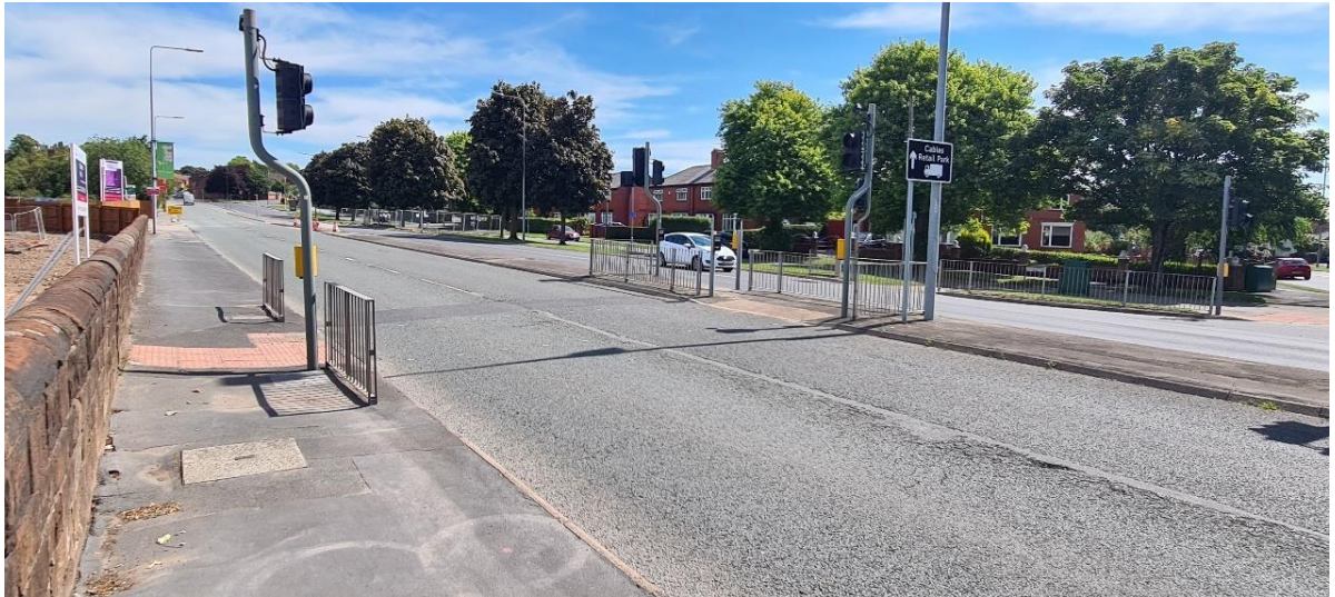
Figure 2.3 – Existing Liverpool Road Pedestrian Infrastructure
