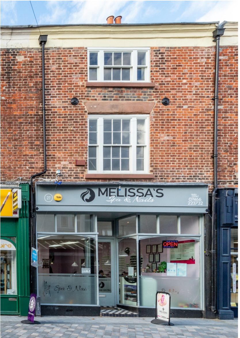
27 Eccleston Street - Shop front to be matched at 25 Eccleston Street
