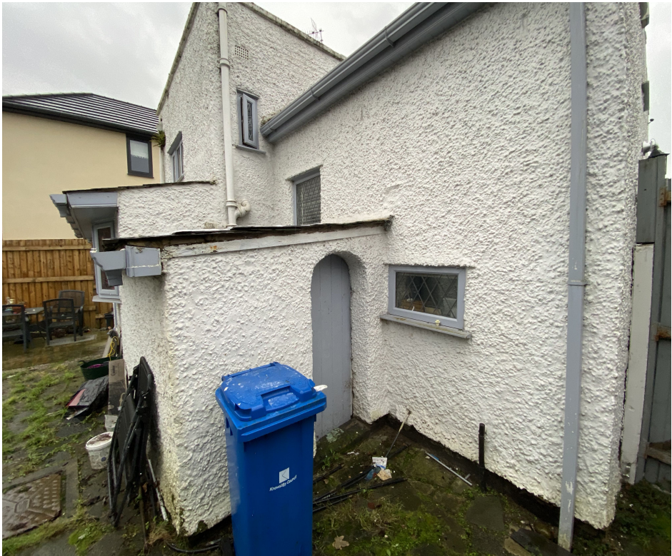
SIDE OF PROPERTY (WEST)
