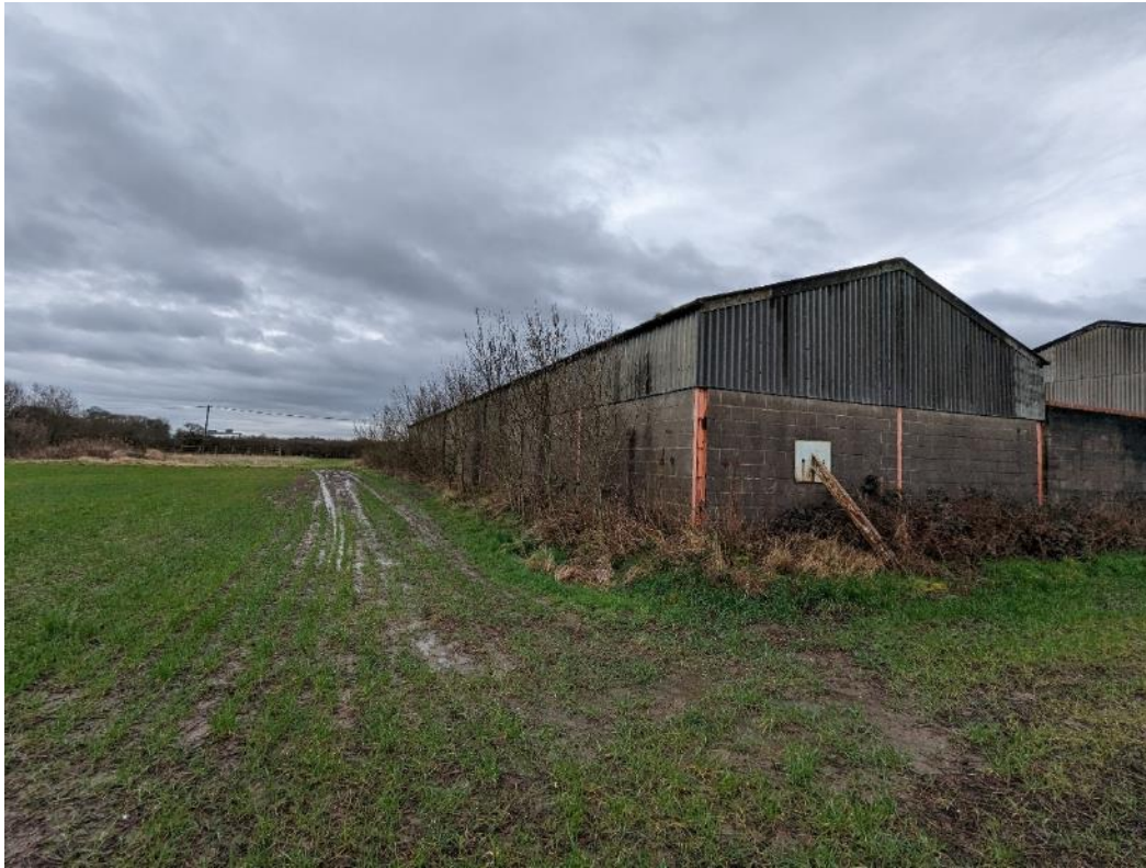
Plate 7 – South-east boundary where the arable abuts the adjacent farm building
