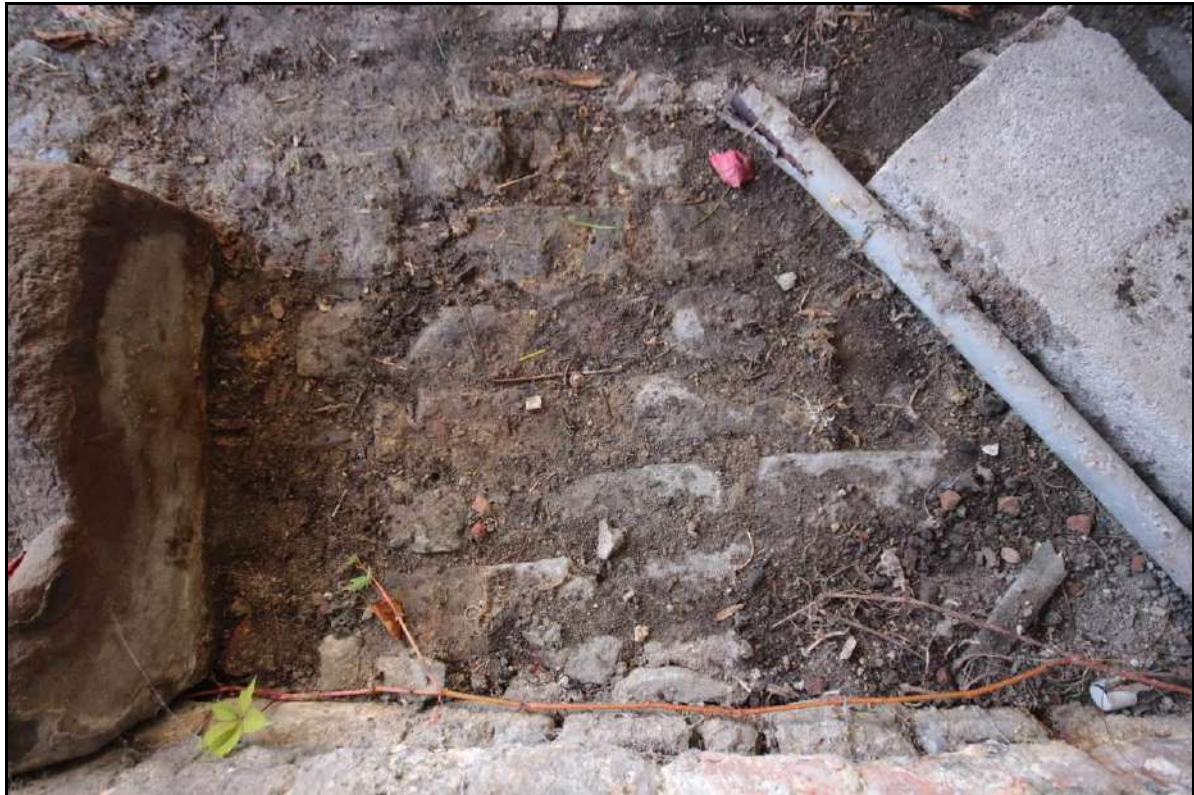
Photograph 76: View of the brick flooring of Room 4, taken facing north (File: HBR_133)
