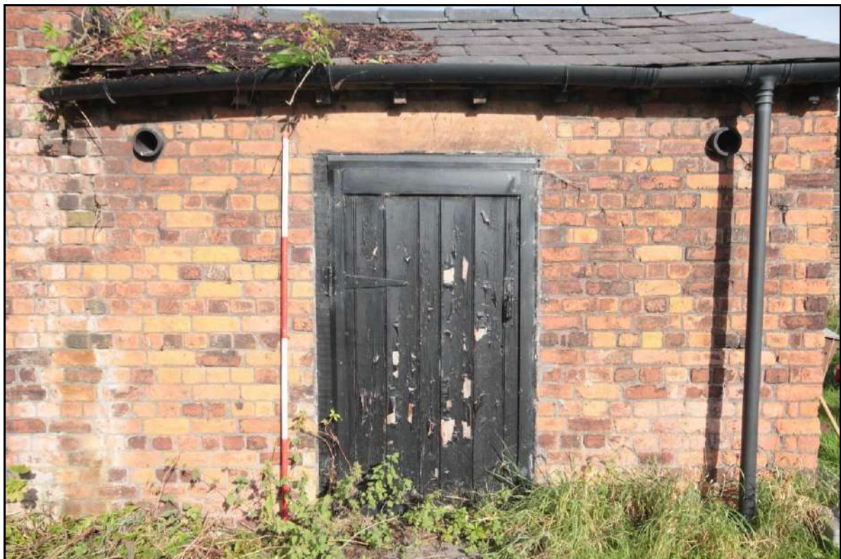
Photograph 32: View of the door flanked by vents on the southern elevation of the outbuilding, taken facing north with 2m scale (File: HBR_40)
