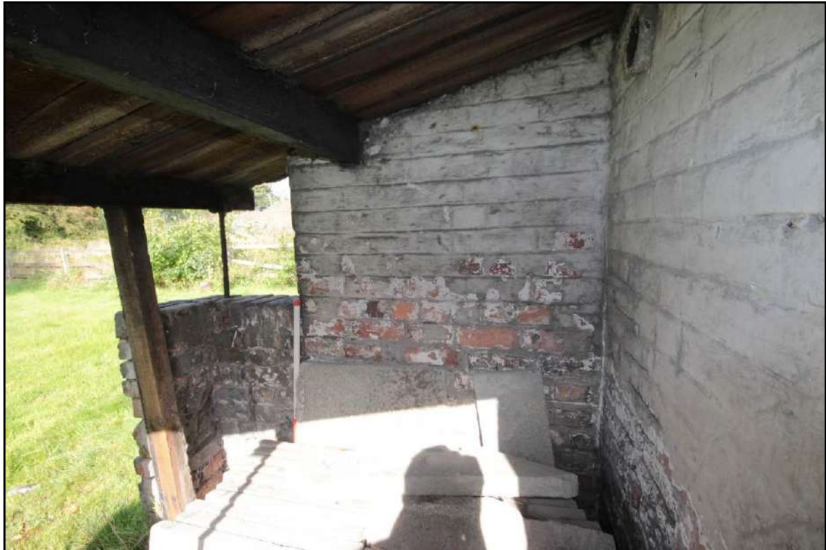
Photograph 82: View of the northern wall of Room 4, taken with 1m scale facing north (File: HBR_132)
