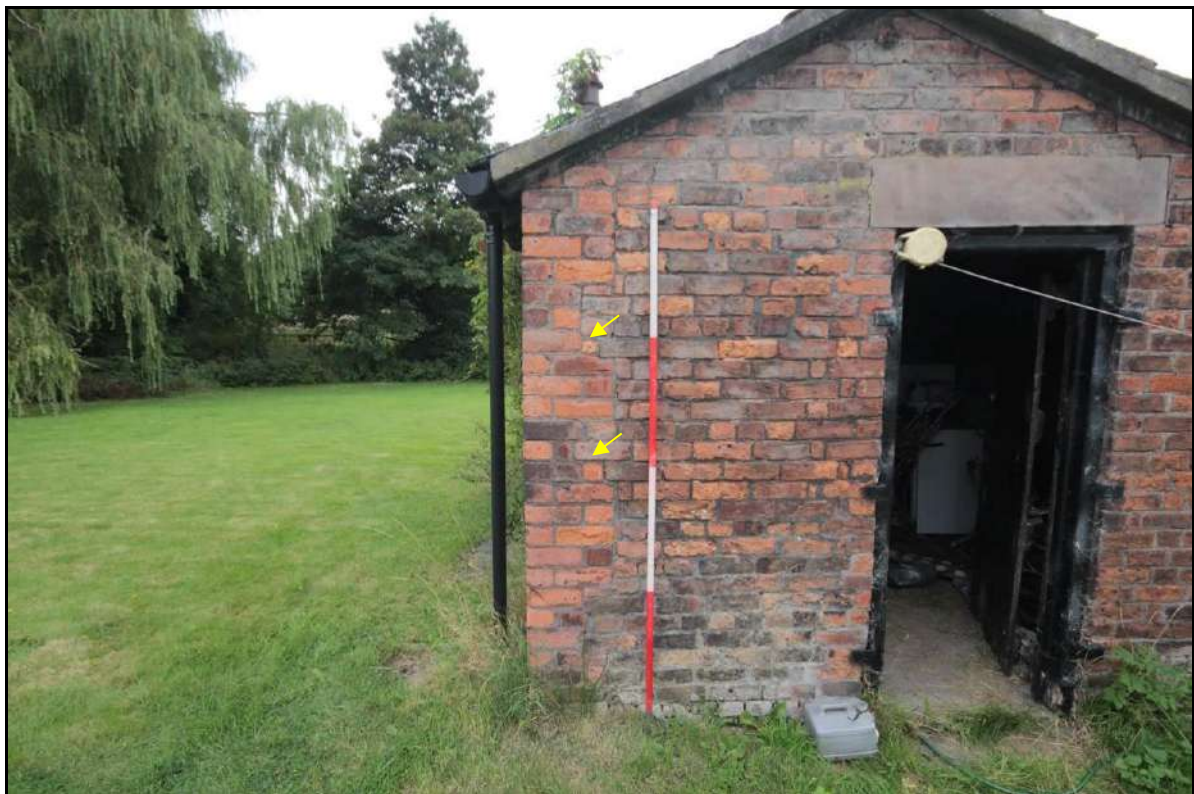
Photograph 48: View of the straight joints of the outbuilding's eastern elevation, delineating the two phases of brickwork. Taken facing west with 2m scale (File: HBR_74)
