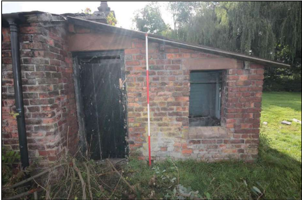
Photograph 41: View of the western extent of the outbuilding's northern elevation, taken with 2m scale facing south (File: HBR_63)
