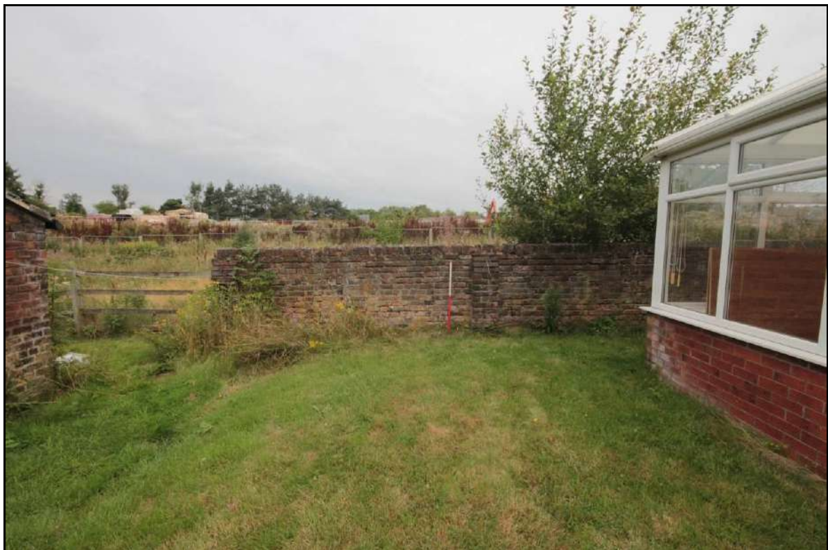
Photograph 16: View of the brick wall attached to the western side of the former Dye House, taken with 1m scale facing north (File: HBR_21)
