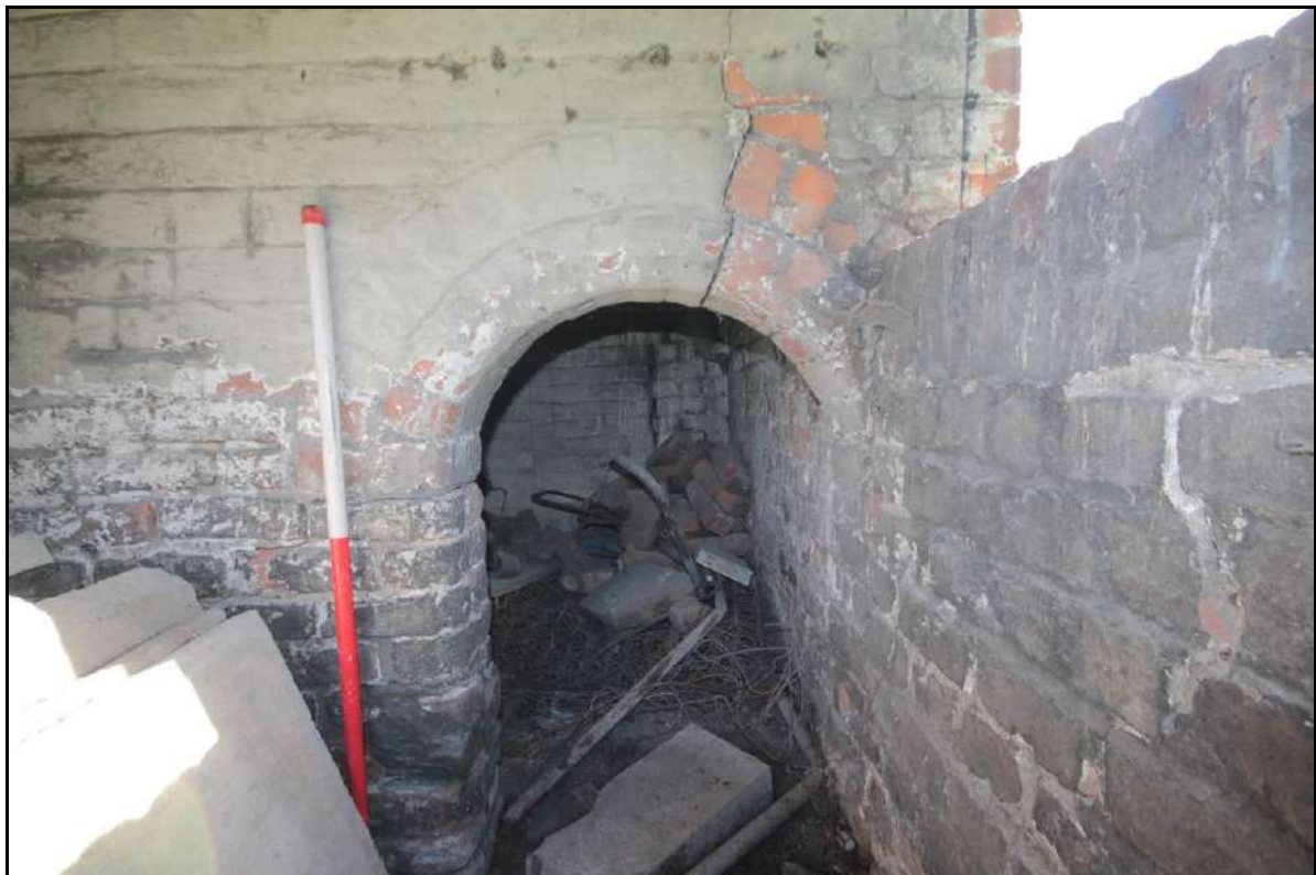
Photograph 81: View of the semi-circular arched aperture on the eastern wall of Room 4, taken with 1m scale facing east (File: HBR_126)
