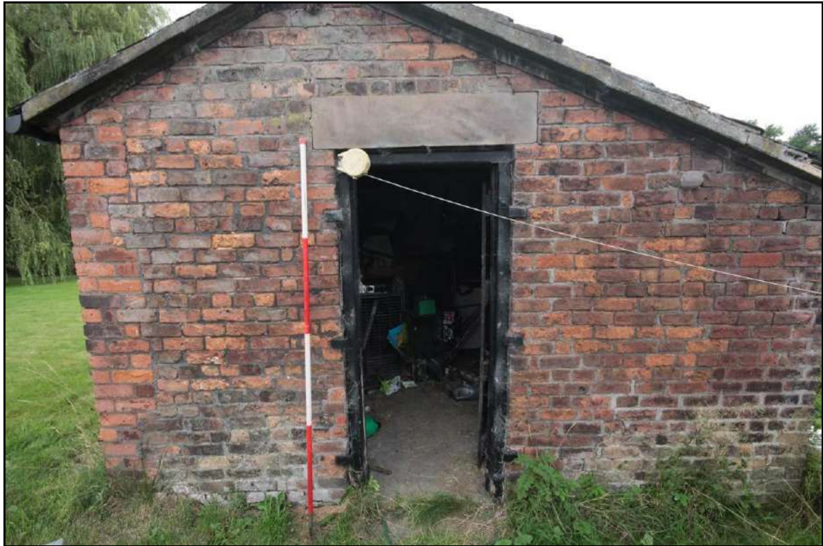
Photograph 47: View of the doorway of the outbuilding's eastern elevation, taken facing west with 2m scale (File: HBR_76)
