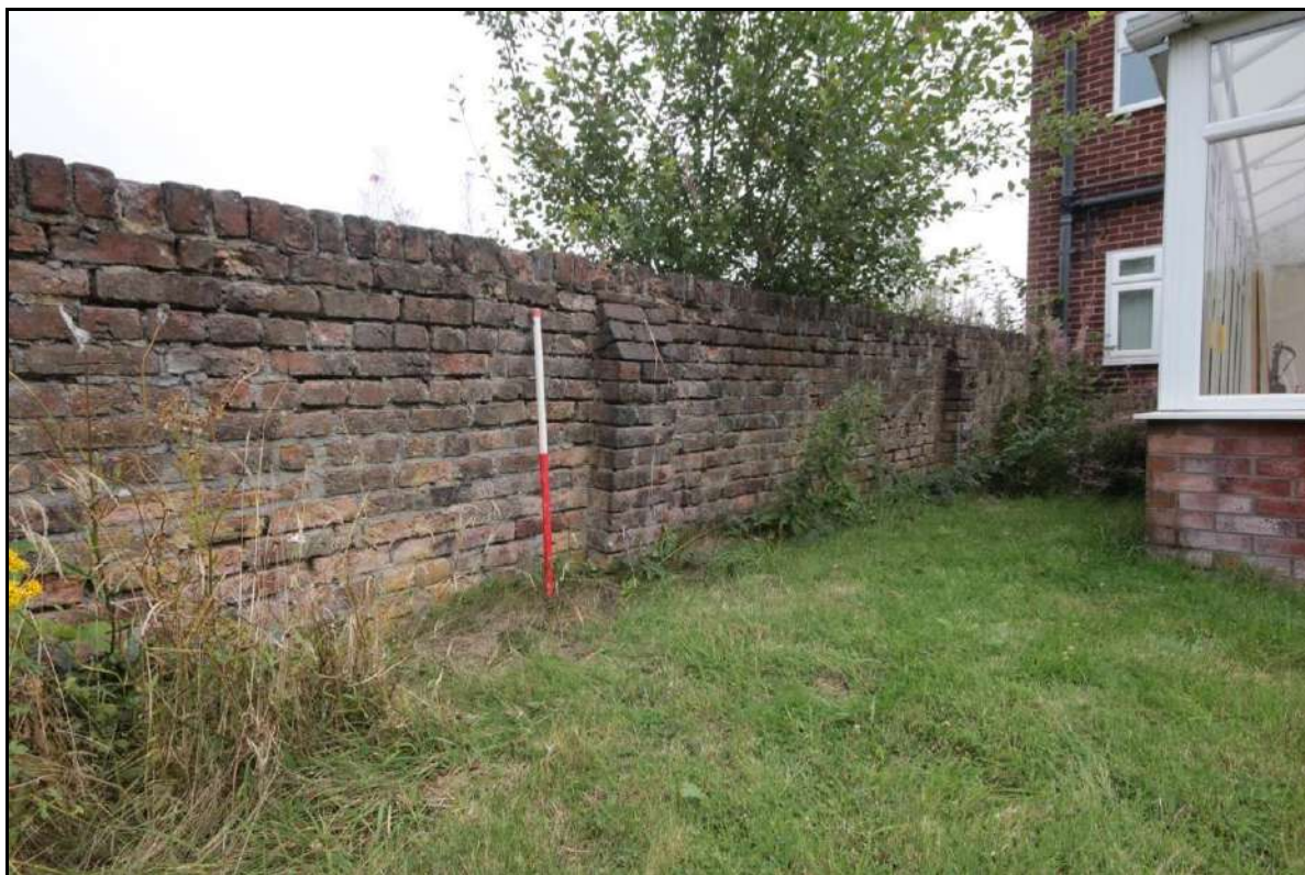
Photograph 17: Oblique view of the brick wall attached to the western side of the former Dye House, taken with 1m scale facing north-east (File: HBR_22)
