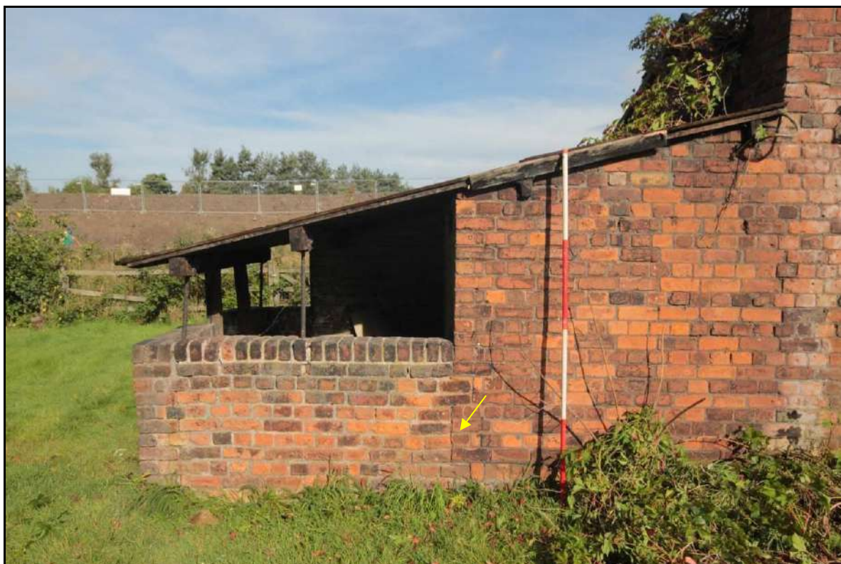
Photograph 34: View of the western end of the outbuilding's southern elevation, with straight joint of the low brick wall highlighted, which delineates its later phase. Taken with 2m scale facing north (File: HBR_44)
