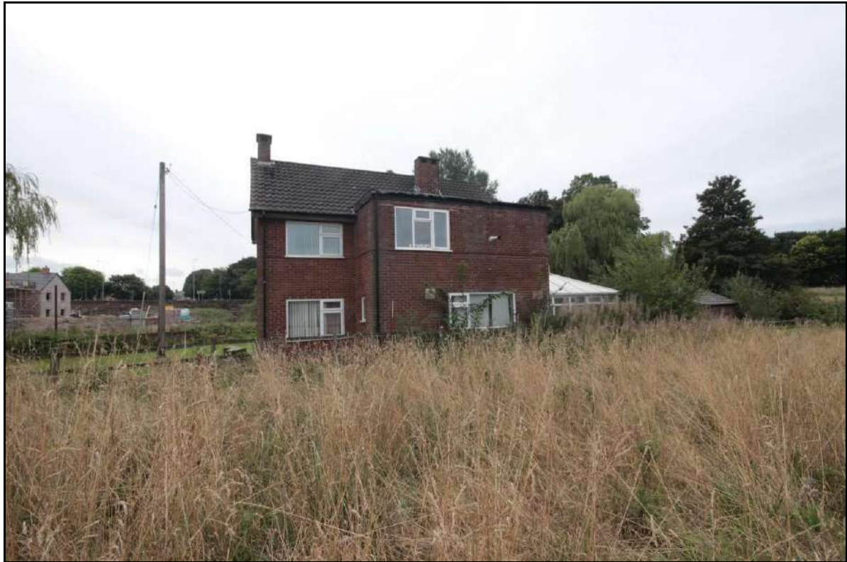
Photograph 15: View of the northern side of the former Dye House, taken facing south with 2m scale (File: HBR_18)
