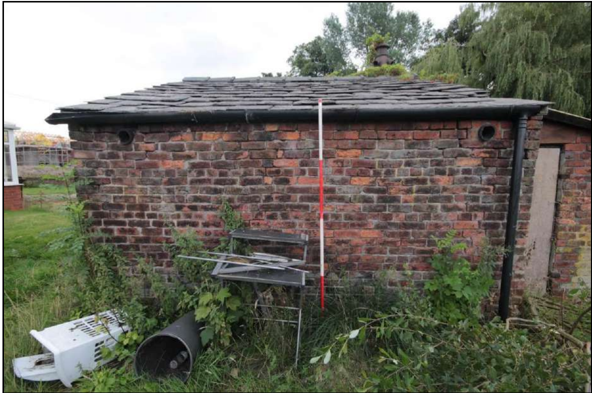
Photograph 43: View of the eastern extent of the outbuilding's northern elevation, taken facing south with 2m scale (File: HBR_66)
