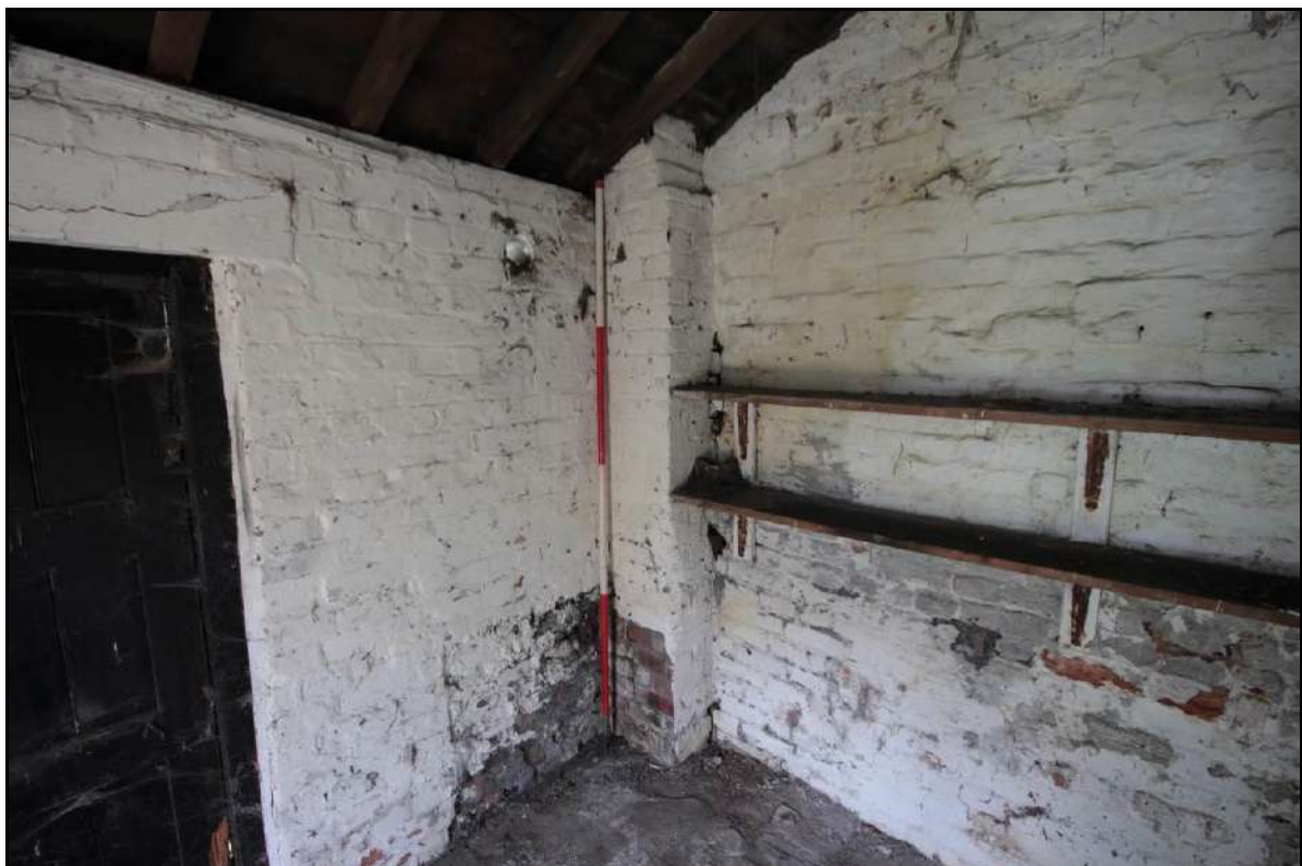
Photograph 55: View of the buildout within the south-western corner of Room 1, taken facing south-west with 2m scale (File: HBR_82)
