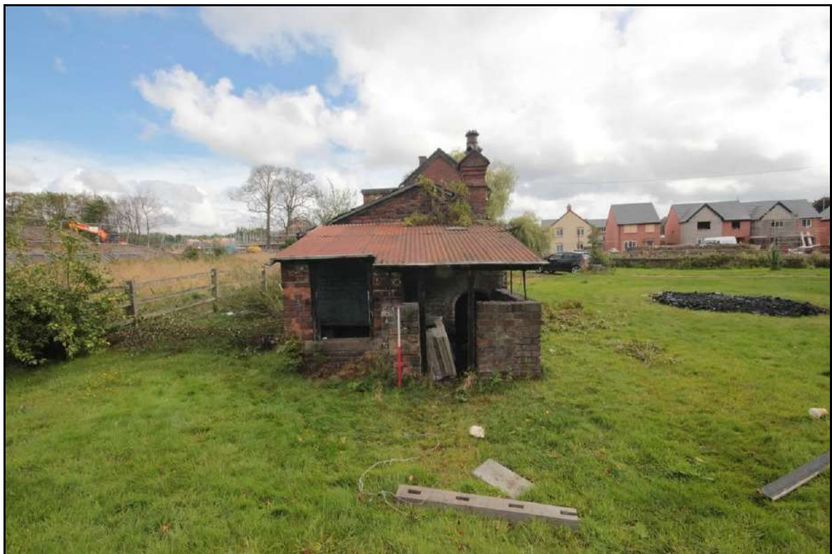
Photograph 36: Central view of the outbuilding's western elevation, taken facing east with 1m scale (File: HBR_46)
