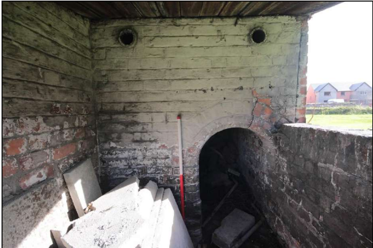
Photograph 80: View of Room 4's eastern wall, taken facing east with 1m scale (File: HBR_125)
