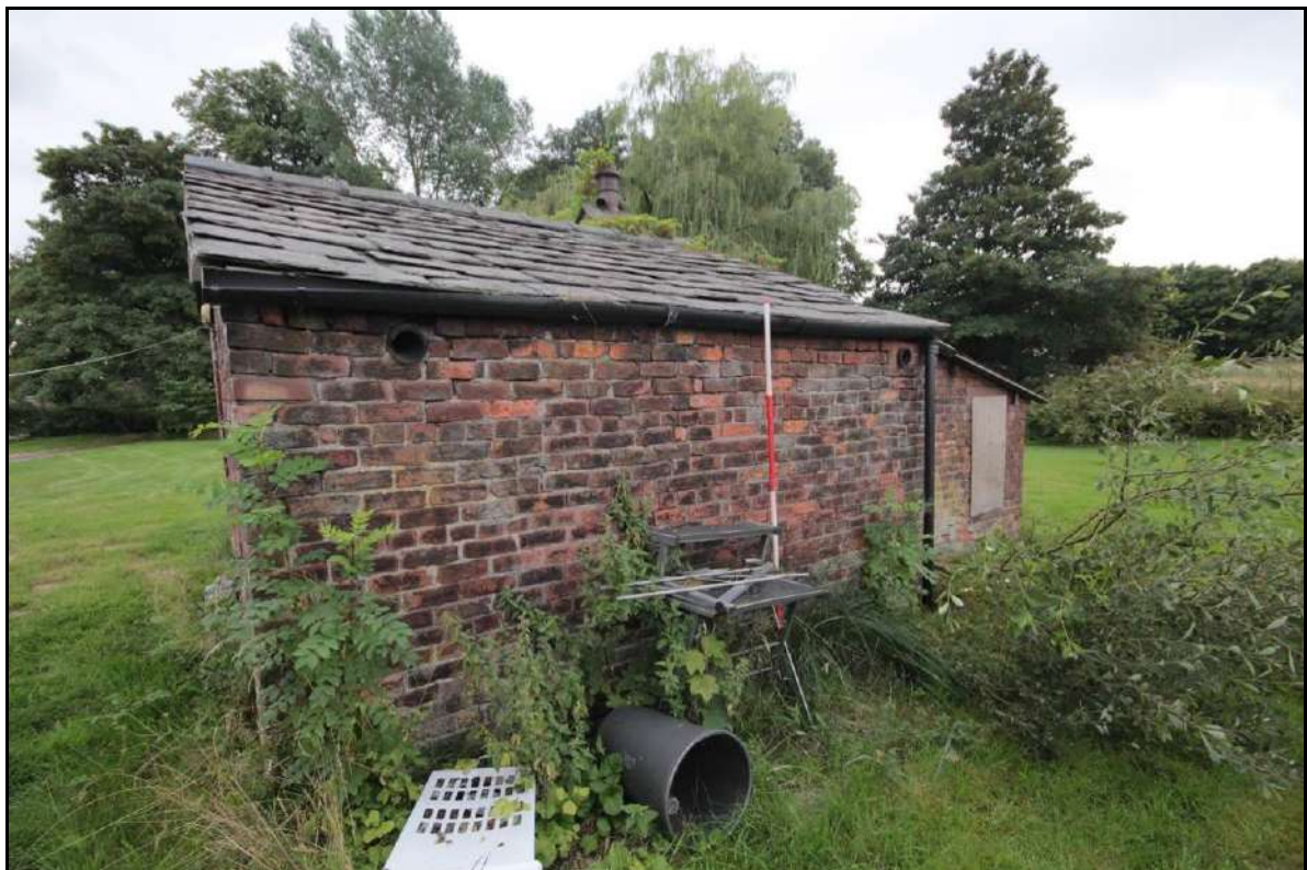
Photograph 40: Oblique view of the outbuilding's northern elevation, taken with 2m scale facing south-west (File: HBR_65)
