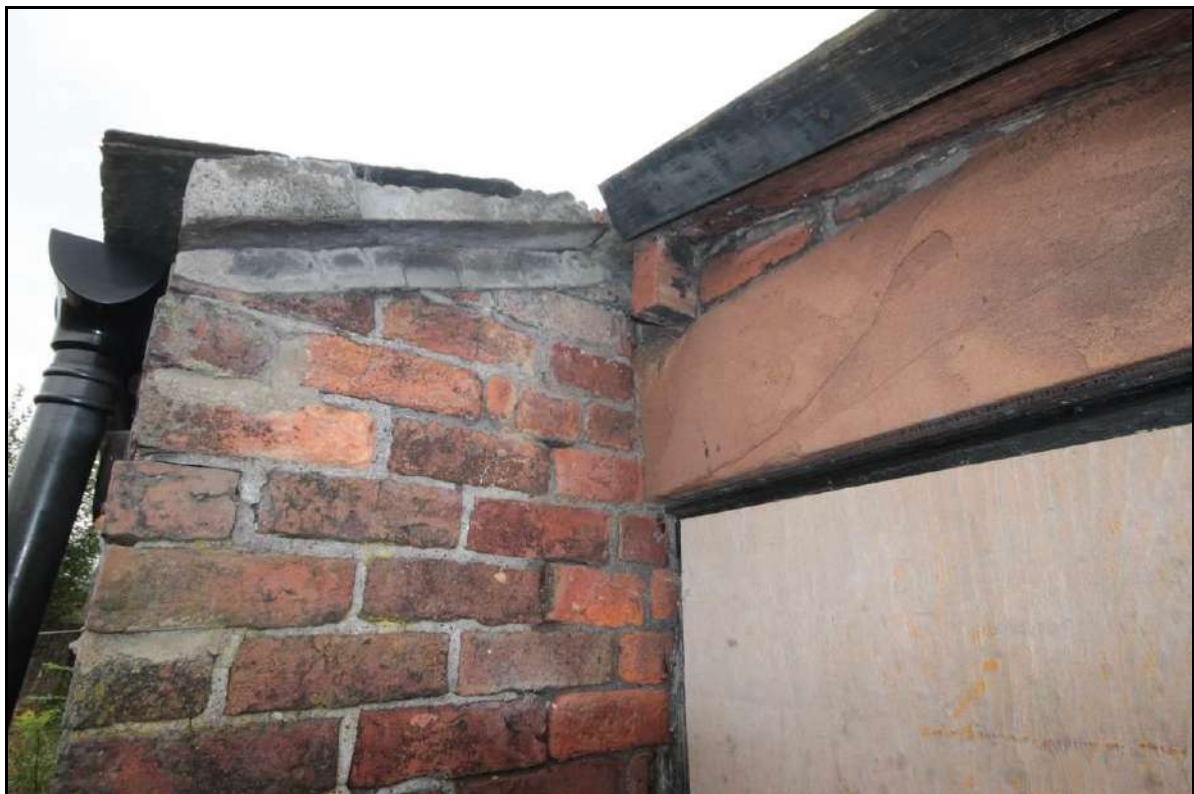
Photograph 42: View of the doorway lintel of the outbuilding's northern elevation, built into the pitched structure's western wall, taken facing south-east (File: HBR_61)
