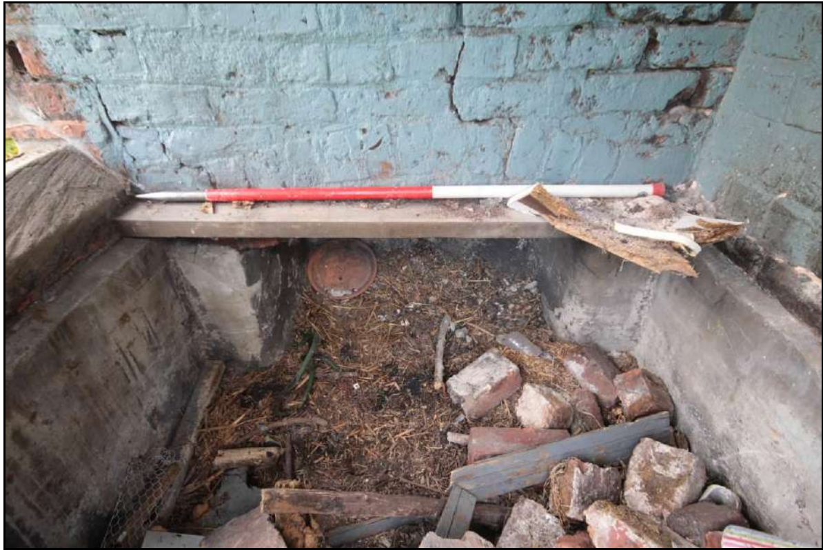
Photograph 70: View of the aperture connecting with the privy of Room 2, on the eastern wall of Room 3, taken with 1m scale facing east (File: HBR_115)
