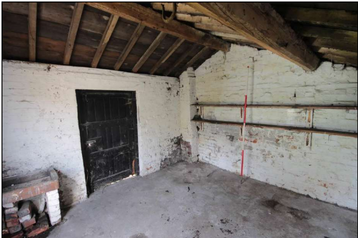
Photograph 49: General view to the south-west within Room 1, taken with 2m scale (File: HBR_77)
