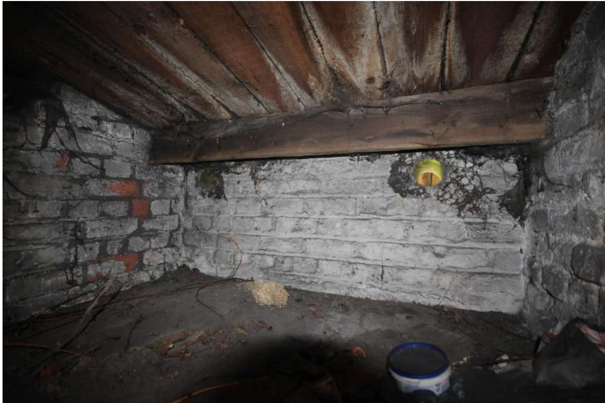
Photograph 94: Oblique view of Room 6's western wall, taken facing south-west (File: HBR_113)
