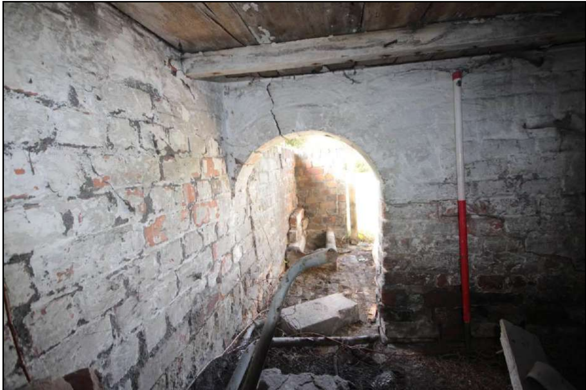
Photograph 89: View of the semi-circular archway on the western wall of Room 5, taken with 1m scale facing west (File: HBR_134)
