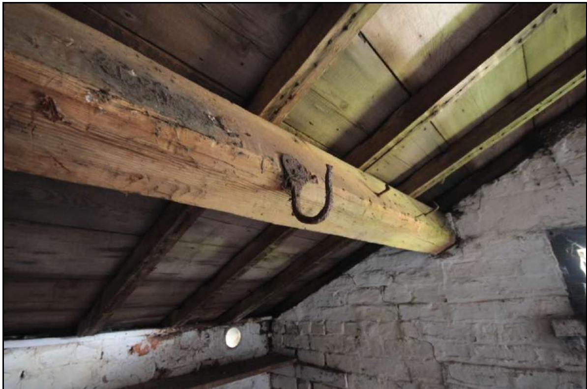
Photograph 51: View of the hook fixture on the northern purlin within Room 1, taken facing north-east (File: HBR_87)
