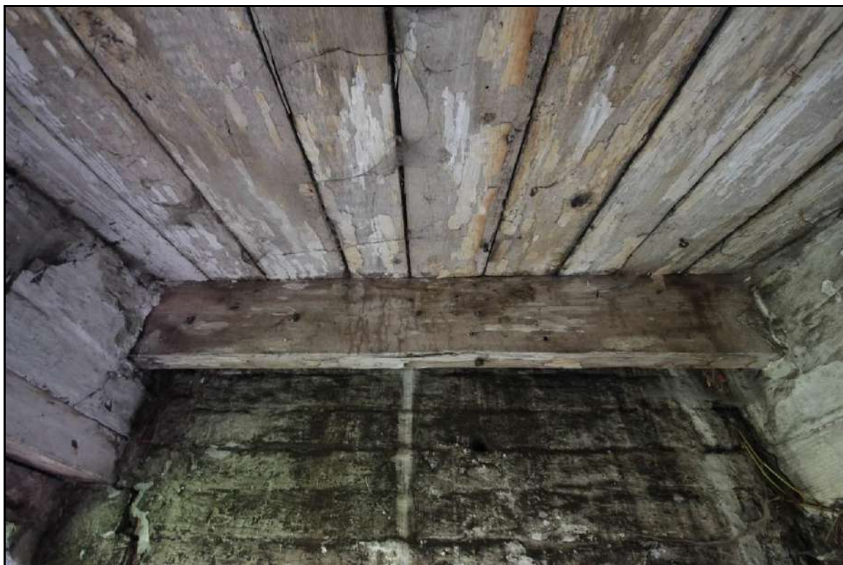
Photograph 61: View of the roof structure within Room 2, taken facing east (File: HBR_97)
