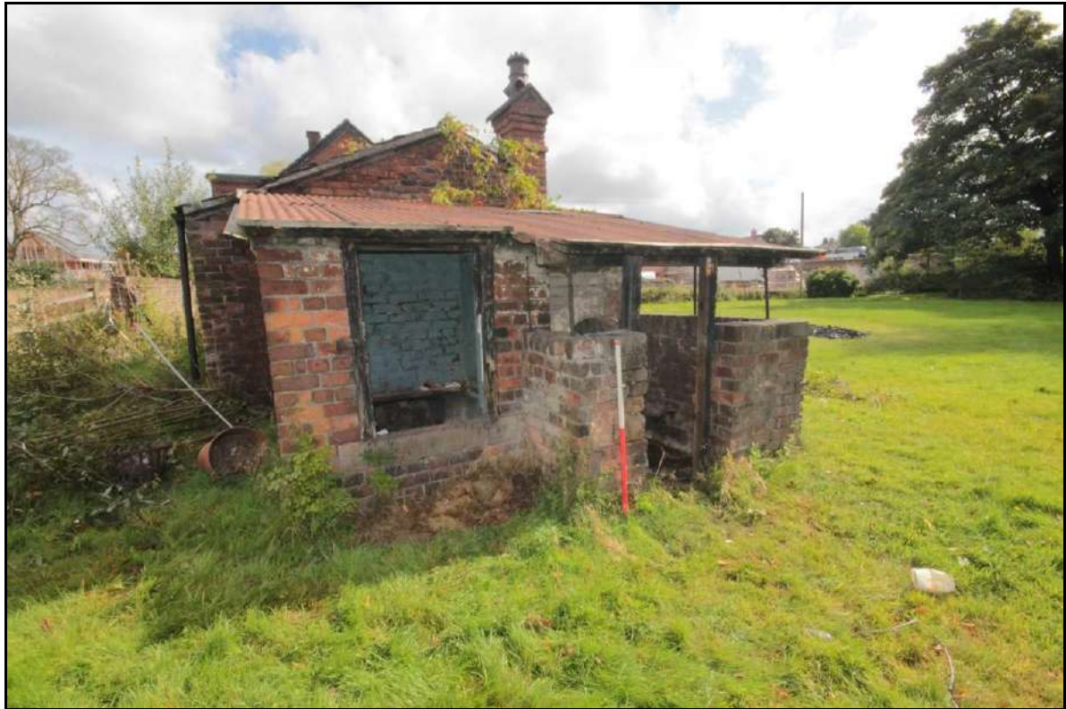
Photograph 35: Oblique view of the outbuilding's western elevation, taken with 1m scale facing south-east (File: HBR_52)
