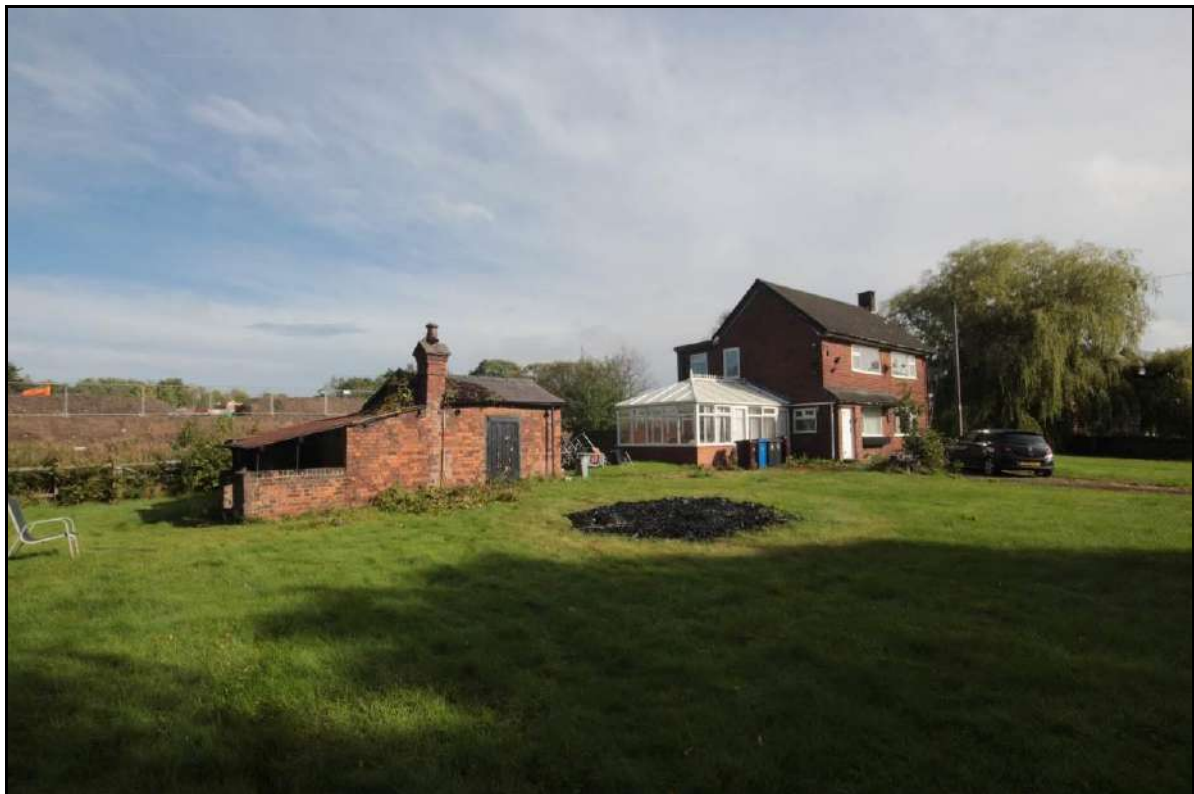
Photograph 5: View of the Dye House and Outbuilding, taken facing north-east from the western extent of the site (File: HBR_23)
