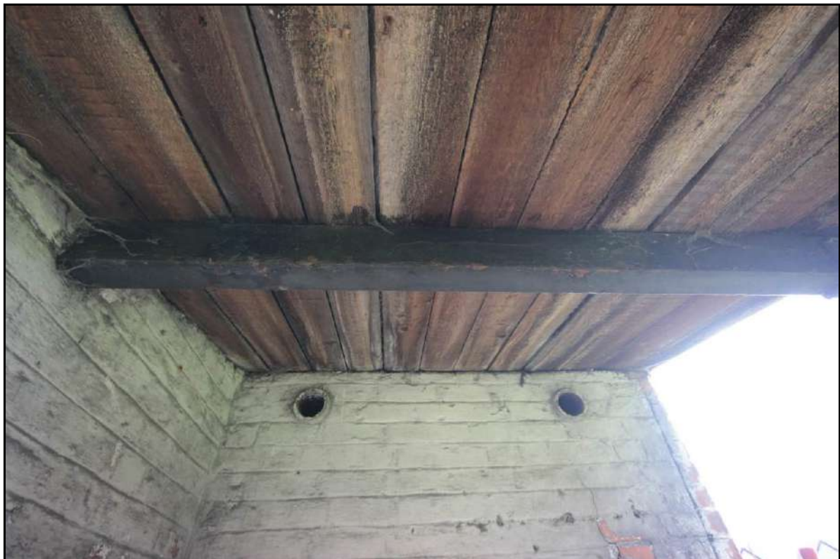
Photograph 75: View of Room 4's roof structure, taken facing east (File: HBR_122)
