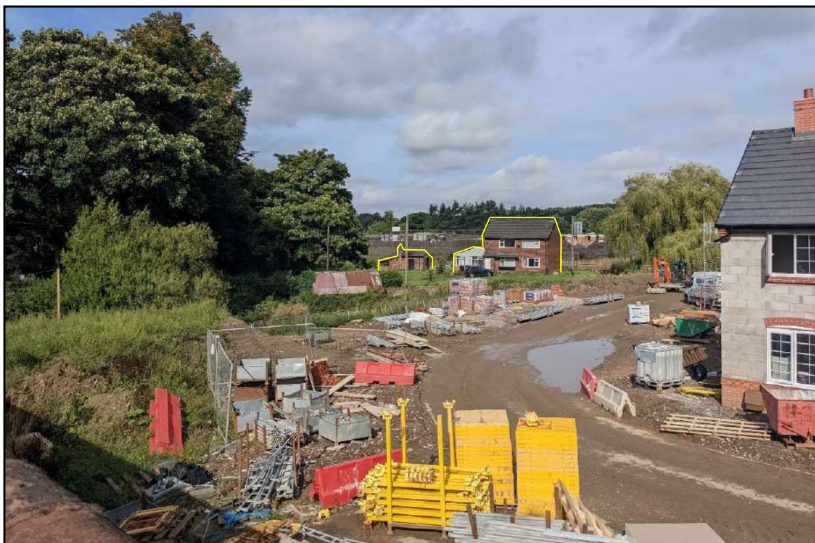
Photograph 11: View of the former Dye House and Outbuilding (highlighted) from Liverpool Road to the south-east, taken facing north-west
