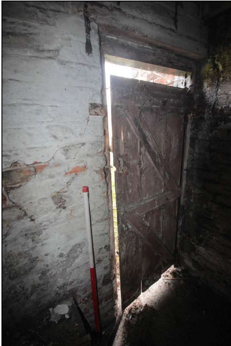
Photograph 65: Oblique view of Room 2's northern wall, taken with 1m scale facing north-east (File: HBR_103)
