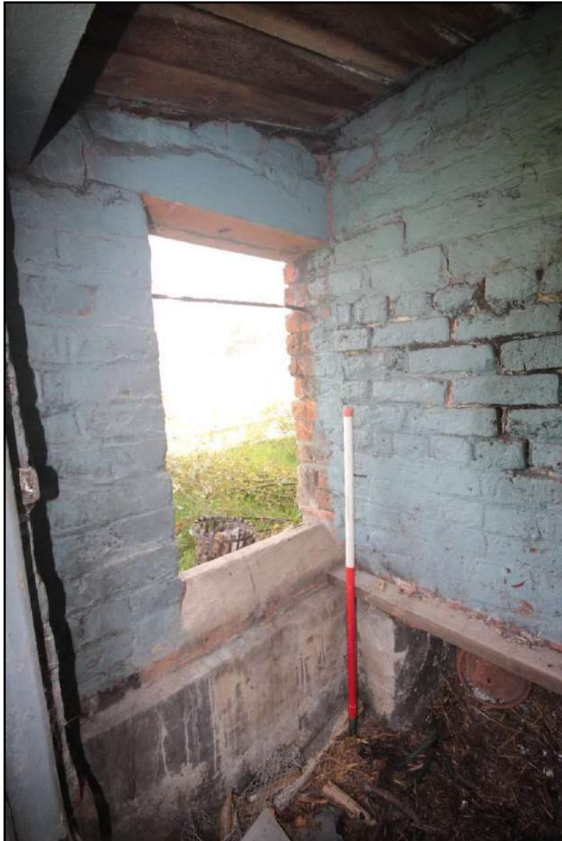
Photograph 72: View of the northern wall of Room 3, taken with 1m scale facing north-east (File: HBR_120)
