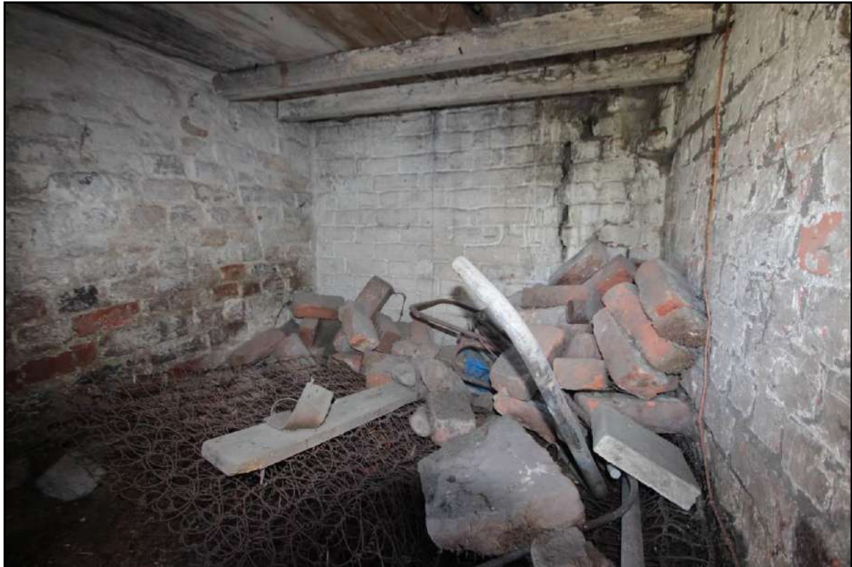
Photograph 83: General view to the east within Room 5 (File: HBR_136)
