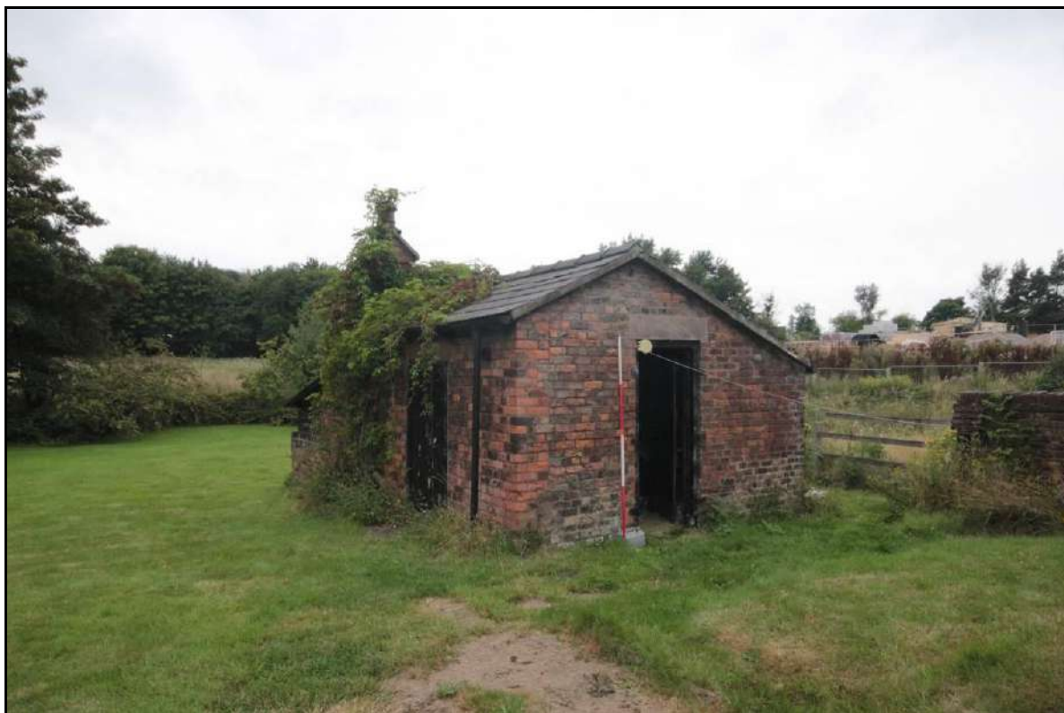
Photograph 45: Oblique view of the outbuilding's eastern elevation, taken facing north-west with 2m scale (File: HBR_72)
