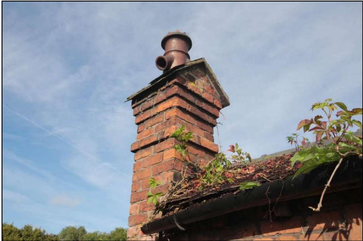
Photograph 27: View of the chimneystack of the outbuilding's pitched roof, taken facing north-west (File: HBR_43)
