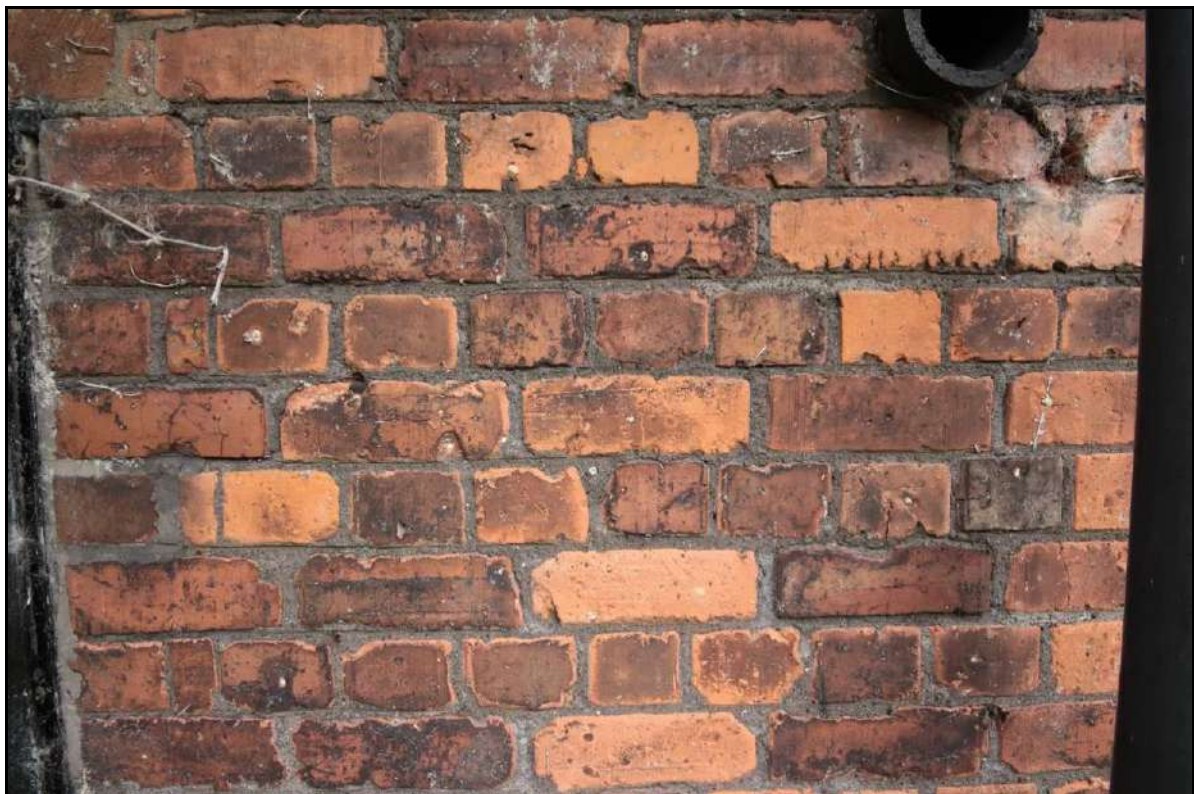
Photograph 28: View of the brick used in the southern and western walls of the outbuilding, taken facing north (File: HBR_39)
