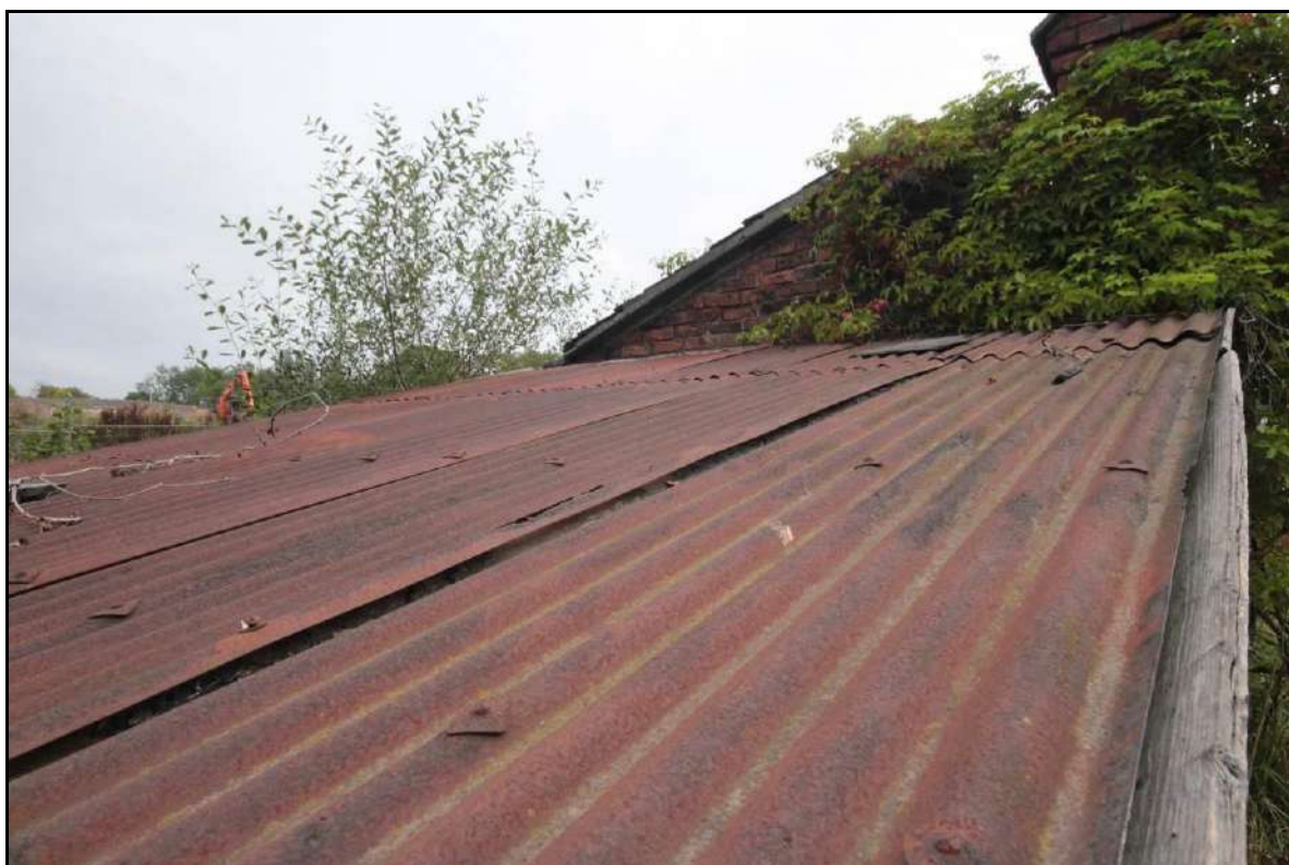
Photograph 26: View of the corrugated roofing sheets of the outbuilding's lean-to, taken facing north-east (File: HBR_56)
