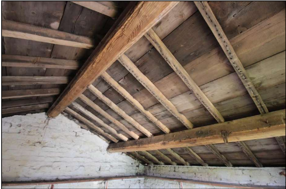
Photograph 50: View of the roof structure within Room 1, taken facing north-west (File: HBR_79)
