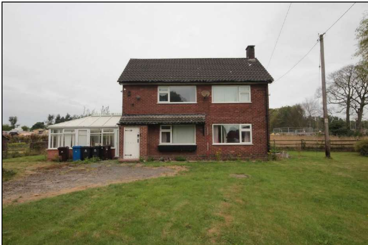
Photograph 12: View of the former Dye House, taken with 2m scale facing north (File: HBR_17)
