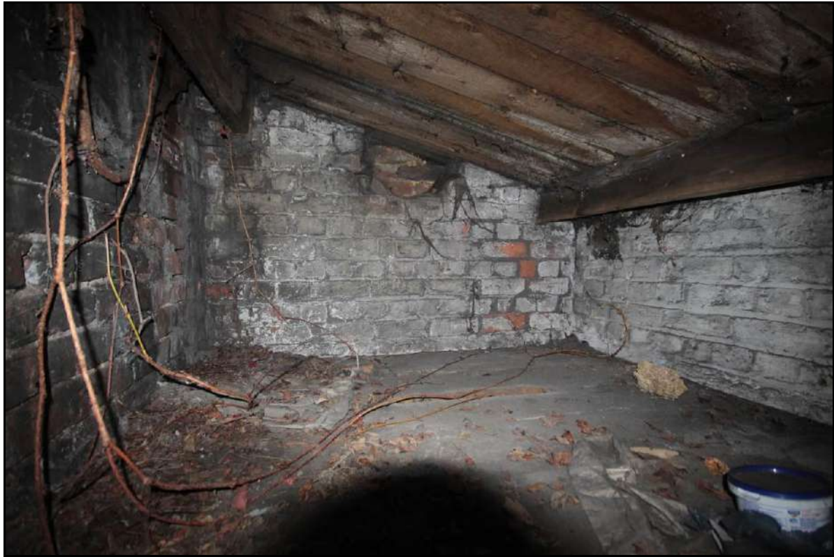
Photograph 90: General view to the south within Room 6 (File: HBR_107)
