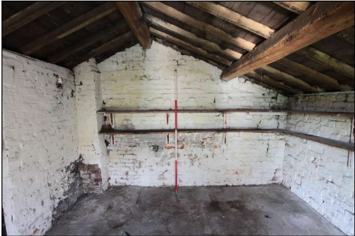
Photograph 54: View of Room 1's western wall, taken facing west with 2m scale (File: HBR_81)
