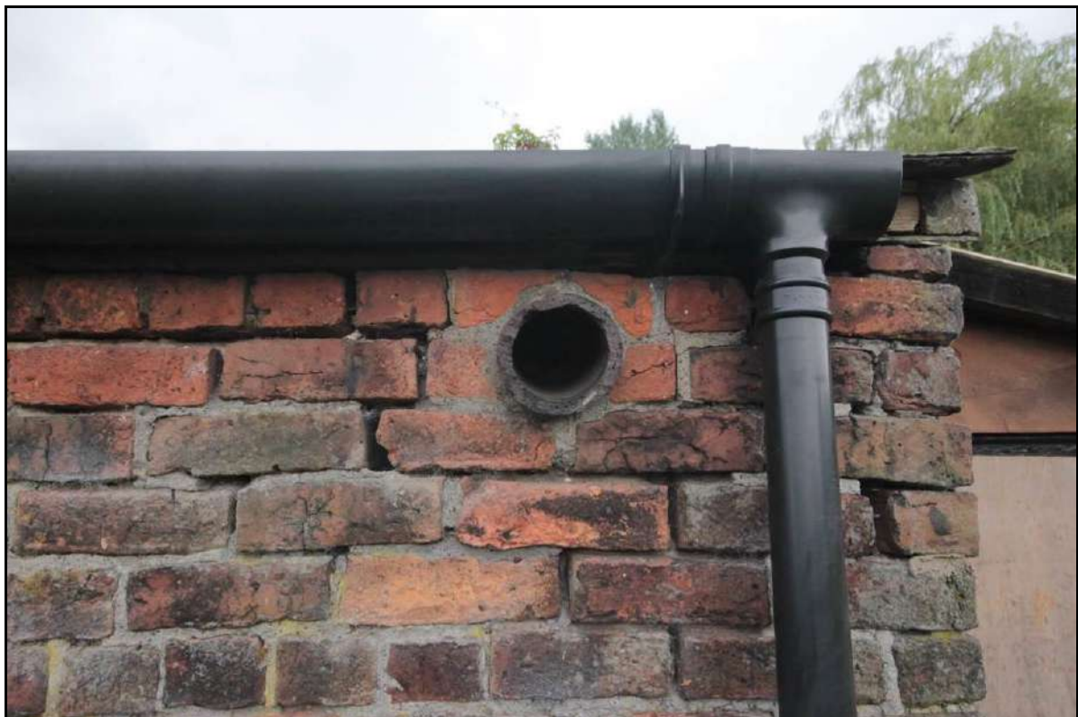
Photograph 44: View of one of the inserted vents of the outbuilding's northern elevation, taken facing south (File: HBR_70)
