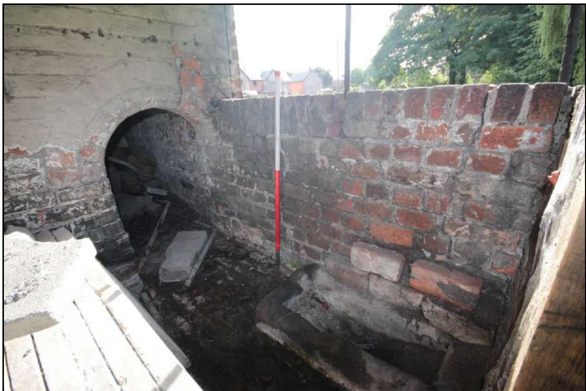
Photograph 79: Oblique view of Room 4's southern wall, taken with 1m scale facing south-east (File: HBR_129)
