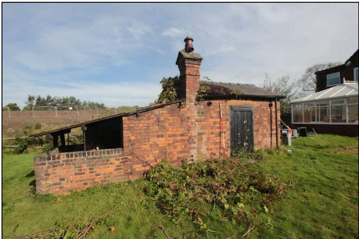
Photograph 30: Oblique view of the outbuilding's southern elevation, taken facing north-east with 2m scale (File: HBR_37)
