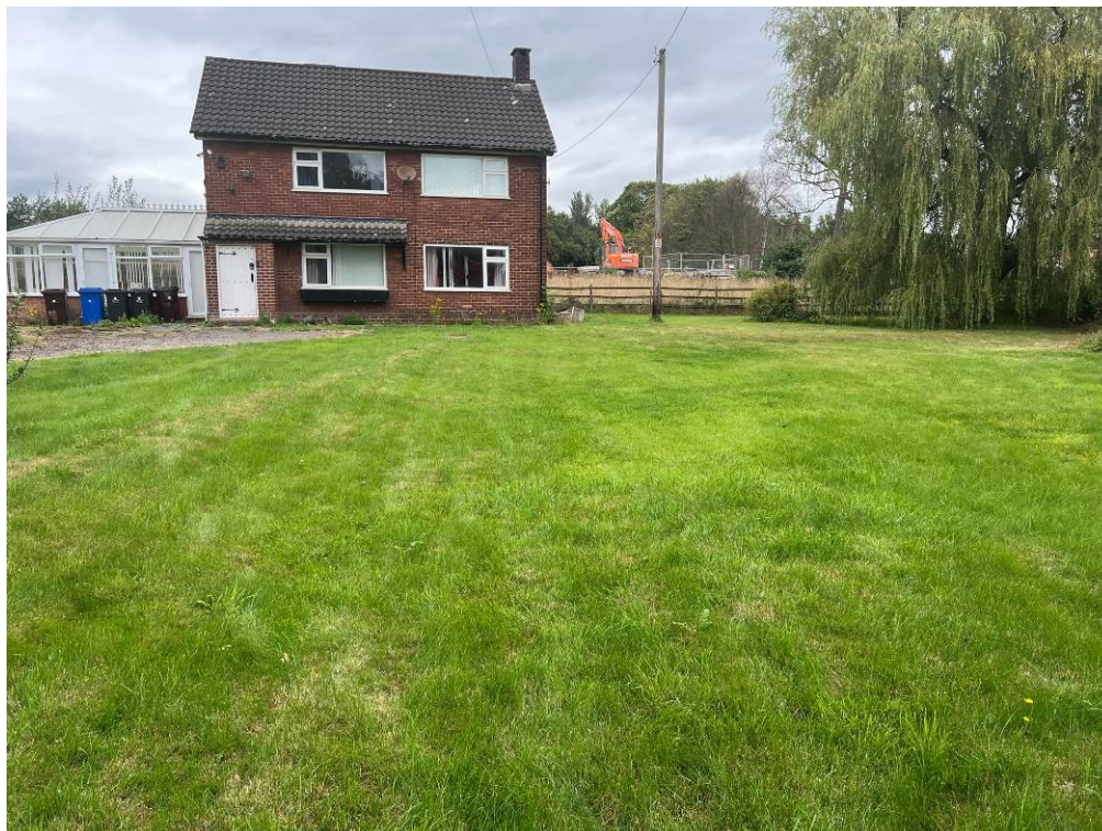
Photo 3; Looking north to Dye House from grasses garden area.
