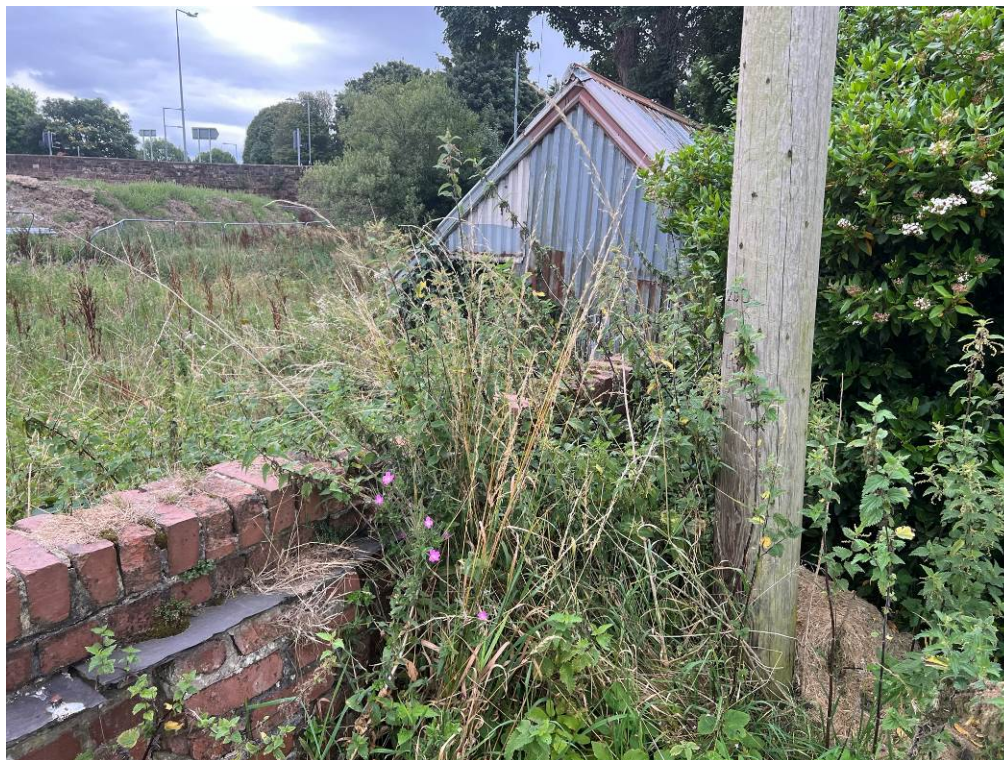
Photo 5; Metal clad outbuilding.
