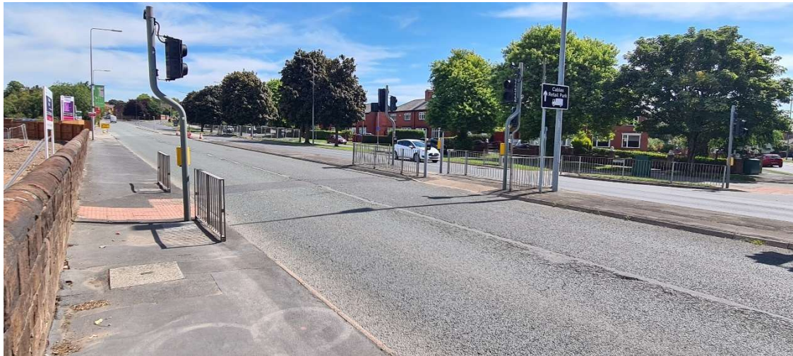
Figure 2.3 – Existing Liverpool Road Pedestrian Infrastructure
