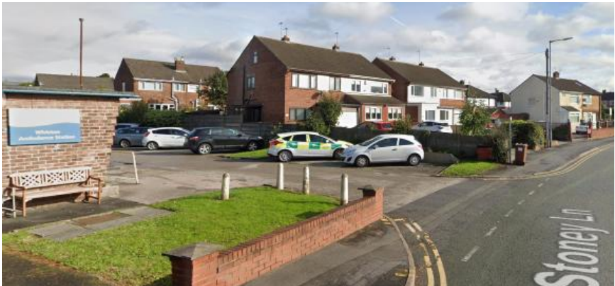
3. Stoney Lane, Newby Ave Junction to east of site
