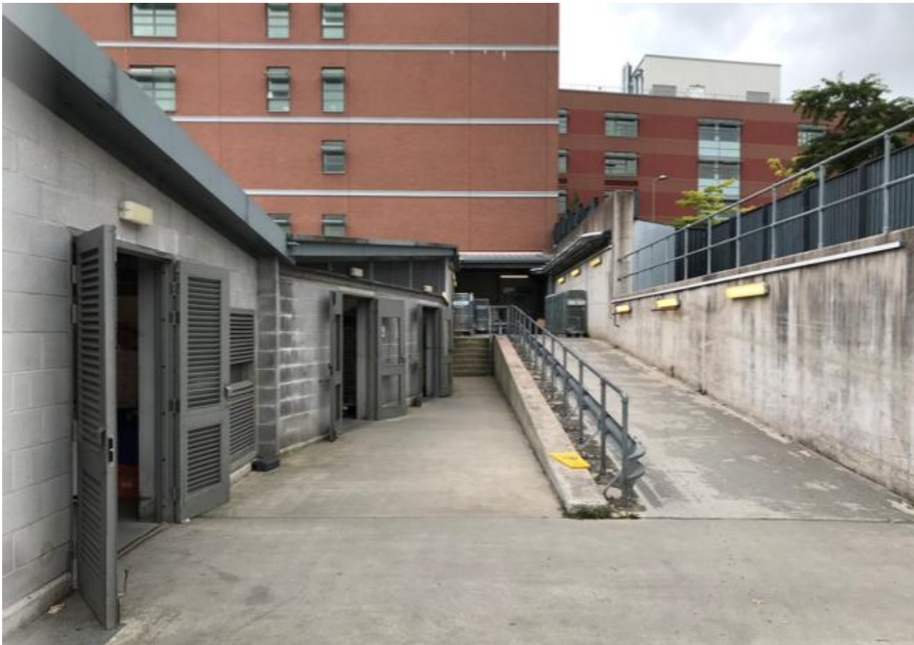
Existing operations - bin stores, ramp, retaining wall
