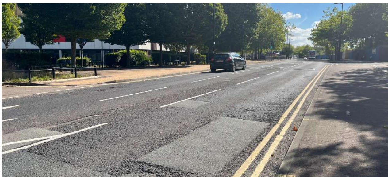
Photograph 2.3 : Cherryfield Drive (eastbound)
