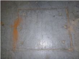
Cover seized in frame Section SW 52
