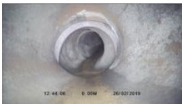
Displaced joint Section SW 29
