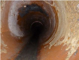
Rainwater pipe missing Section SW 1
