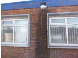
Rainwater pipe missing
