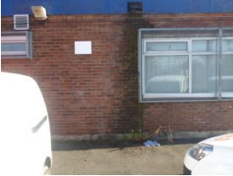
Rainwater pipe missing
