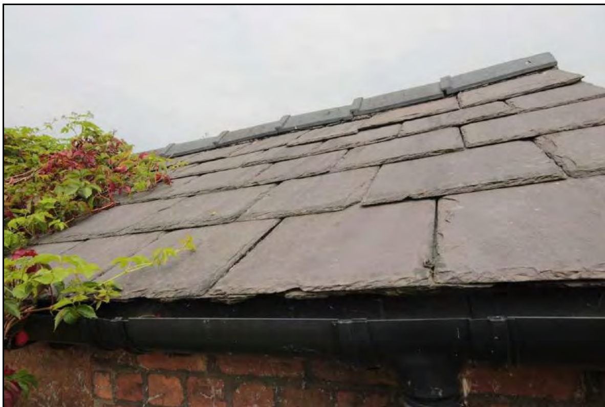
Photograph 25: View of the pitched slate roof of the outbuilding, taken facing north-west (File: HBR_55)
