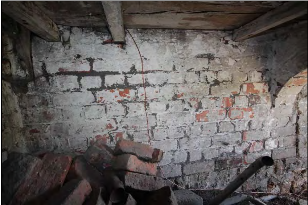
Photograph 87: View of the southern wall of Room 5, taken facing south (File: HBR_135)
