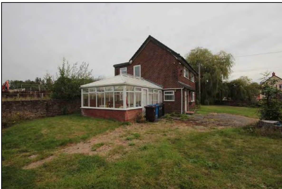
Photograph 14: View of the western extent of the former Dye House, taken with 2m scale facing north-east (File: HBR_19)
