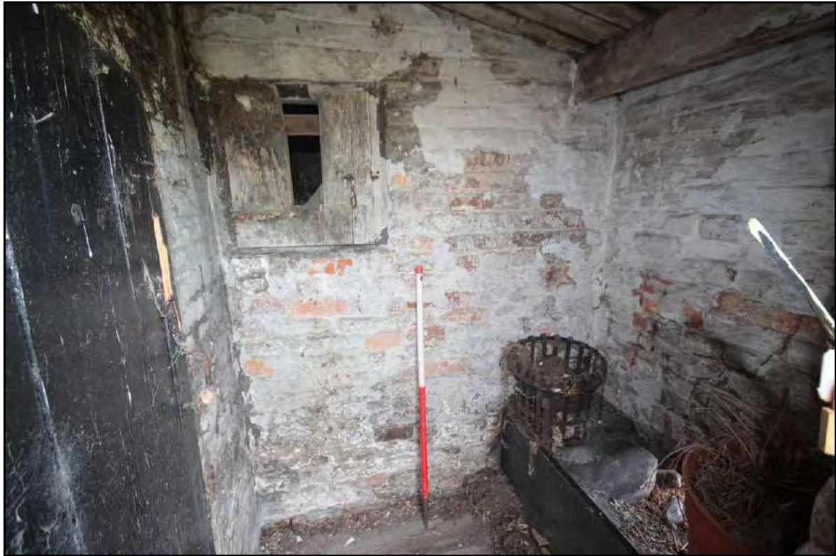
Photograph 60: General view into Room 2, taken with 1m scale facing south (File: HBR_96)
