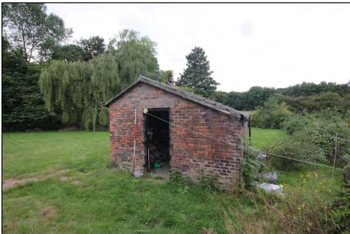
Photograph 46: Oblique view of the outbuilding's eastern elevation, taken facing south-west with 2m scale (File: HBR_73)
