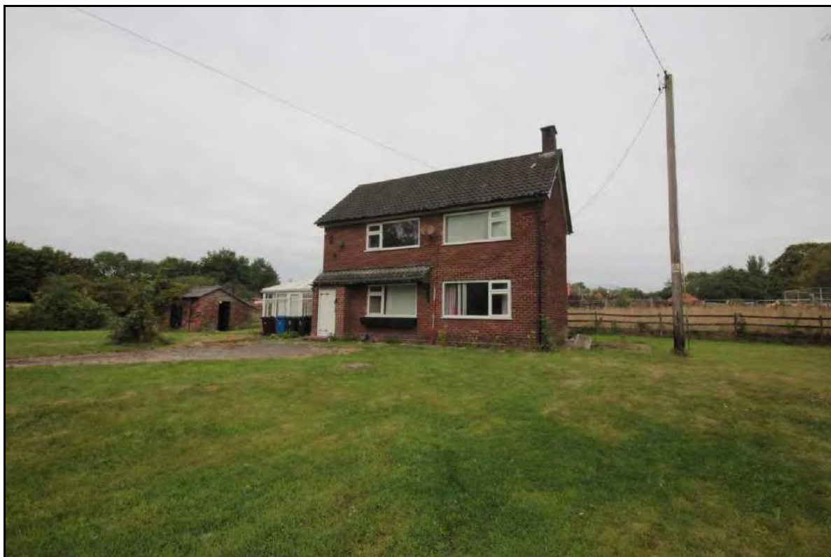
Photograph 13: Oblique view of the former Dye House, taken facing north-west with 2m scale (File: HBR_12)
