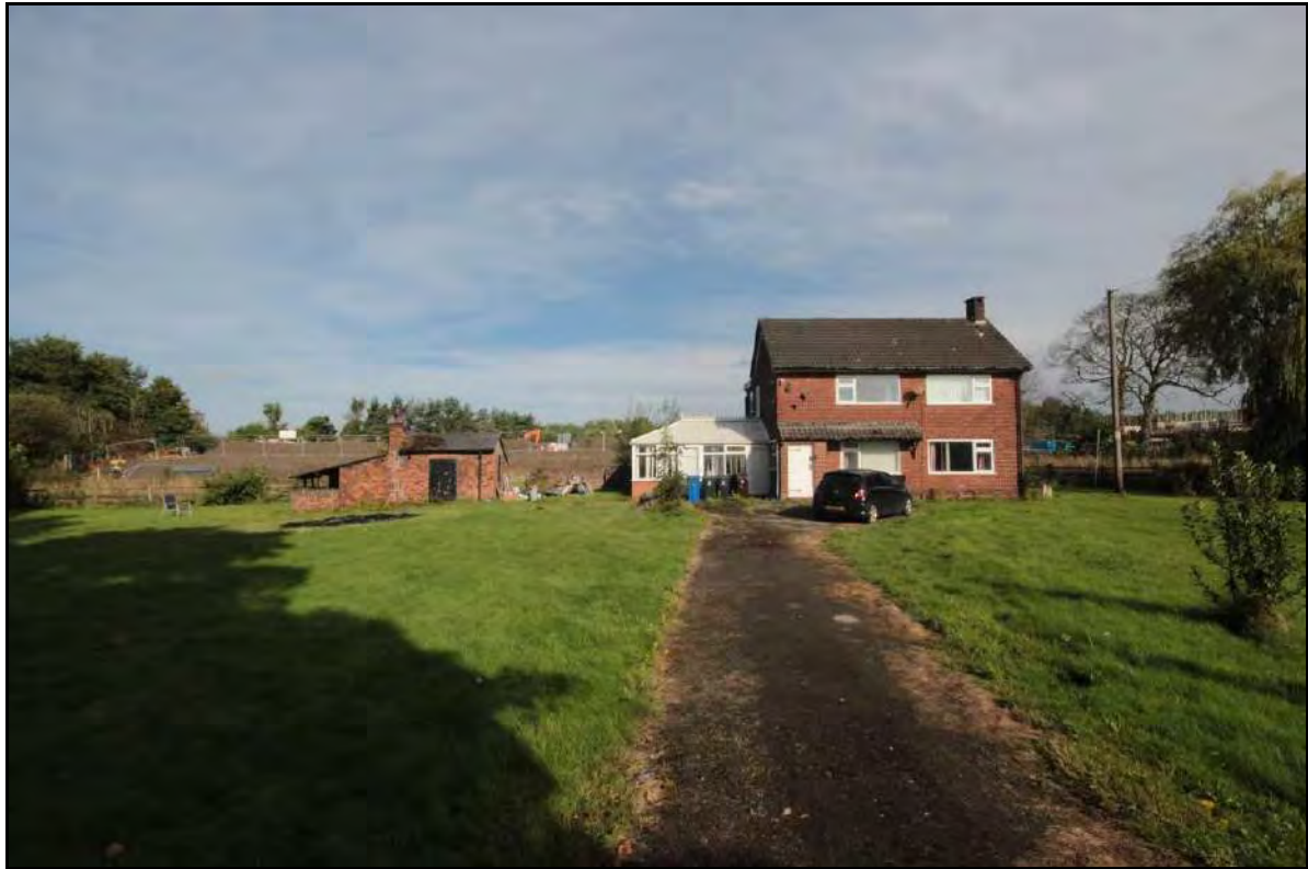
Photograph 4: View of the former Dye House and Outbuilding, situated within the northern extent of the site, taken facing north (File: HBR_24)
