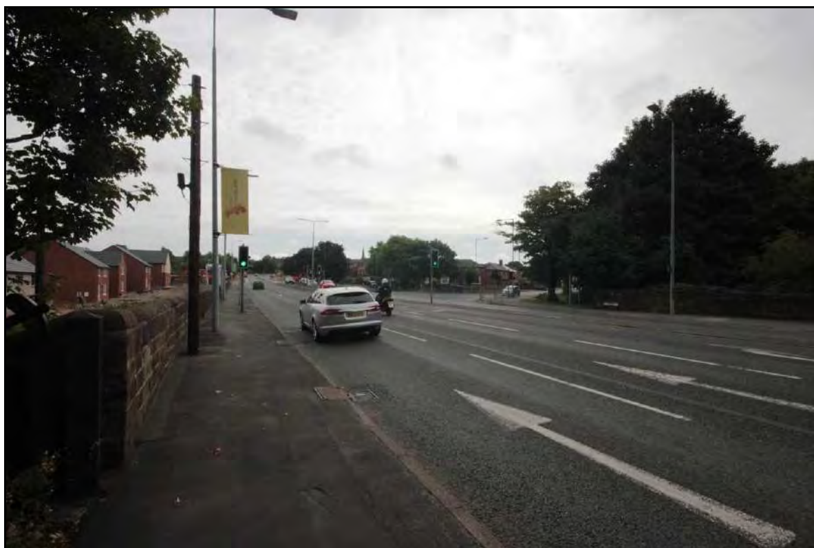
Photograph 1: View to the east on Liverpool Road, from the access point to the site (File: HBR_1)
