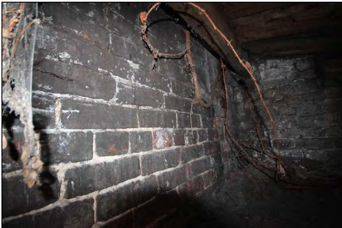
Photograph 95: View of the eastern wall of Room 6, taken facing south-east (File: HBR_110)
