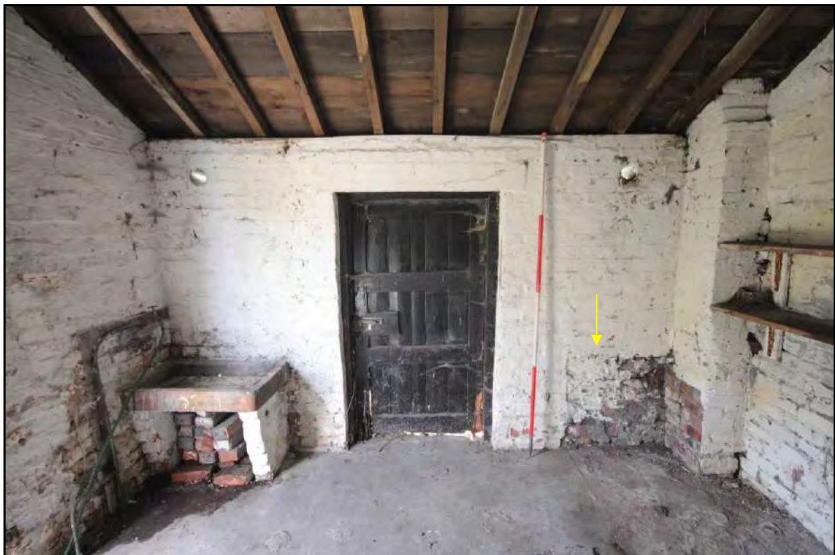
Photograph 59: View of the southern wall of Room 1, with scarring associated with an earlier brick structure highlighted. Taken facing south with 2m scale (File: HBR_91)
