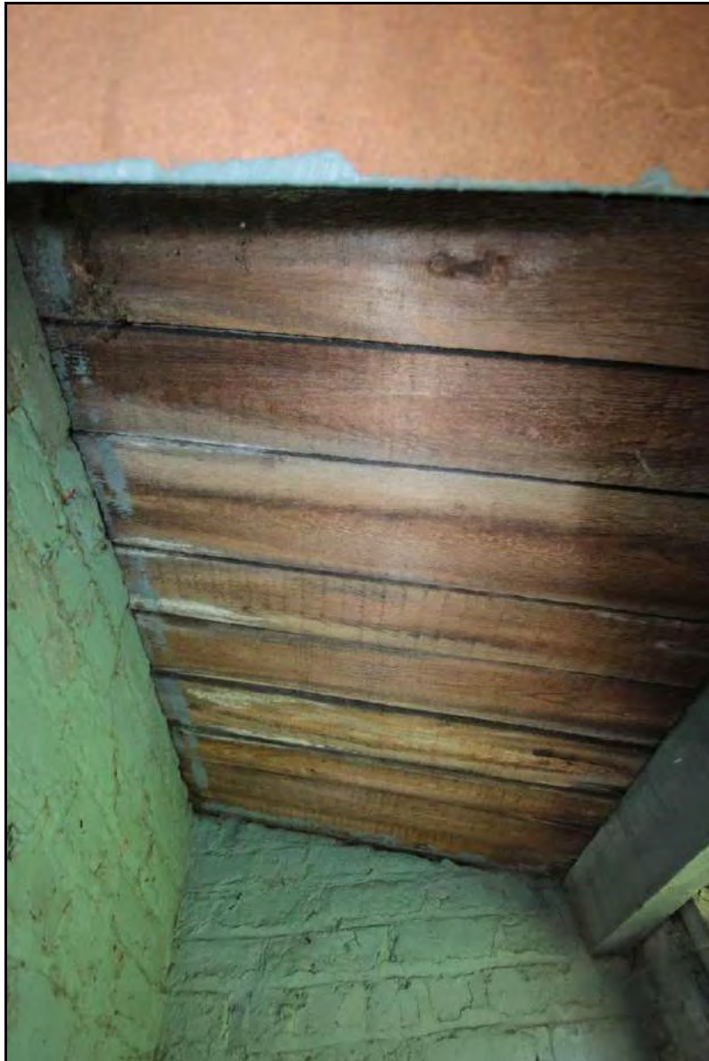
Photograph 69: View of Room 3's roof structure, taken facing south (File: HBR_117)
