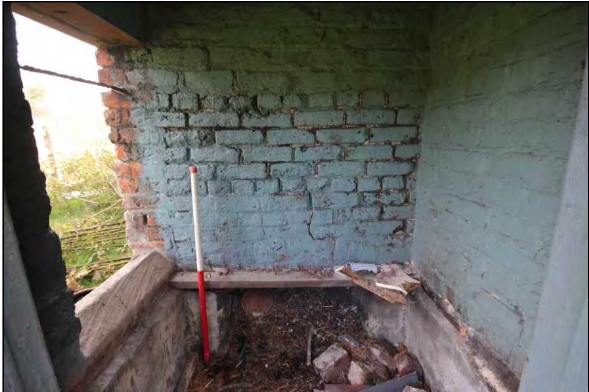
Photograph 68: View of the eastern wall of Room 3, taken with 1m scale facing east (File: HBR_114)
