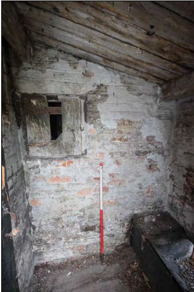
Photograph 66: View of Room 2's southern wall, taken facing south with 1m scale (File: HBR_105)
