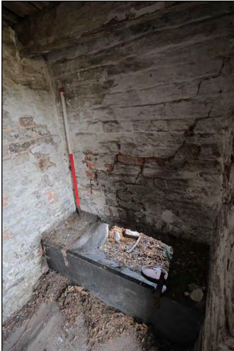
Photograph 63: Oblique view of Room 2's western wall, taken with 1m scale facing south-west (File: HBR_100)
