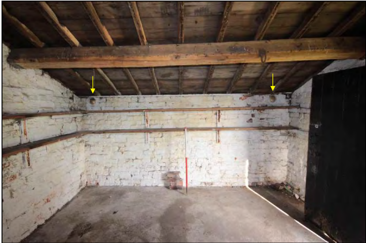
Photograph 56: View of the northern wall of Room 1, with vents highlighted, taken facing north with 1m scale (File: HBR_83)
