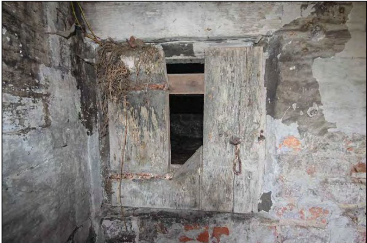
Photograph 67: View of the timber plank shutters on the southern wall of Room 2, taken facing south (File: HBR_106)
