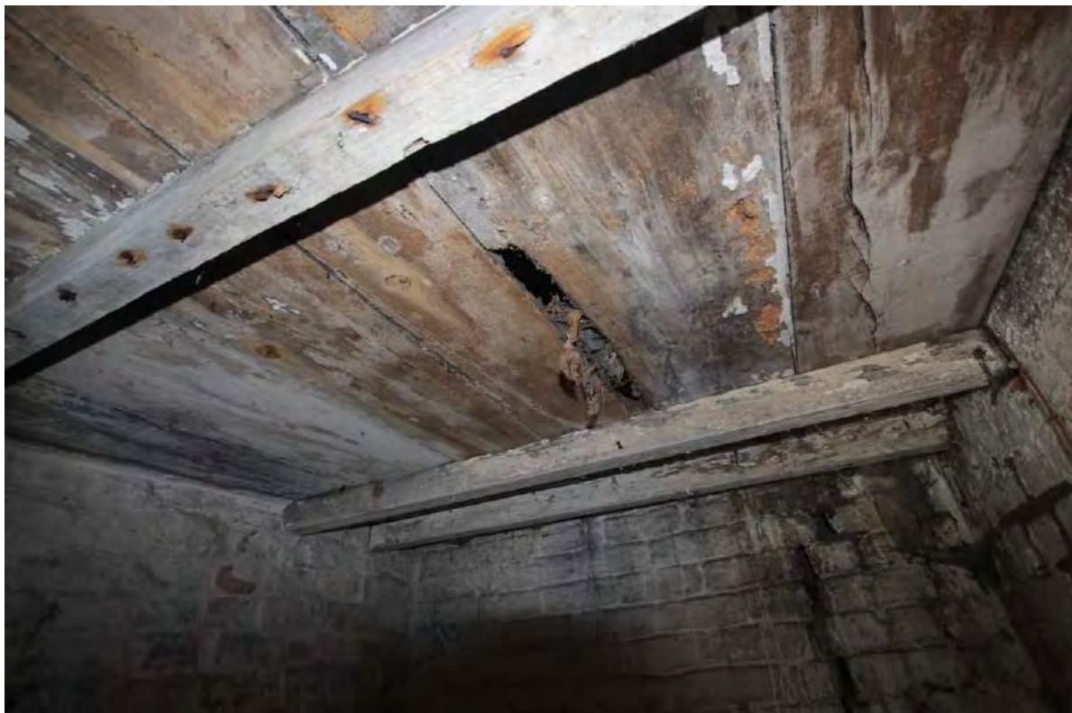
Photograph 84: View of the ceiling structure of Room 5, taken facing north-east (File: HBR_139)
