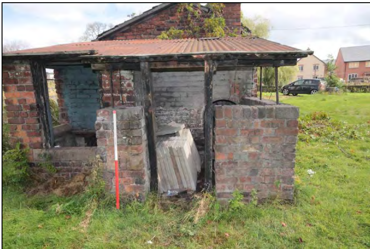
Photograph 37: View of the southern portion of the outbuilding's western elevation, taken with 1m scale facing east (File: HBR_50)
