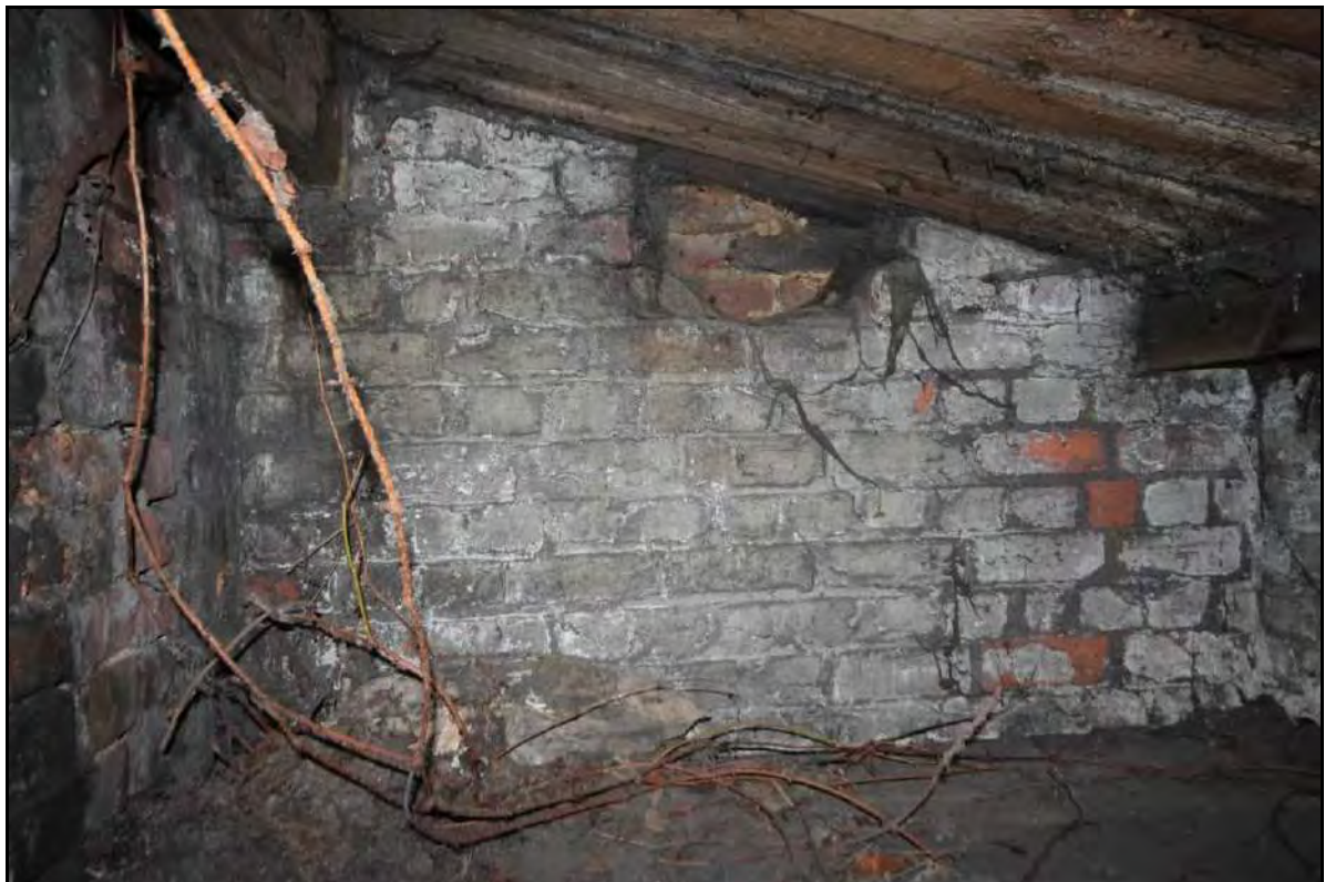
Photograph 93: View of the southern wall of Room 6, taken facing south (File: HBR_111)
