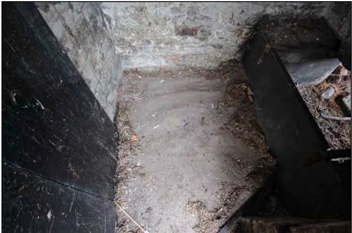
Photograph 62: View of the concrete flooring within Room 2, taken facing south (File: HBR_99)
