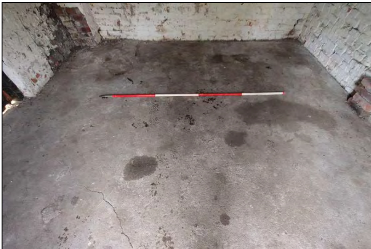
Photograph 52: View of the concrete flooring of Room 1, taken facing west with 2m scale (File: HBR_78)
