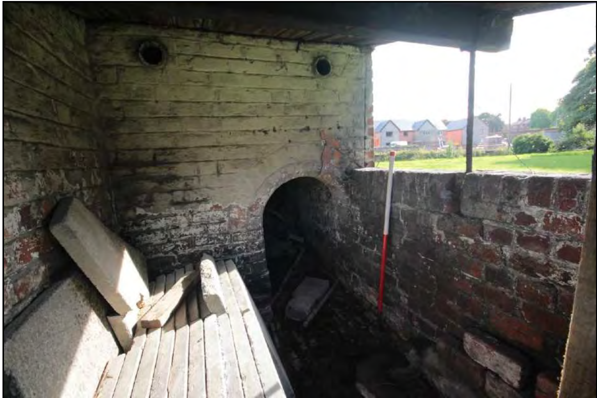
Photograph 74: General view to the south-east within Room 4, taken with 1m scale (File: HBR_121)
