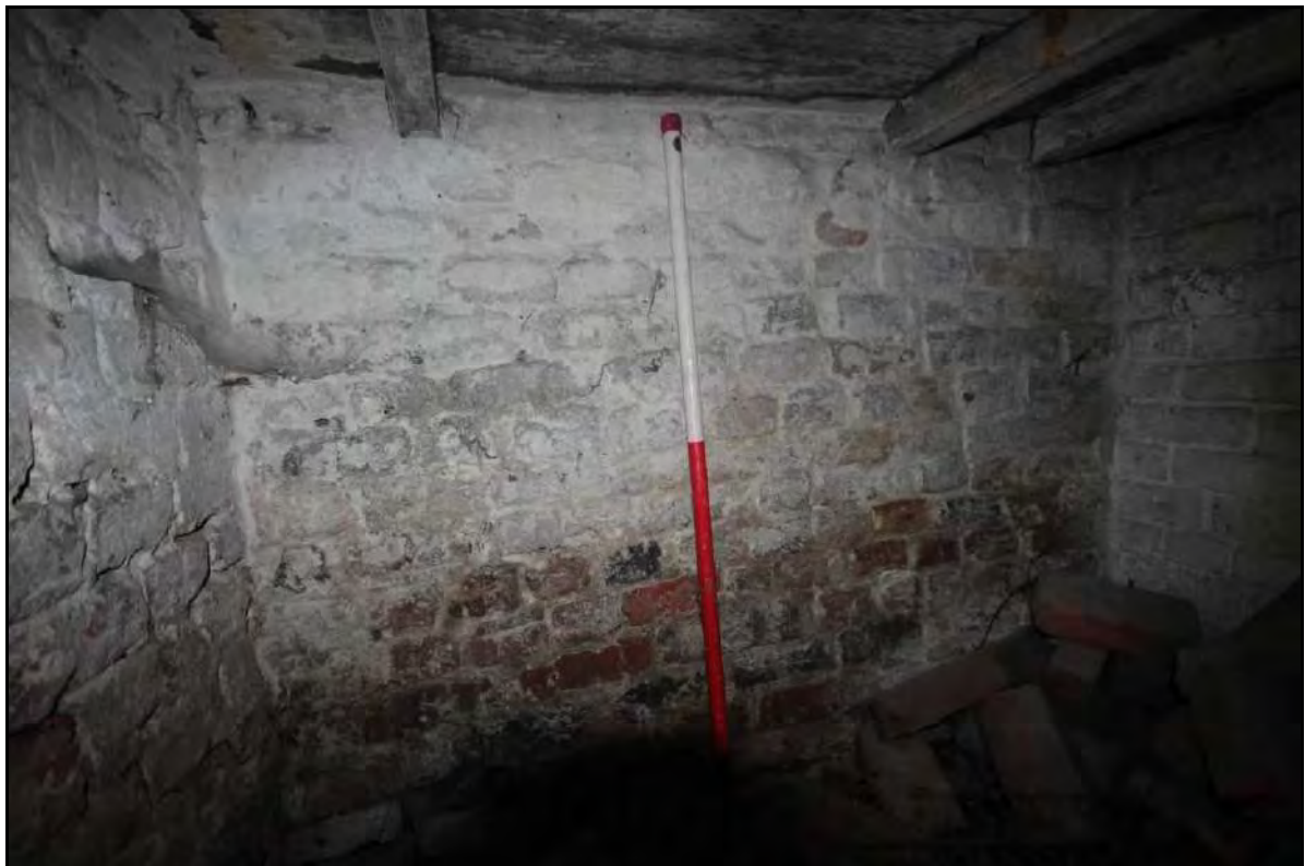
Photograph 86: View of the northern wall of Room 5, taken with 1m scale facing north (File: HBR_141)
