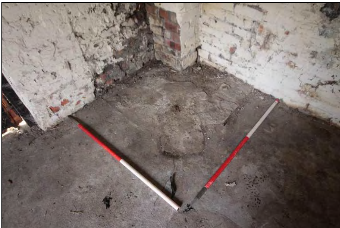
Photograph 53: View of the structural scarring where the wash copper stood within the south-western corner of Room 1's flooring, taken with 2 x 1m scale facing south-west (File: HBR_80)
