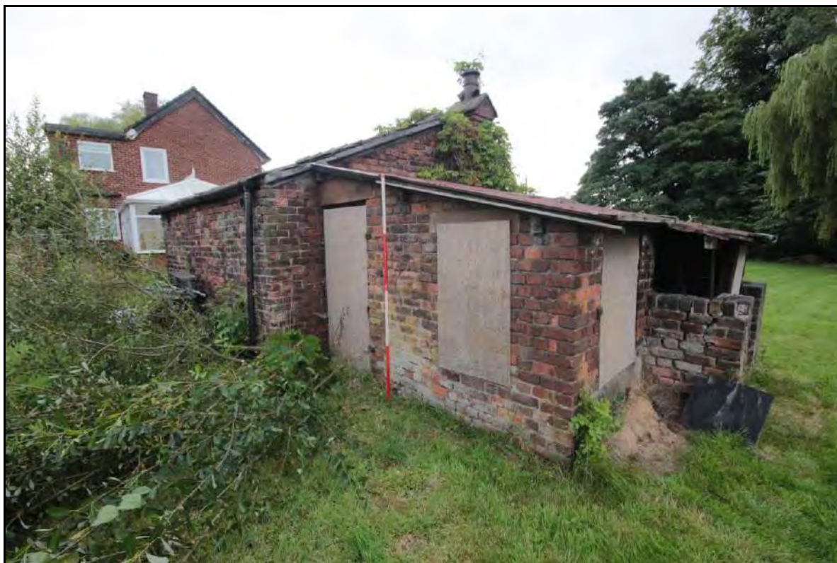
Photograph 39: Oblique view of the outbuilding's northern elevation, taken with 2m scale facing south-east (File: HBR_58)
