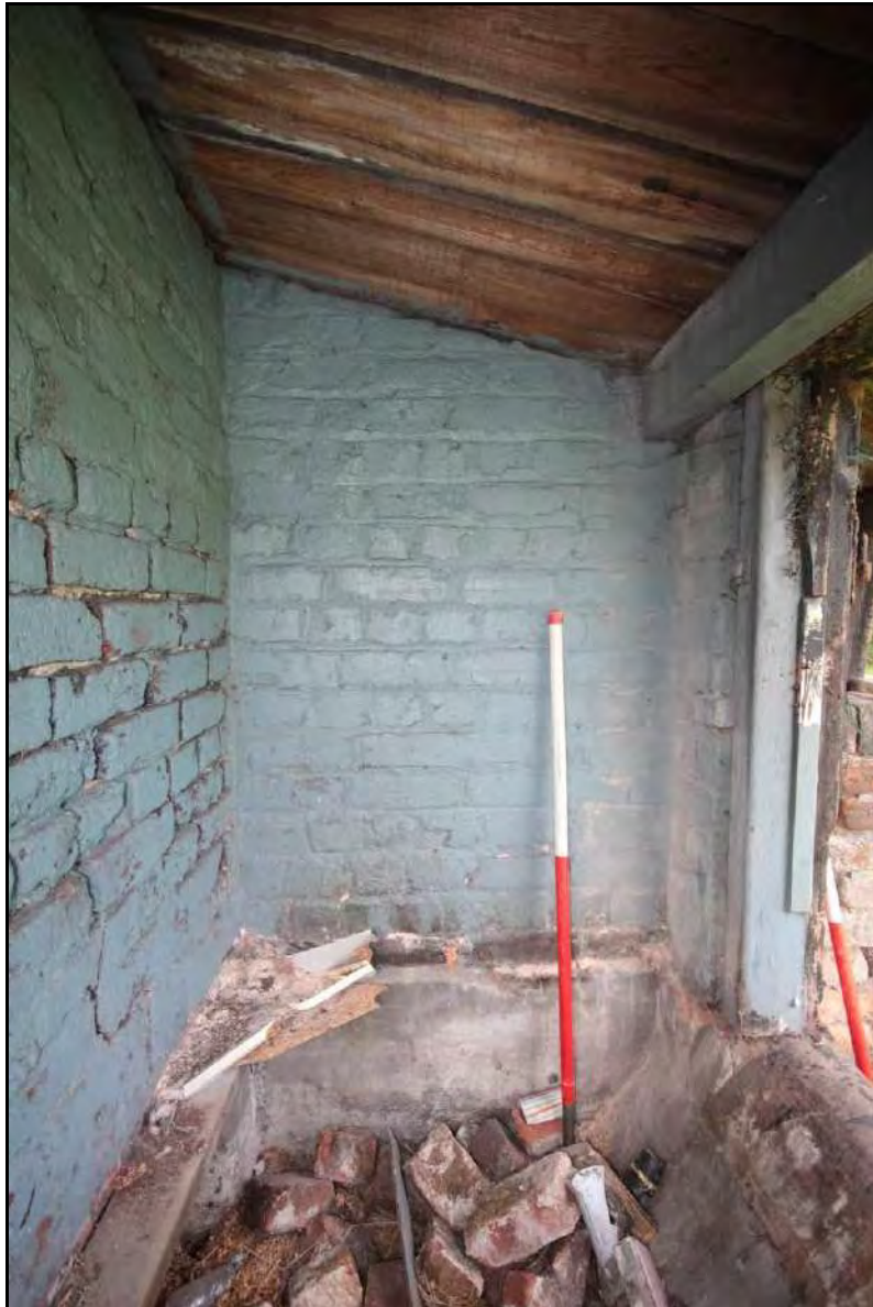
Photograph 73: View of the southern wall of Room 3, taken with 1m scale facing south (File: HBR_116)
