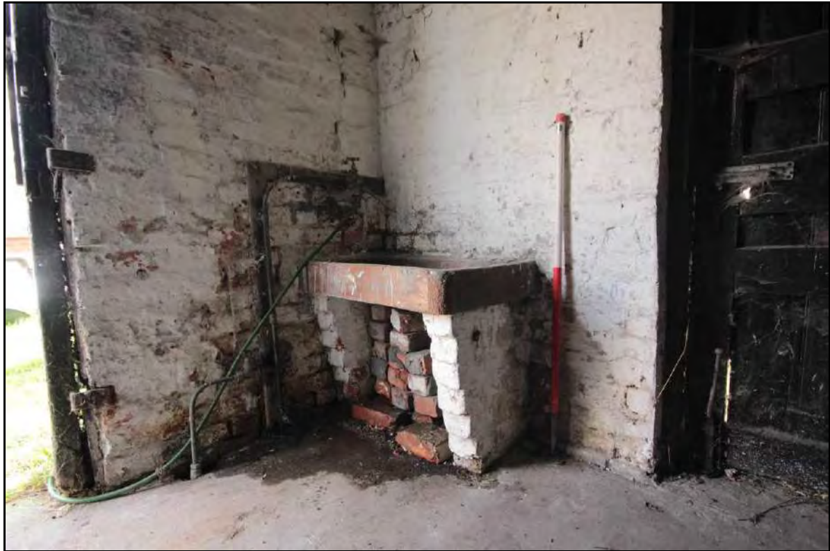
Photograph 58: View of the basin within the south-eastern corner of Room 1, taken facing south-east with 1m scale (File: HBR_89)
