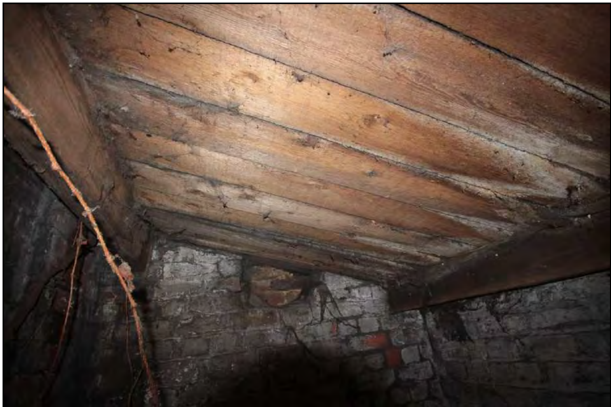
Photograph 91: View of the roof structure of Room 6, taken facing south (File: HBR_108)
