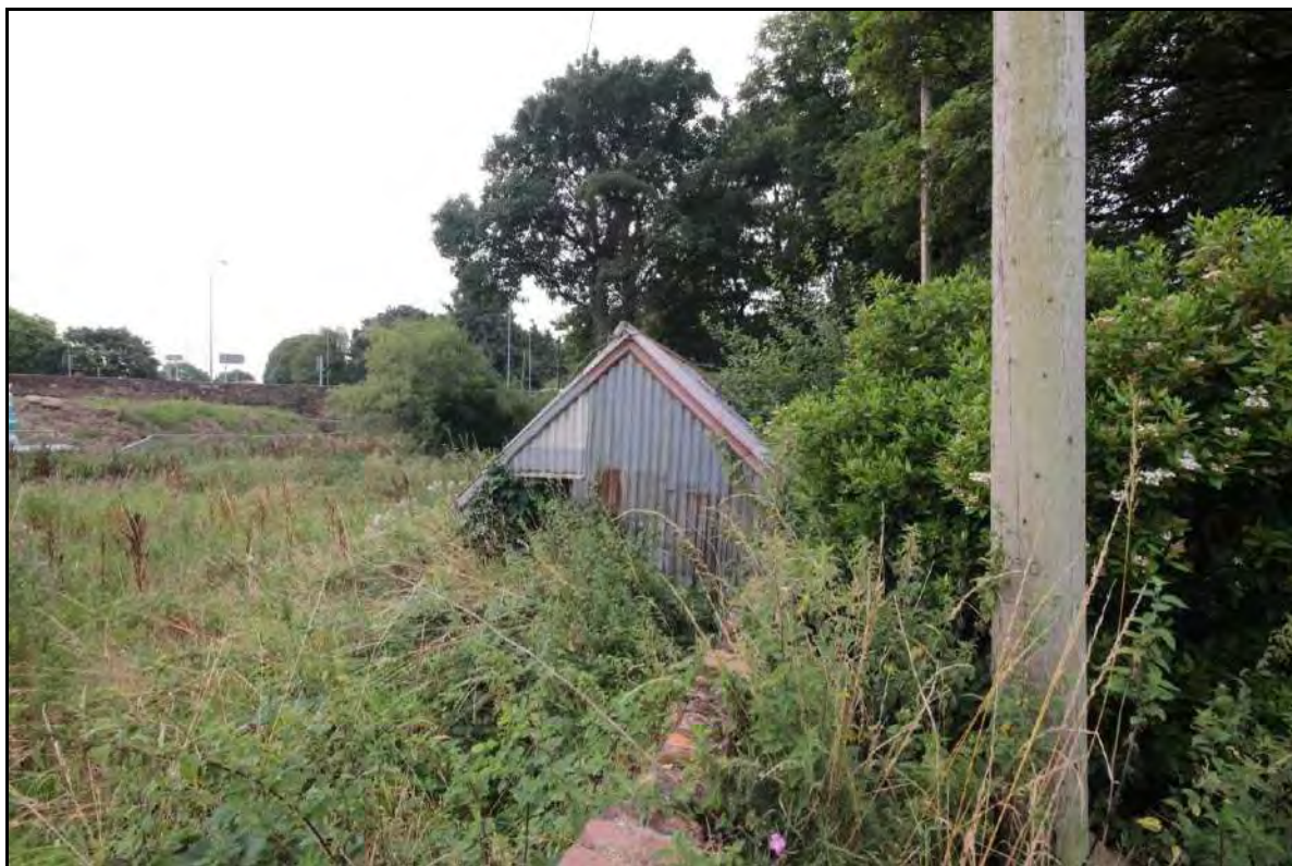
Photograph 10: View of the structure on the eastern side of the eastern boundary of the site, taken facing south-east (File: HBR_6)
