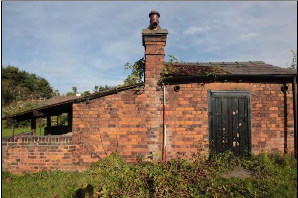
Photograph 33: View of the central extent of the outbuilding's southern elevation, taken facing north with 2m scale (File: HBR_42)
