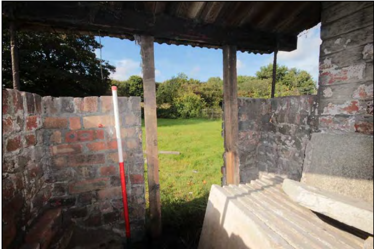
Photograph 78: View of the western wall of Room 4, taken facing west with 1m scale (File: HBR_130)
