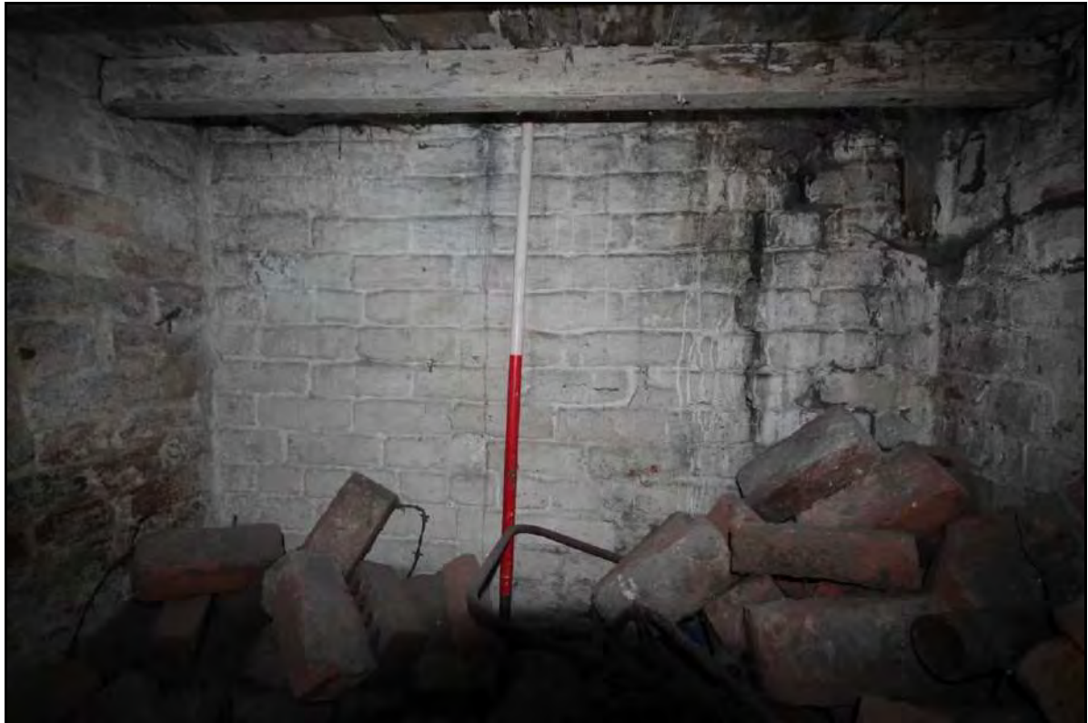
Photograph 85: View of the eastern wall of Room 5, taken with 1m scale facing east (File: HBR_141)
