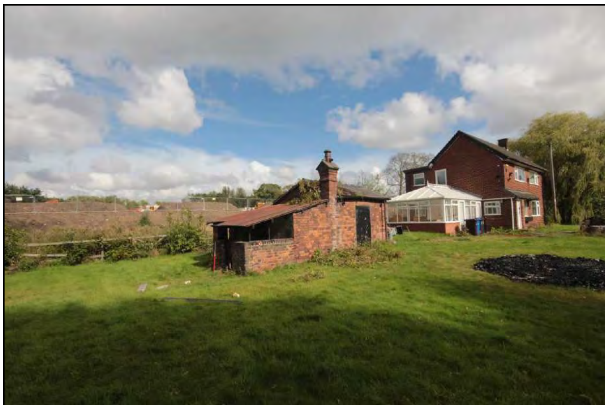
Photograph 24: View of the outbuilding from the south-west, taken with 1m scale facing north-east (File: HBR_49)
