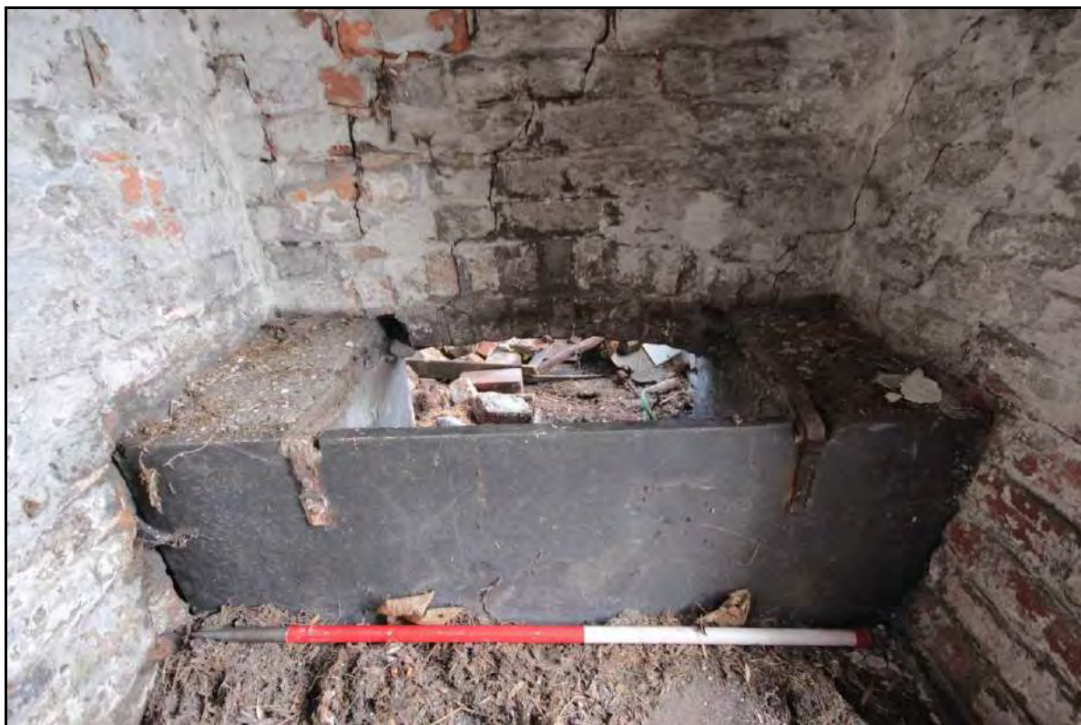
Photograph 64: View of the slate privy attached to the western wall of Room 2, taken with 1m scale facing west (File: HBR_101)
