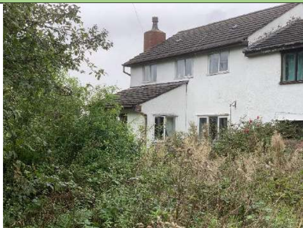
P4: The south of the farm house
