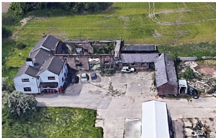
Figure 2. Aerial Image of Foxhill Farmhouse and Buildings G & I (Source: Google Earth).
