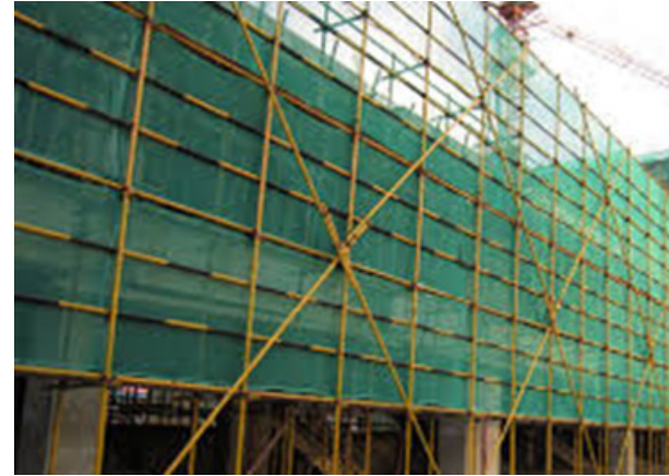
Figure 12. Debris netting
