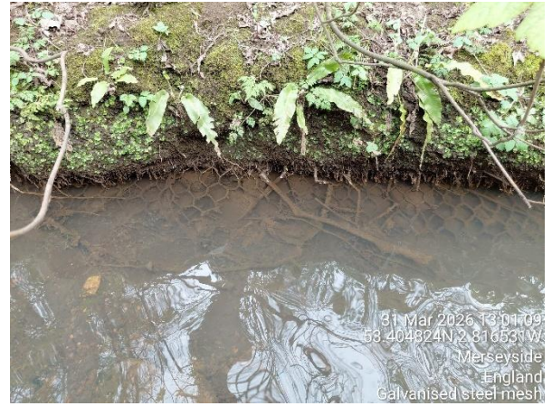
Photo 36: Galvanised steel mesh in water channel, attached to bank (SJ 45813 90089)
