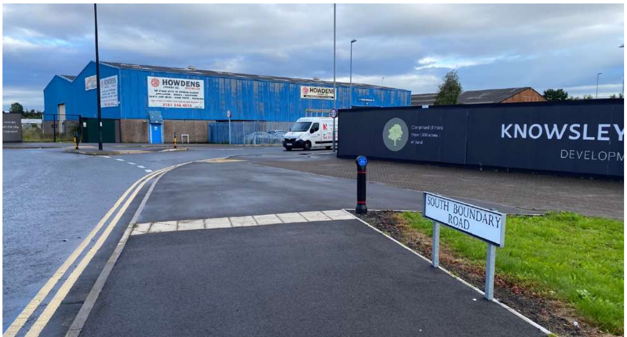
Photograph 5.1: Existing Footway Provision – South Boundary Road / Gale Road
