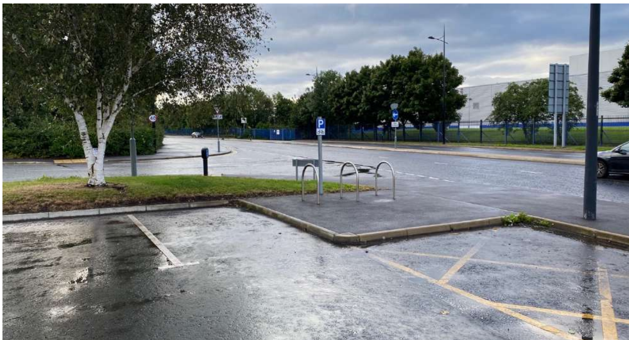
Photograph 3.4 : Admin Road / South Boundary Road
