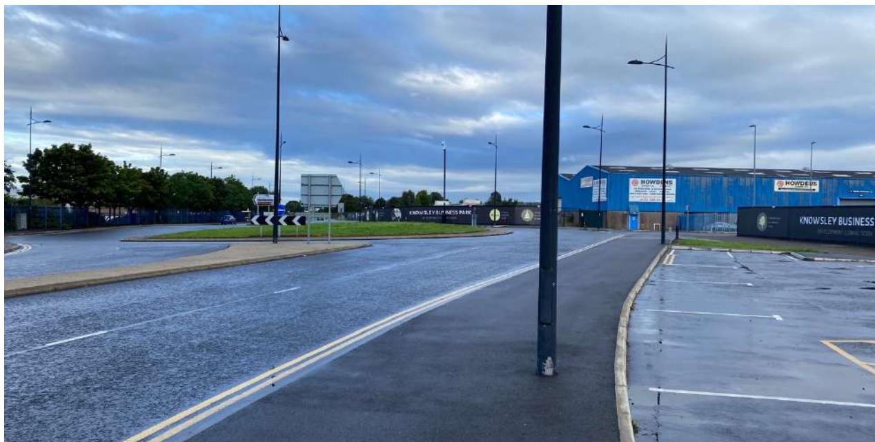
Photograph 5.2: Existing Footway Provision – South Boundary Road
