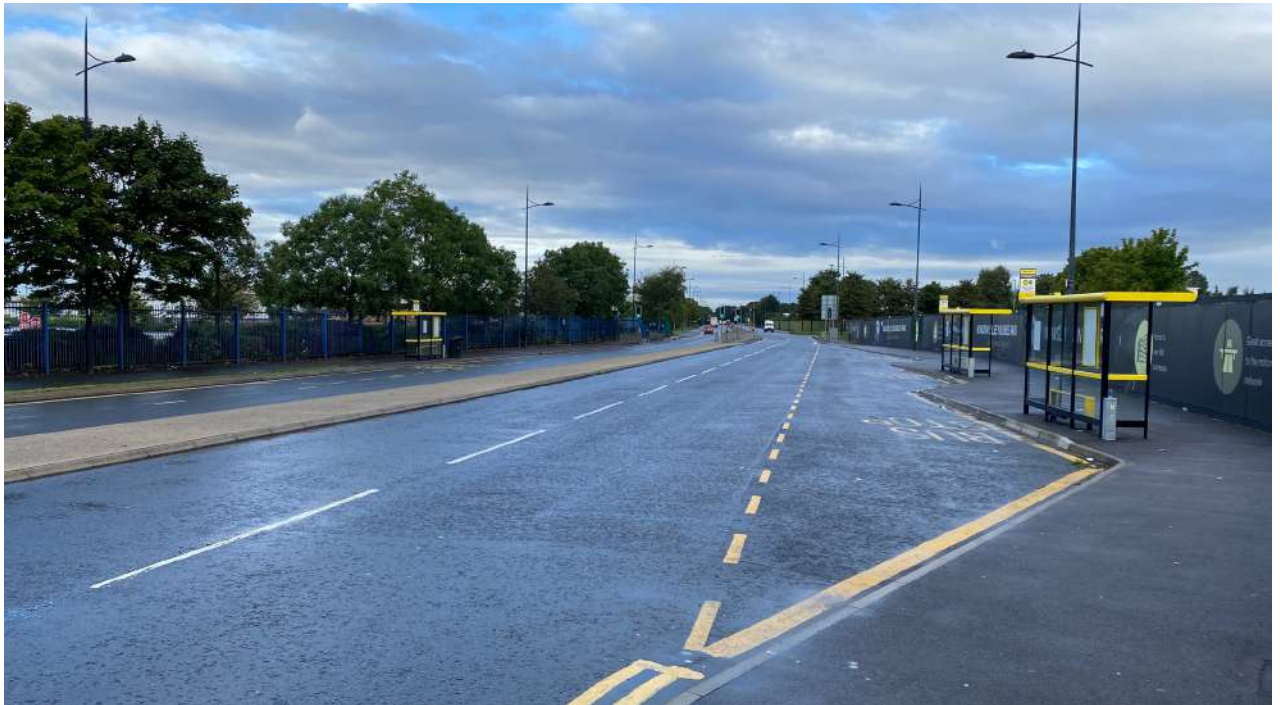
Photograph 2.1 : South Boundary Road – Westbound
