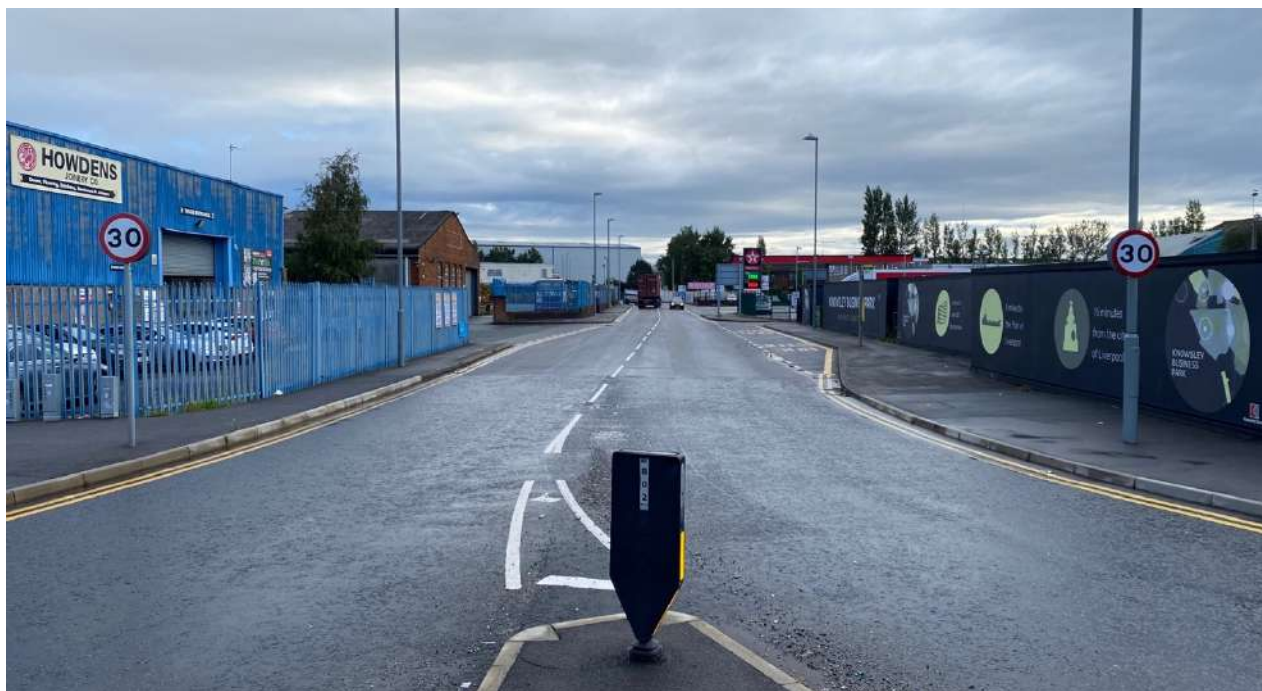
South Boundary Road (A5208) / Gale Road Roundabout
