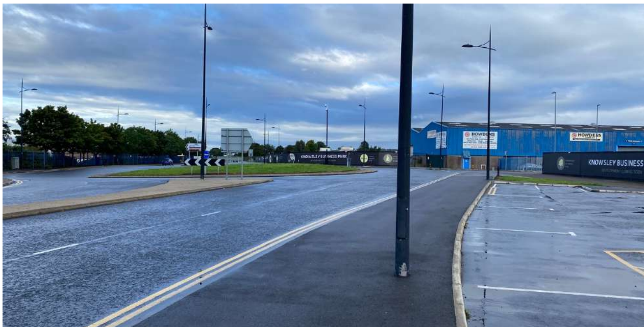
Photograph 5.2: Existing Footway Provision – South Boundary Road
