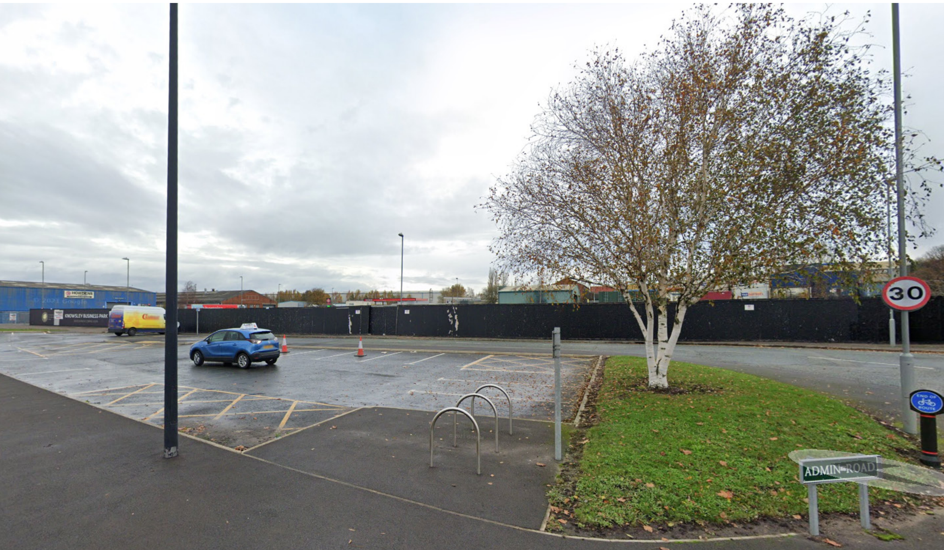
View of existing car park and site from South Boundary Road
