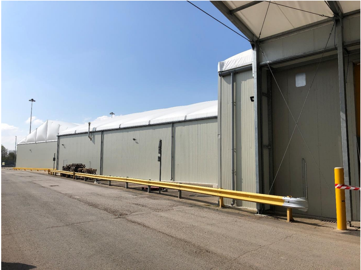
East Elevation of South Tent
