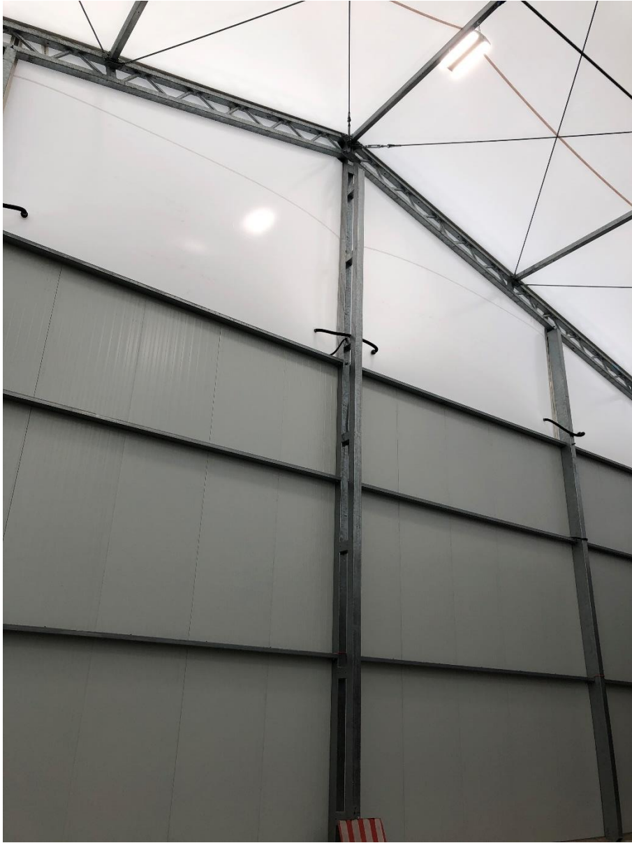
Ceiling structure of South Tent
