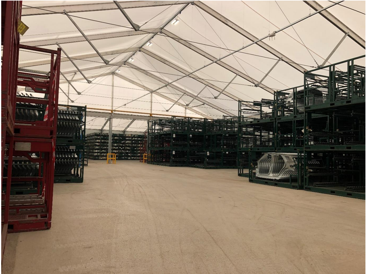
Racking inside South Tent
