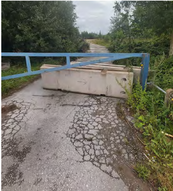
24. Proposed substation entrance looking east.
