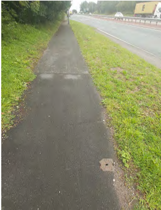
25. A580 pathway looking east from A5208 junction.
