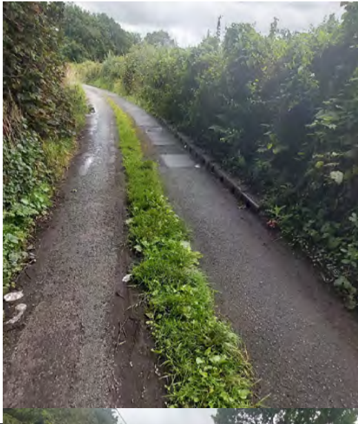
29. Hewitts Lane looking north, inbuilt drains along righthand side of road.
