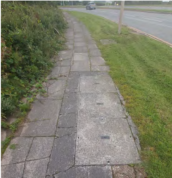
23. One of the various telecoms access grates indicating buried services under A5208 path.
