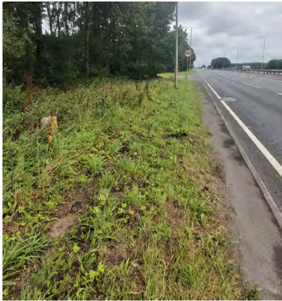
28. Hewitts Lane/A580 junction looking east, MP gas indicator to the left in the verge.
