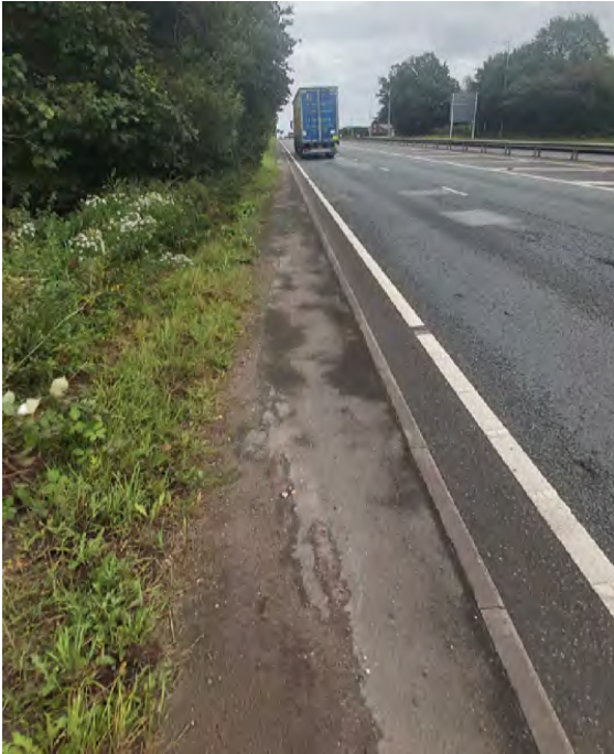
26. The A580 pathway narrows significantly to the east.
