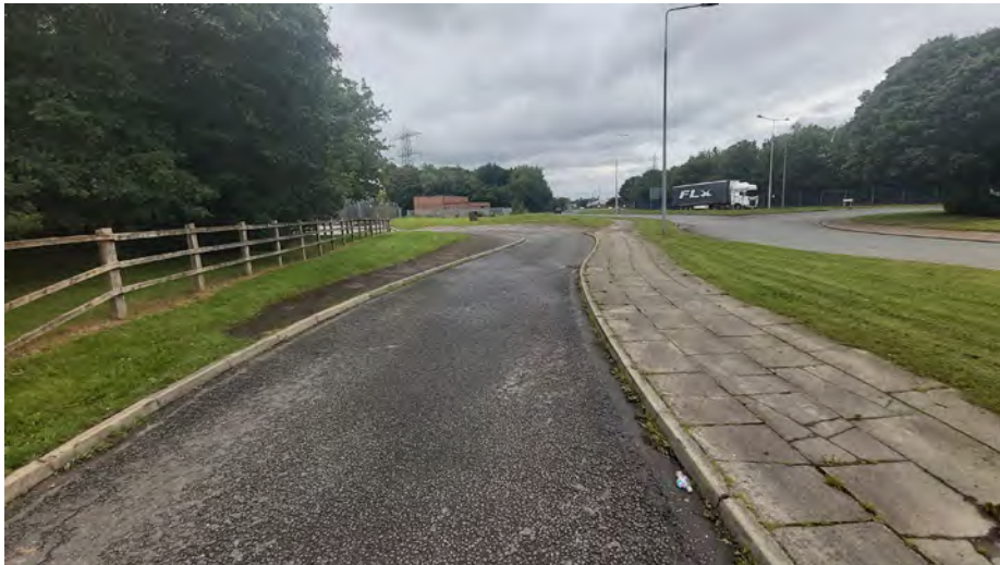
22. A5208 pathway looking north from Molly's Lane junction looking south.
