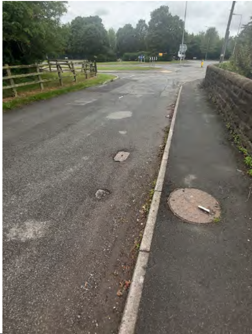
21. Molly's Lane/A5208 junction looking west.
