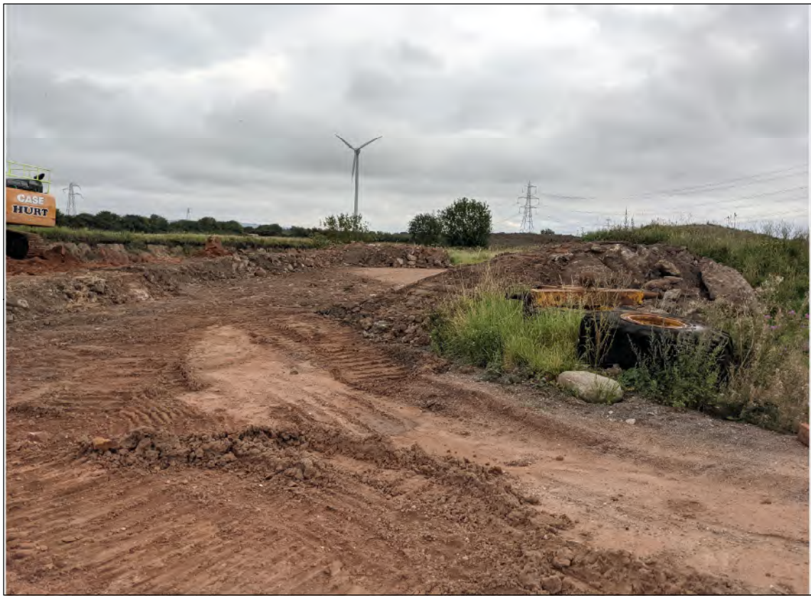
Plate 5) View towards eastern boundary of the Site, looking north-east
