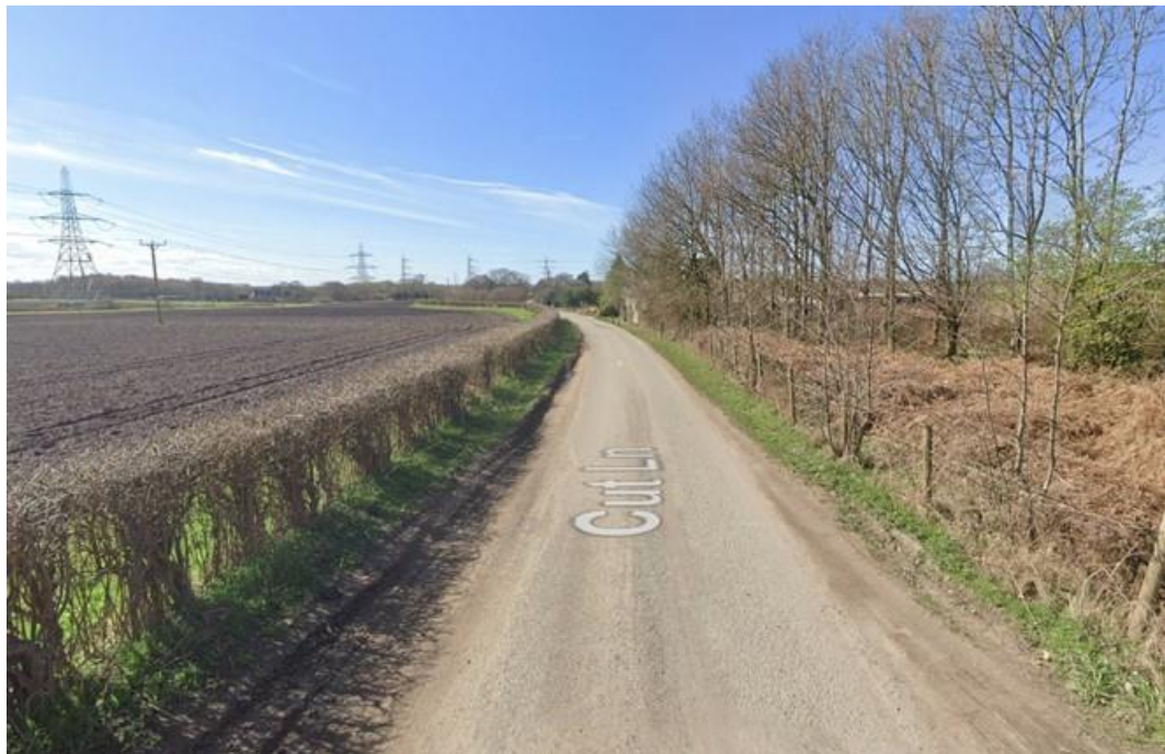
Figure 3. General Characteristics of Cut Lane
