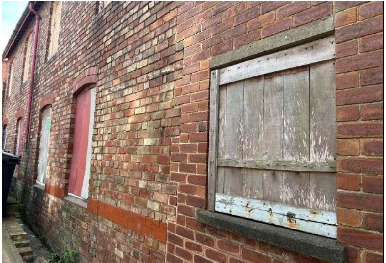
10. Brickwork reveals how the building was extended to form the entrance
