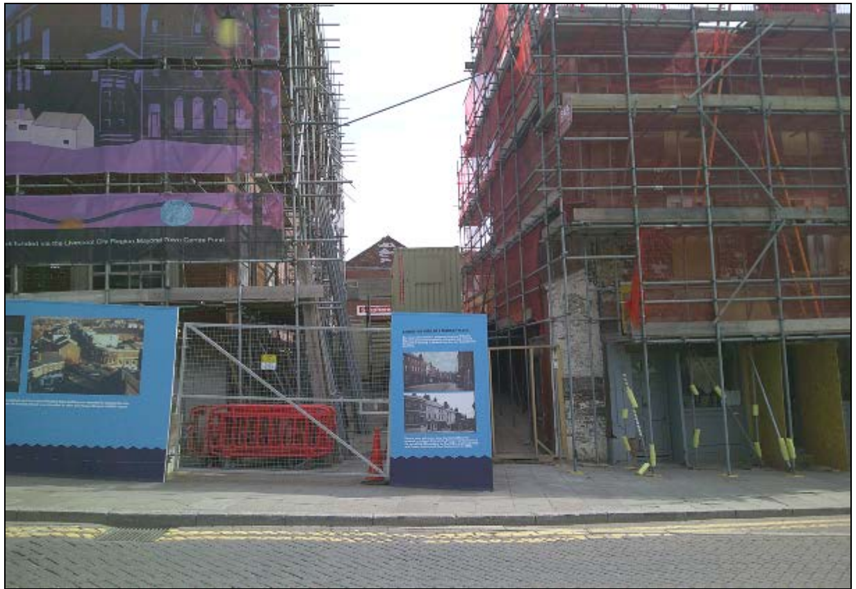
1. Glimpsed view of the buildings between numbers 2 and 7 Market Place
