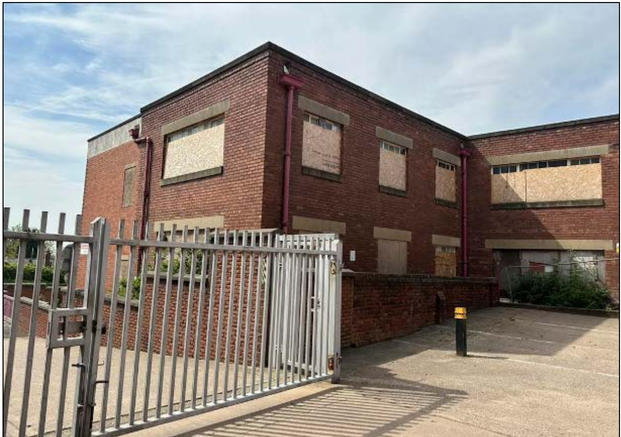
13. Three storey block at the south end of the site
