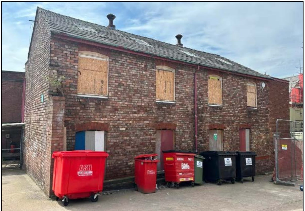
9. North elevation of the 1920s building
