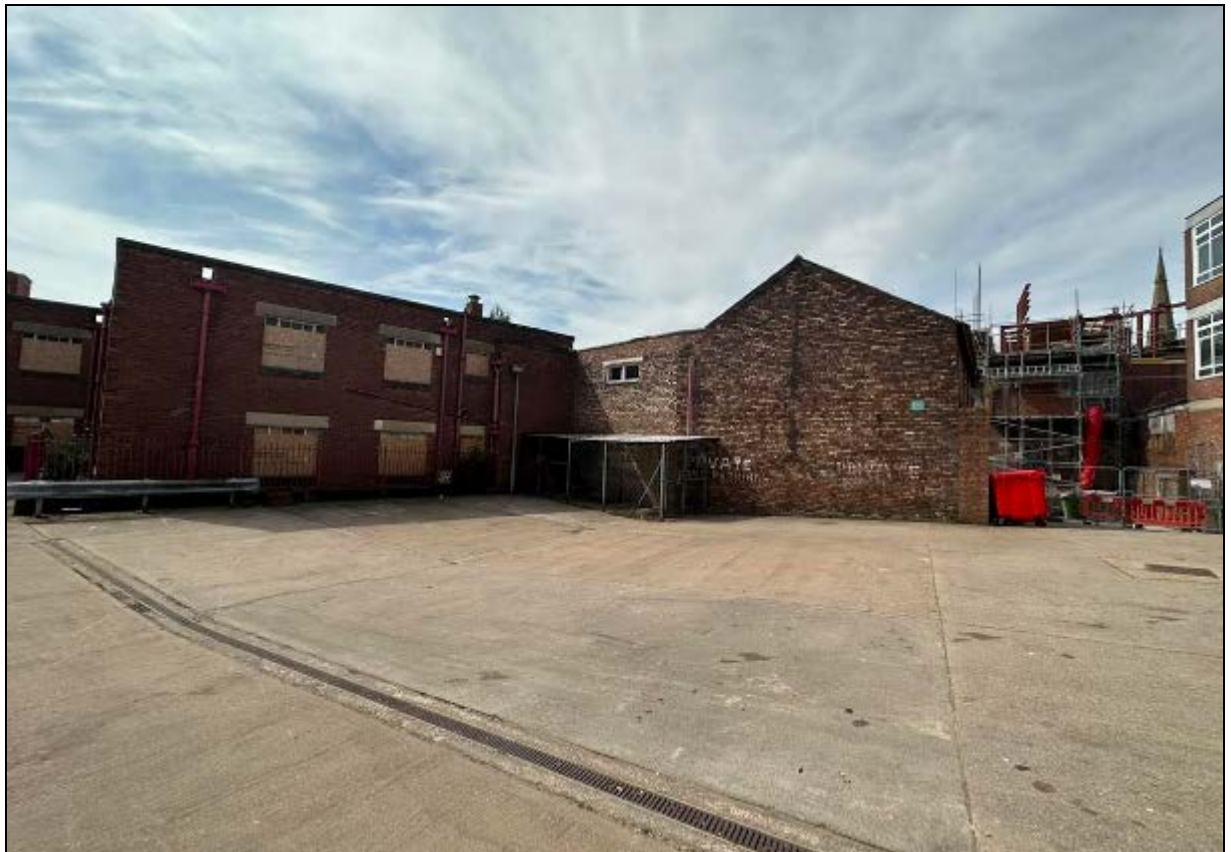
12. View west through the site, showing 1920s building (right) and 1950s elements attached
