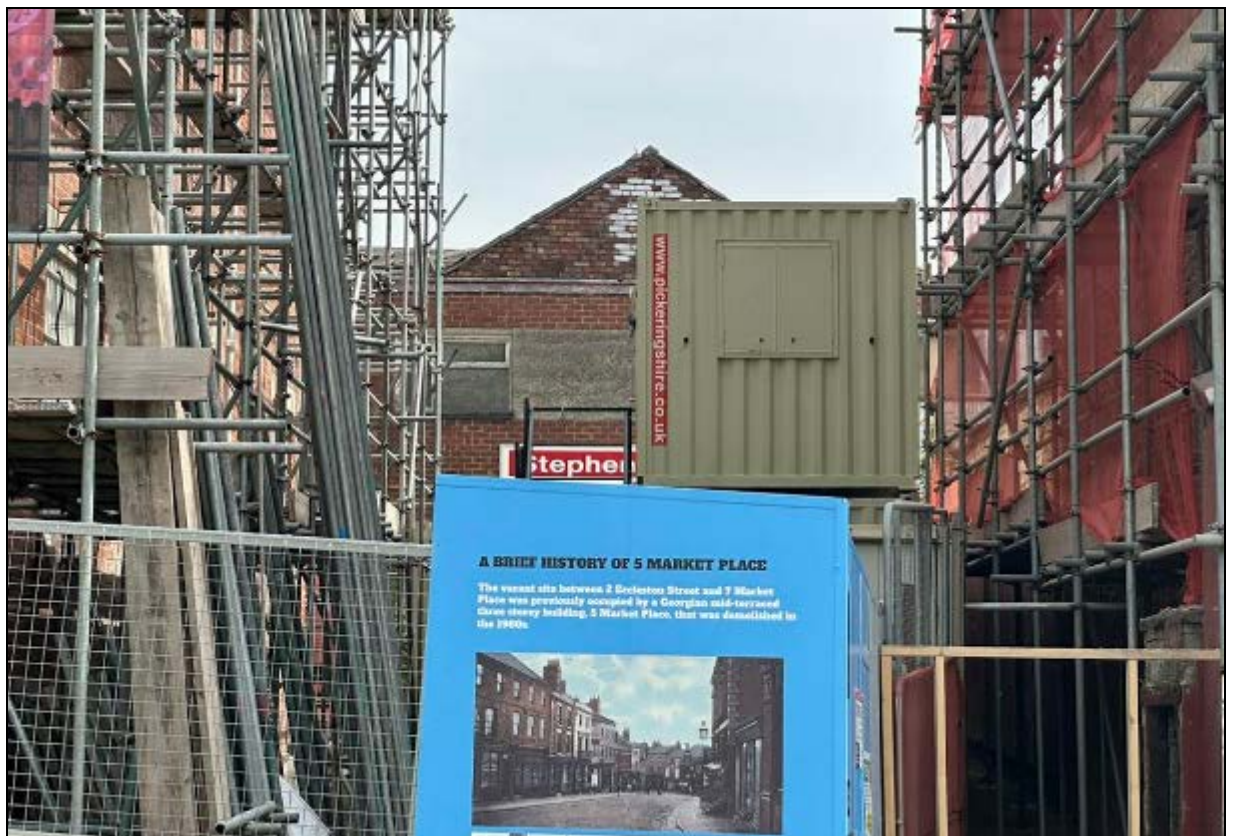
7. The building is now largely obscured from view by adjoining site works
