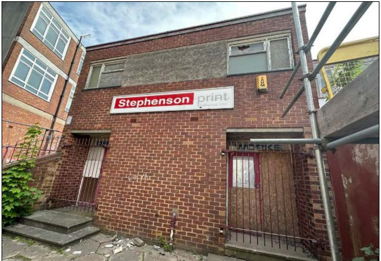
8. The entrance building, a 1950s extension of the 1920s structure behind
