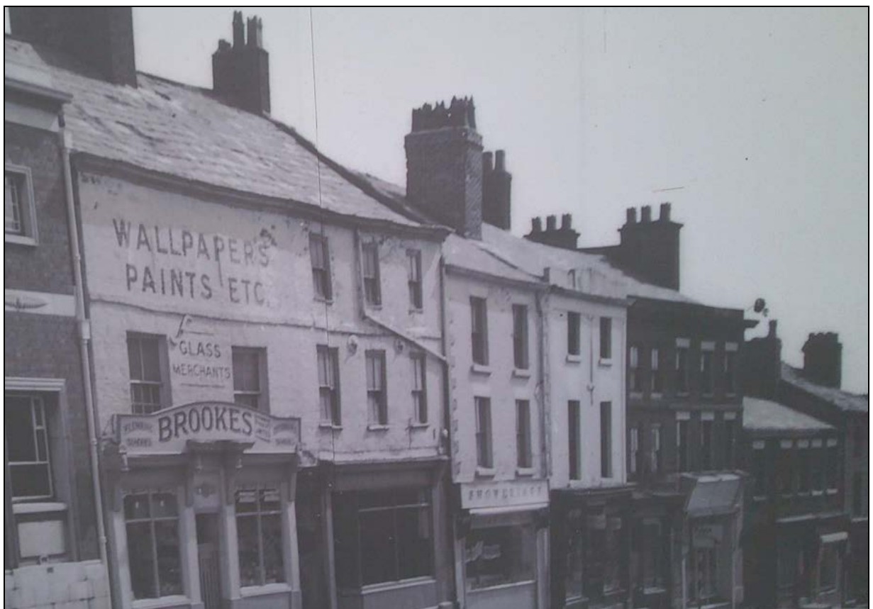
5. Mid-20 th century view of the Georgian row of which it forms part
