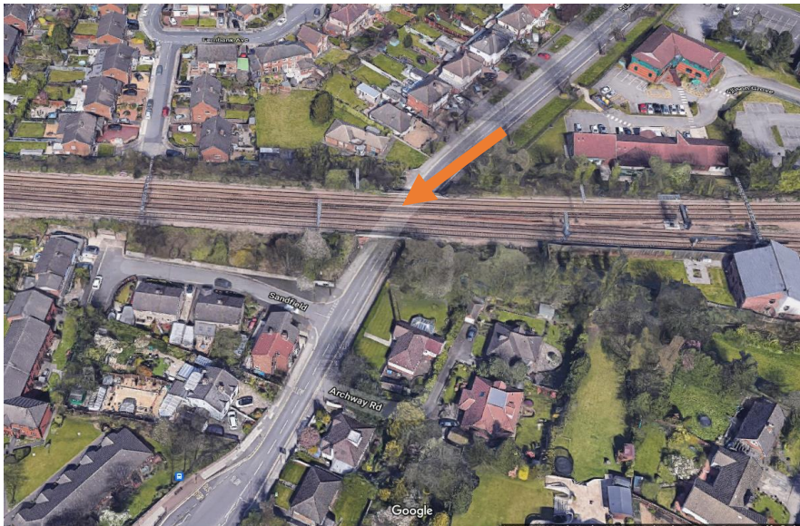
FIGURE 1 LOCATION OF THE GRADE II LISTED RAILWAY BRIDGE, ARCHWAY ROAD © GOOGLE MAPS
