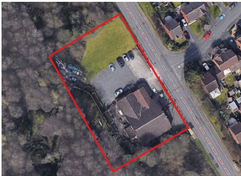
Figure 1 - Aerial Image of Site (Google Earth)
