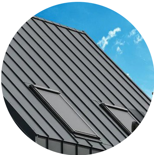
Standing seam Zinc roof in grey
