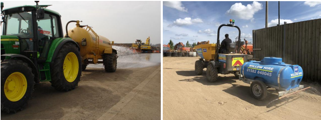
Dust control measures – dampening down techniques
