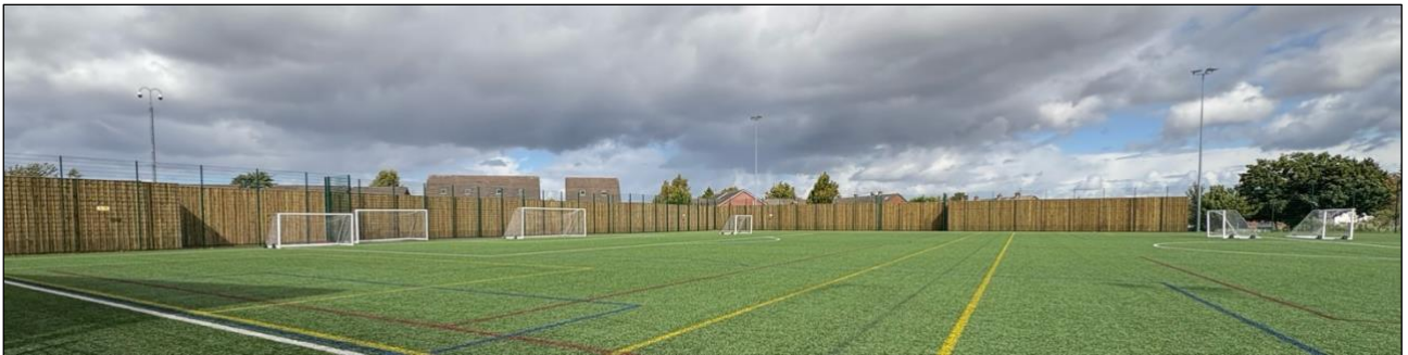
P2 : Photograph looking northwest from AGP hardstanding at newly constructed acoustic screen
