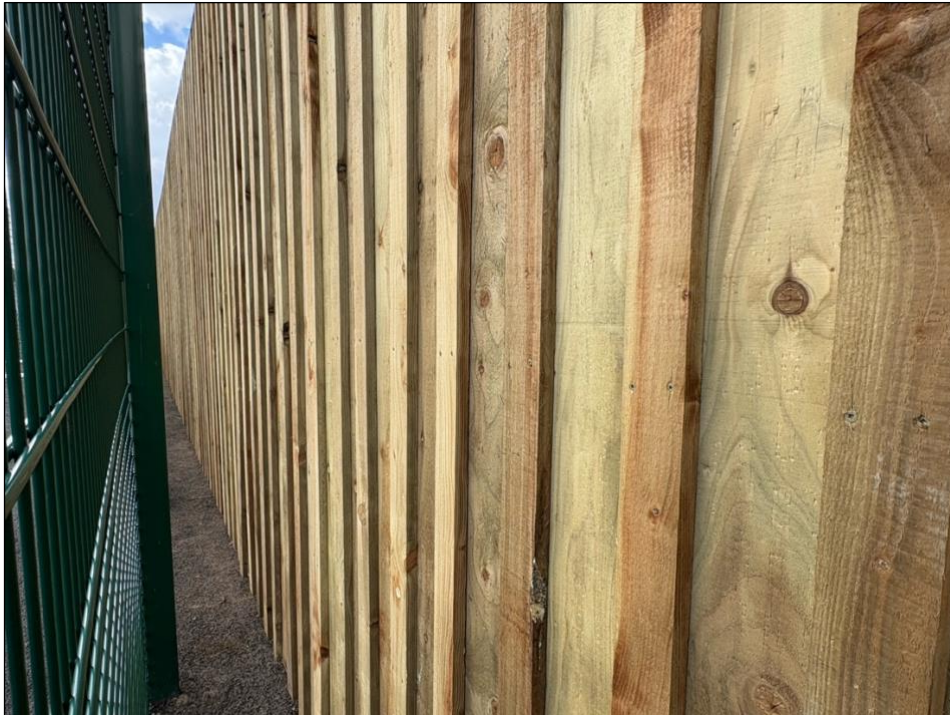
P3 : Photograph close-up of new acoustic screen (detailing no gaps, overlapping timber)
