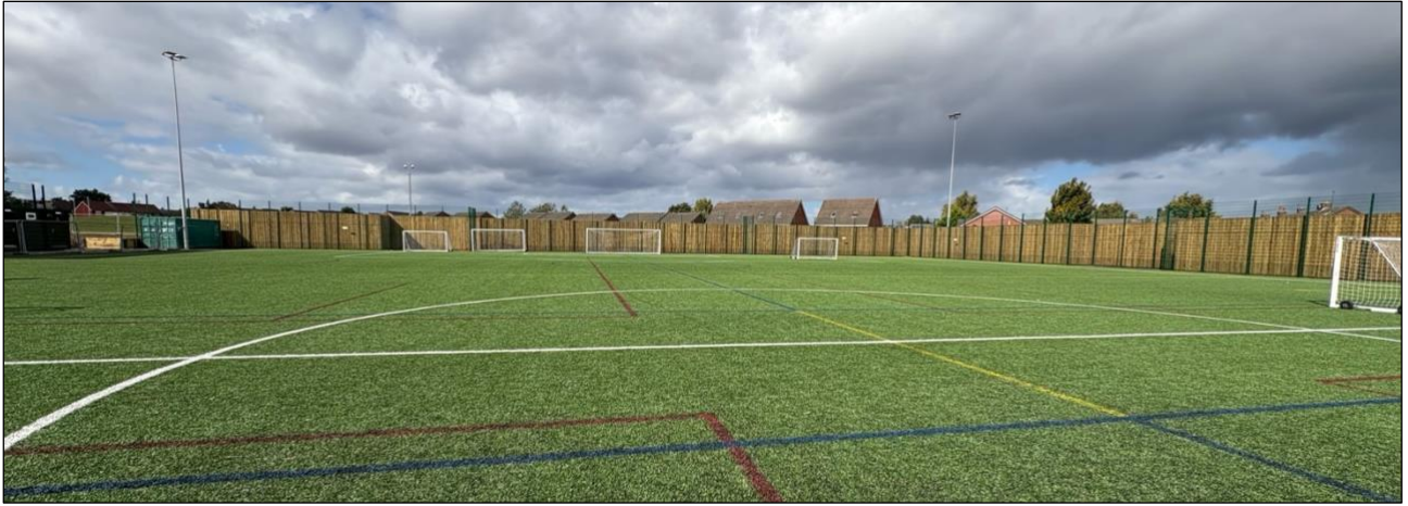
P1 : Photograph looking west from AGP at newly constructed acoustic screen
