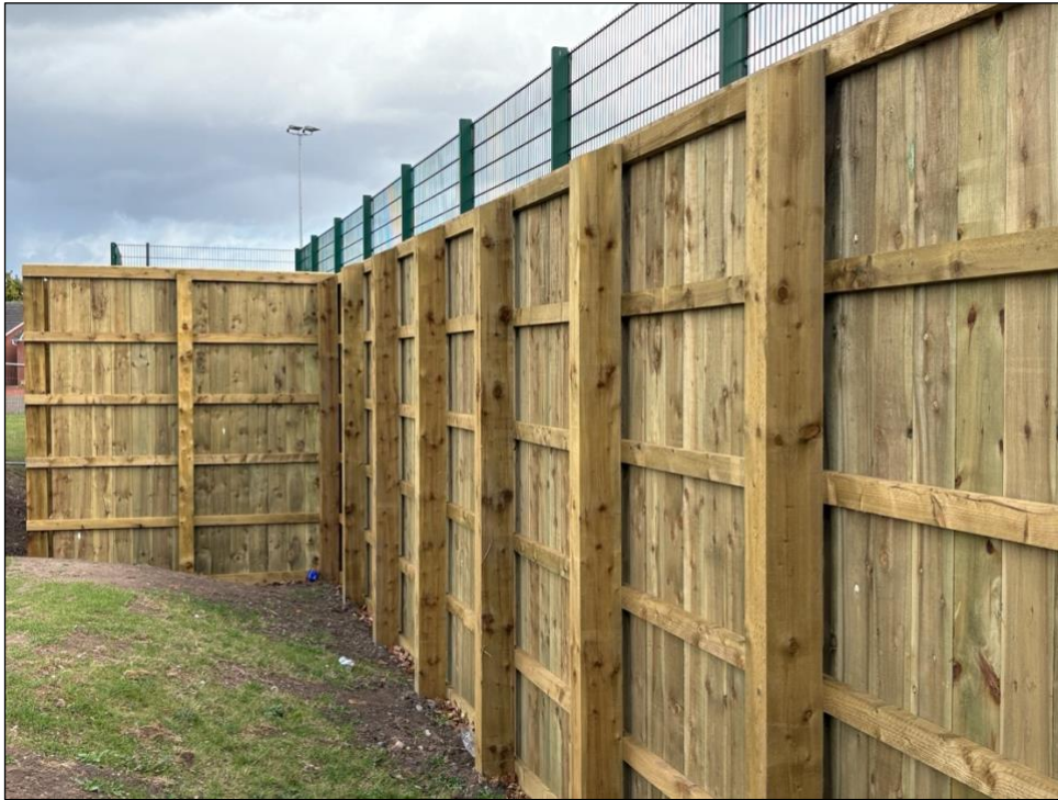
P4 : Photograph of rear of acoustic screen (detailing no gaps, overlapping timber)
