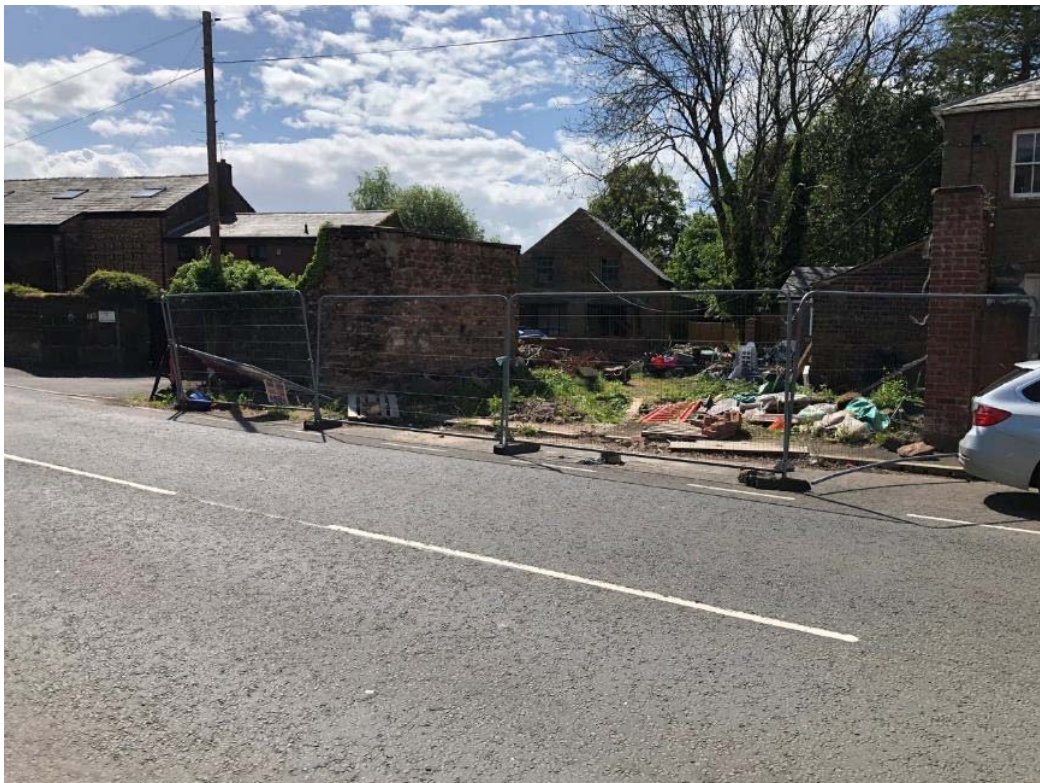
Plate 18. View facing south-east to Sandfield Cottage, The Purlins and End Barn adjacent Sandfield House. Note the missing section of Halsnead Park boundary wall
