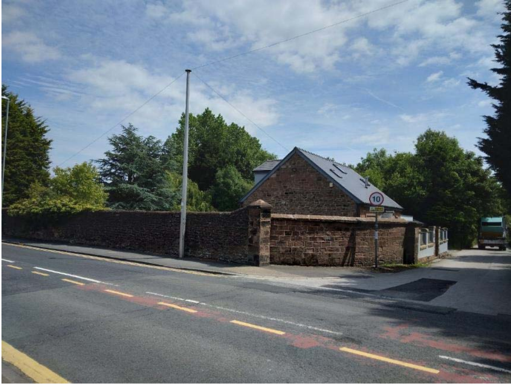
Plate 27. View facing east of Church Lodge and adjacent stone Piers and flanking walls (MME18747) at the junction of Windy Arbor Road and Main Drive
