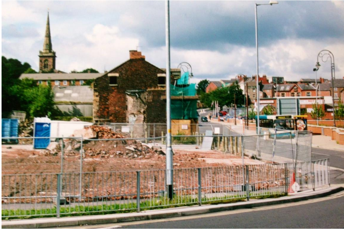
Figure 19: Sewell Street from the south, during demolition of buildings prior to construction of doctors' surgery; east side of Sewell Street shows garage in orange brick still standing (From Facebook page Born & Raised in Prescott, Photo by John Hopkins)
