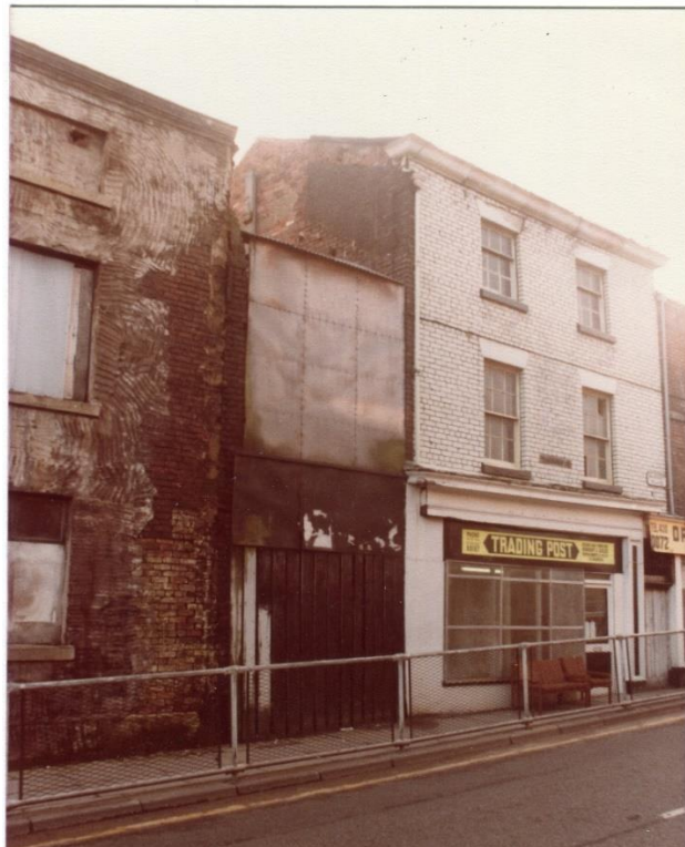
Figure 30: Kemble Street: Front of nos 6 (part visible to left, with blocked door), no 4 occupied by wooden hoarding, and no 2 (white front with Trading Post sign), all demolished; undated probably 1980s (courtesy of Owen Barton, Knowsley BC)
