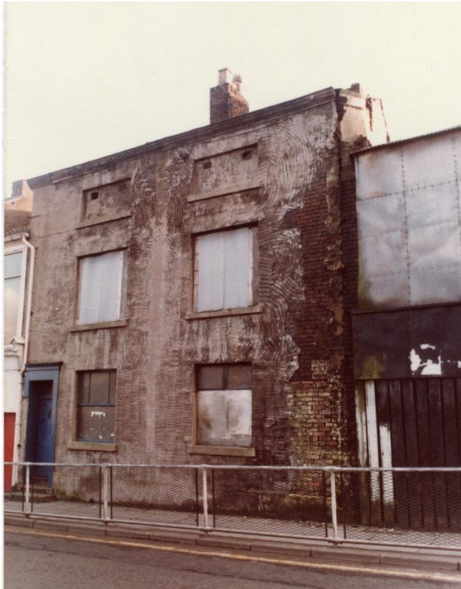
Figure 29: Nos 6 Kemble Street (with blue door) and No 4 occupied by wooden hoardings, both now demolished, 1980s (photograph courtesy of Owen Barton, Knowsley Borough Council)
