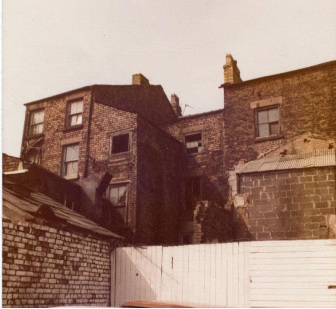
Figure 31: Rear of nos 48-50 Market Place to left and nos 2-4 Kemble Street, undated probably 1980s (courtesy of Owen Barton, Knowsley BC)
