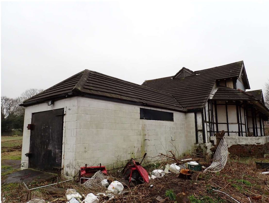
Photograph 4 – The northwestern aspect of Building 1.
