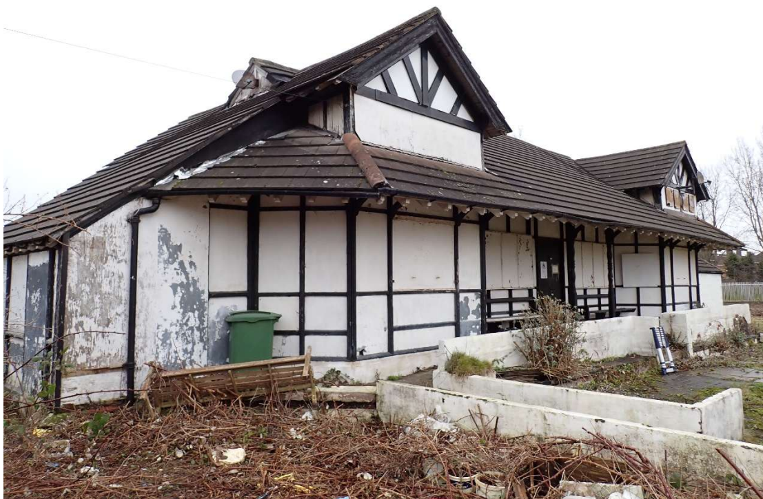
Photograph 1 – The southeastern aspect of Building 1.
