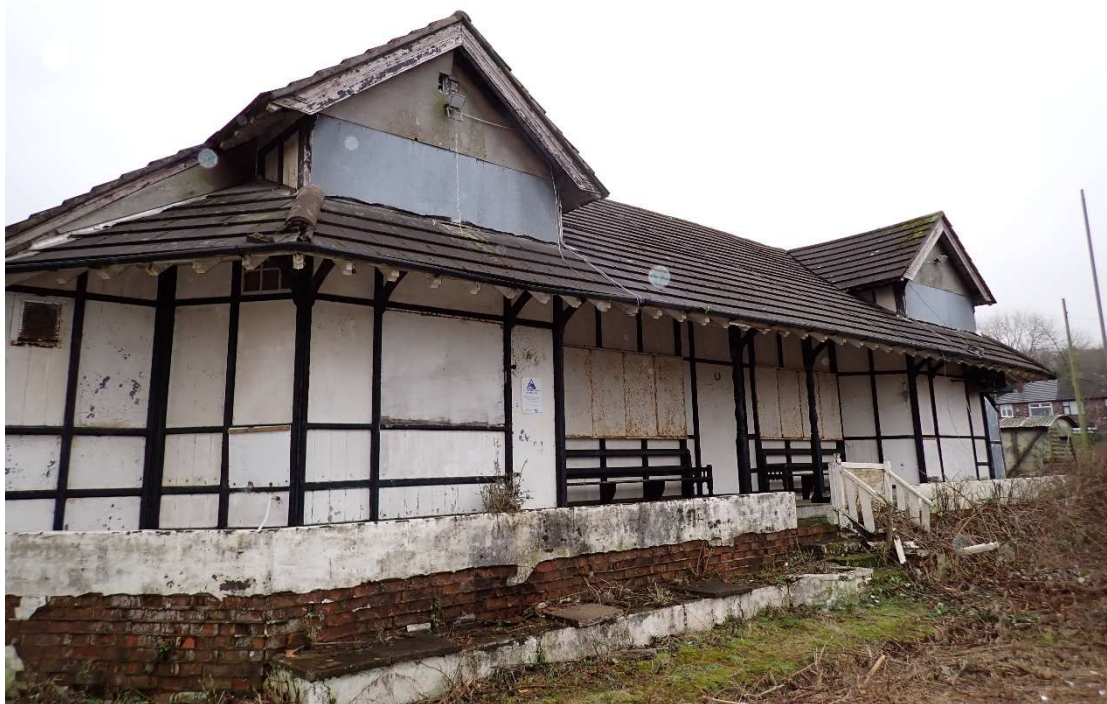
Photograph 2 – The western aspect of Building 1.
