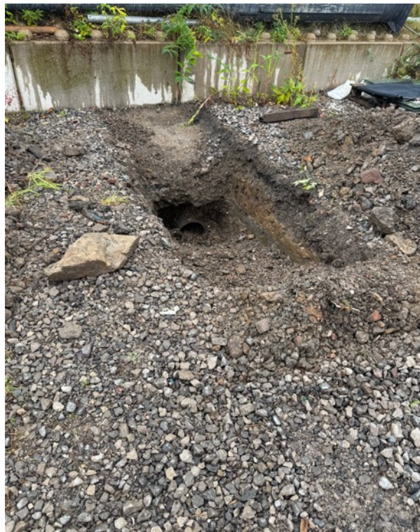
Photo 4: Exposed surface water pipe stub into site.
