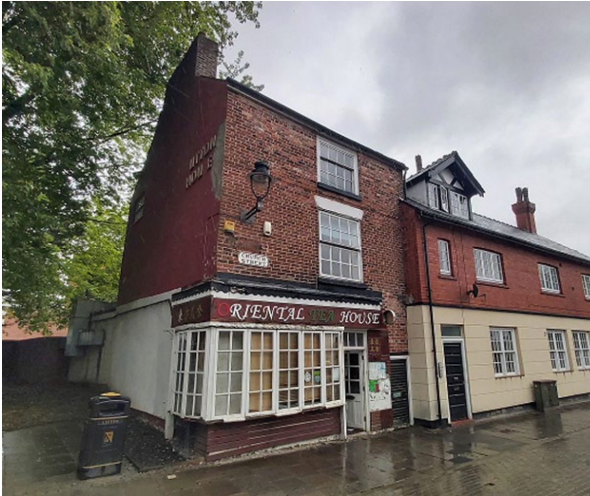
A view of the frontage of No.12 Church Street, Prescott.
