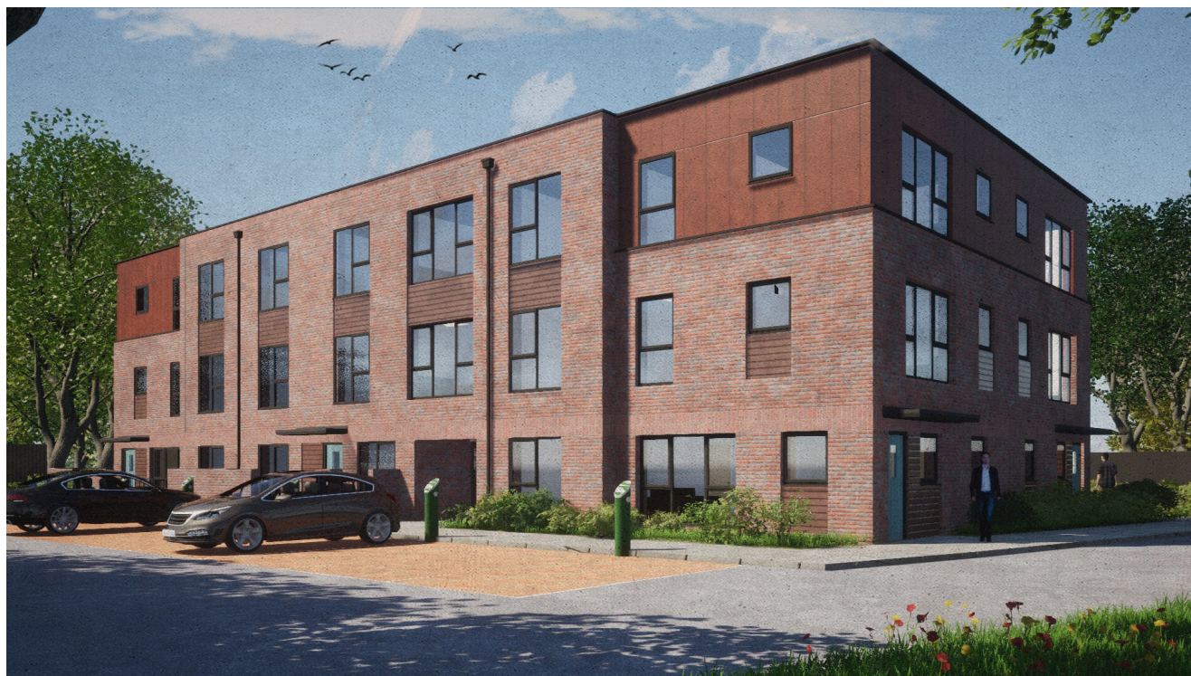
Fig.17 View of the car park where the bin & cycle store is accessed, hidden towards the back
