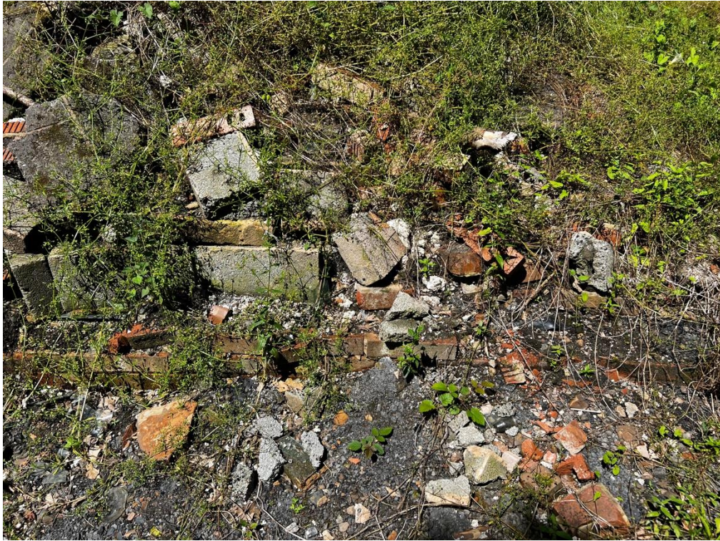
Pic 3; rubble of the previous demolished building
