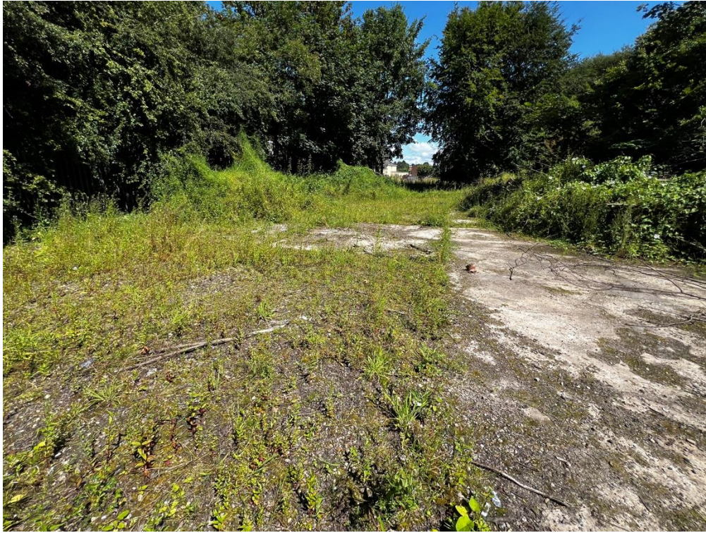
Pic 1; Looking North across the site
