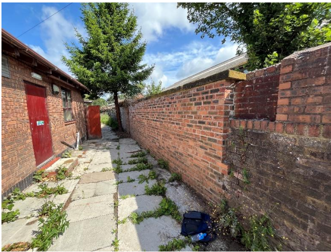
Rebuilt section adjacent Section 1. Junction of original and rebuilt.
