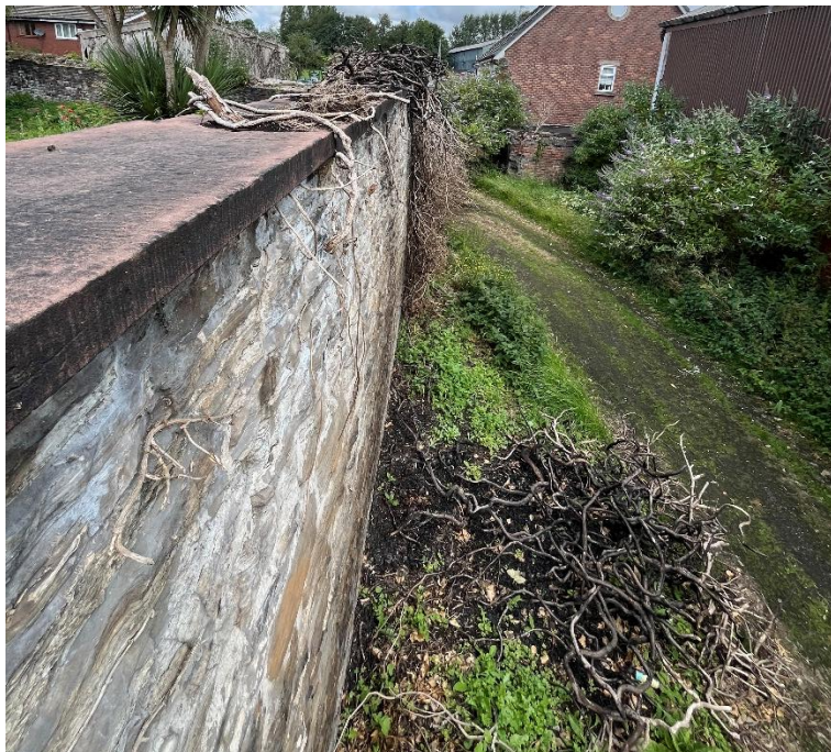
Rebuilt section adjacent Section 1. Junction of original and rebuilt.
