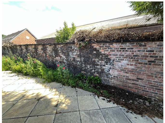
Rebuilt section adjacent Section 1. Junction of original and rebuilt.
