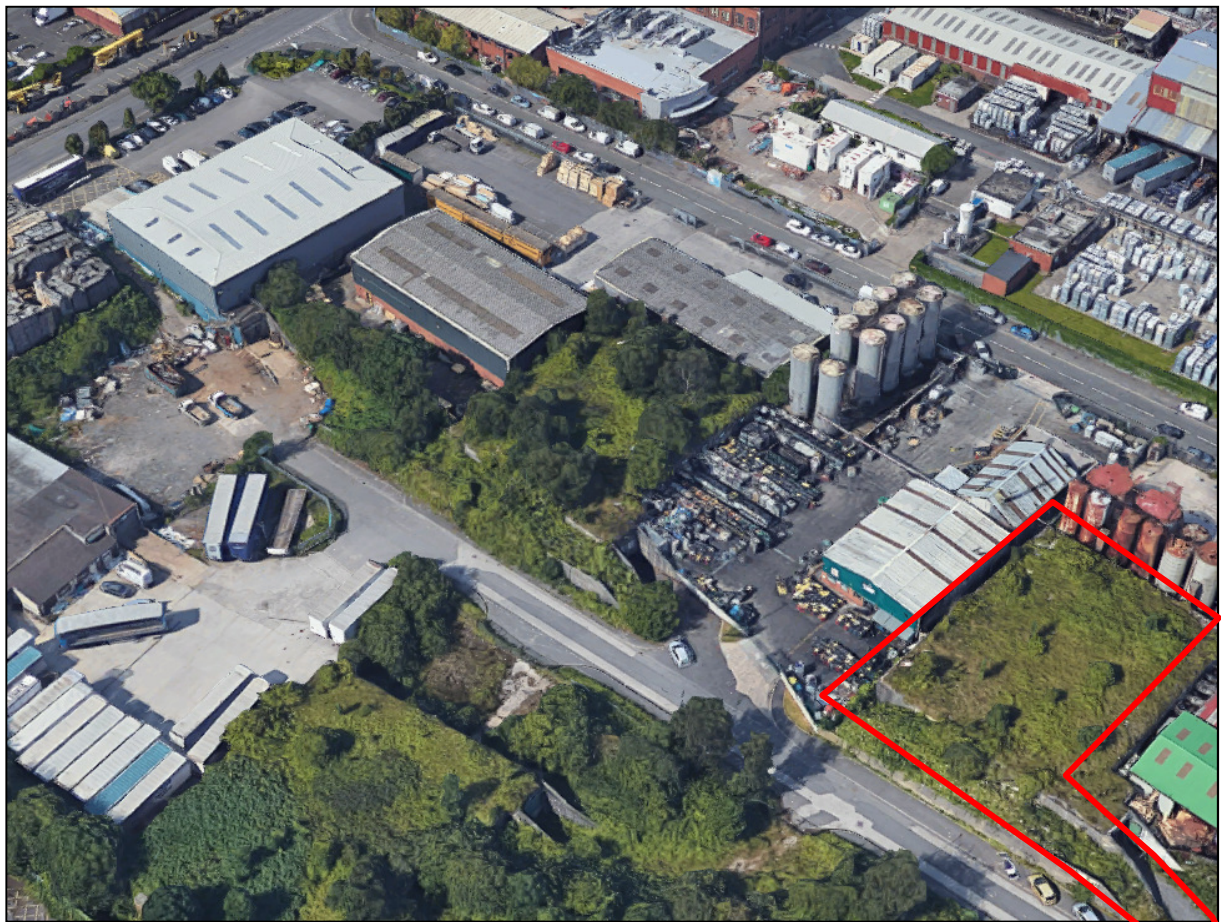
Site Position on Draw Well Road, highlighted in Red
