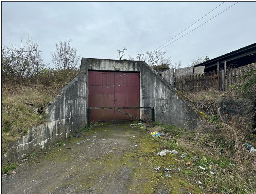
Figure 5 - Magazine 9-8 Entrance door.
