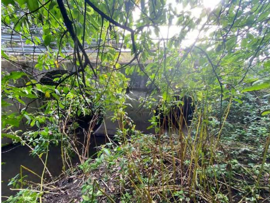
Photograph 5: Greensbridge Lane Structure IMG_2752.JPEG. Photo looking downstream
