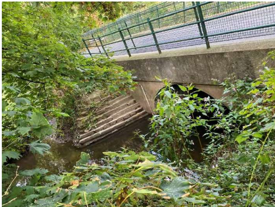
Photograph 2: Cartbridge Lane Structure IMG_2772.JPEG. Photo looking upstream
