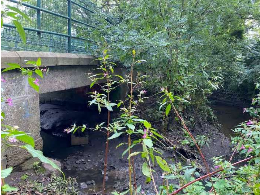
Photograph 3: Cartbridge Lane Structure IMG_2776.JPEG. Photo looking upstream
