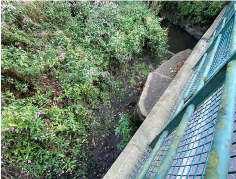
Photograph 1: Cartbridge Lane Structure IMG_2784.JPEG. Photo looking upstream shows that there is an overflow channel (dry) located higher than the main channel (water present). This is reflected in the modelled survey data.
