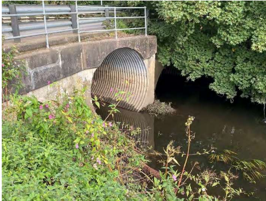
Photograph 7: Greensbridge Lane Structure IMG_2764.JPEG. Photo looking upstream
