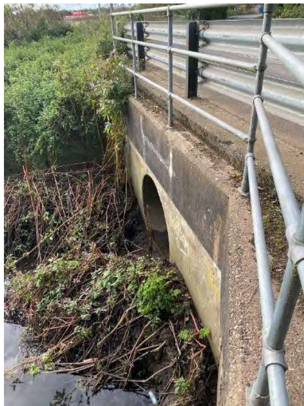
Photograph 8: Greensbridge Lane Structure IMG_2769.JPEG. Photo looking upstream
