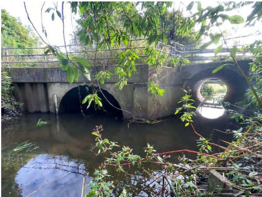
Photograph 4: Greensbridge Lane Structure IMG_2745.JPEG. Photo looking downstream
