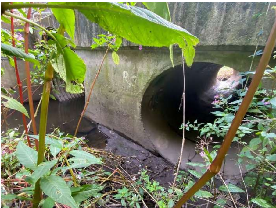
Photograph 6: Greensbridge Lane Structure IMG_2754.JPEG. Photo looking downstream
