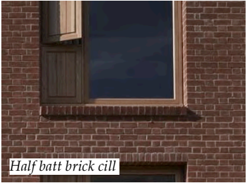
Brick double header course
